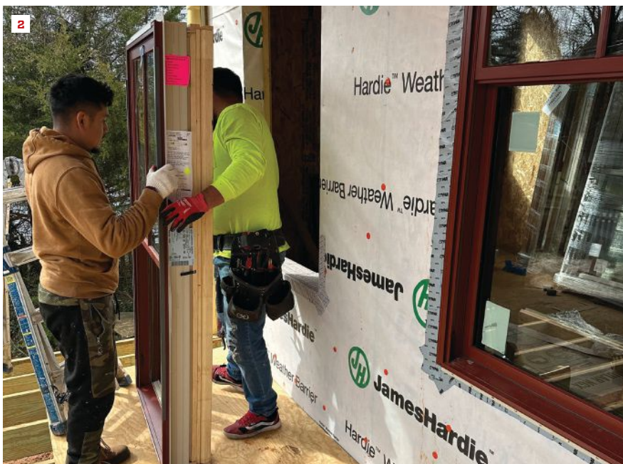
Exterior performance. The crew installs low-E, argon-filled double-pane windows (2) that meet Energy Star Version 3.1 standards for solar heat gain and insulation value in climate zone 4. On the exterior (3), they created a rainscreen with 1x4 pressure-treated wood furring strips installed 16 inches on-center.
