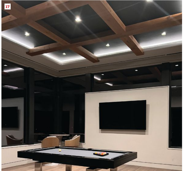
Concealed LED strip lighting was used to accentuate the high, vaulted ceiling planes in the main living room (16). The finished rec room ceiling included coffers (17).
