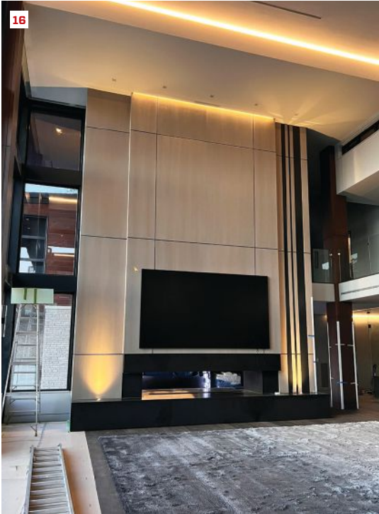
Concealed LED strip lighting was used to accentuate the high, vaulted ceiling planes in the main living room (16). The finished rec room ceiling included coffers (17).
