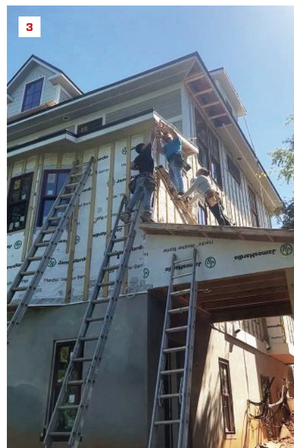
Exterior performance. The crew installs low-E, argon-filled double-pane windows (2) that meet Energy Star Version 3.1 standards for solar heat gain and insulation value in climate zone 4. On the exterior (3), they created a rainscreen with 1x4 pressure-treated wood furring strips installed 16 inches on-center.
