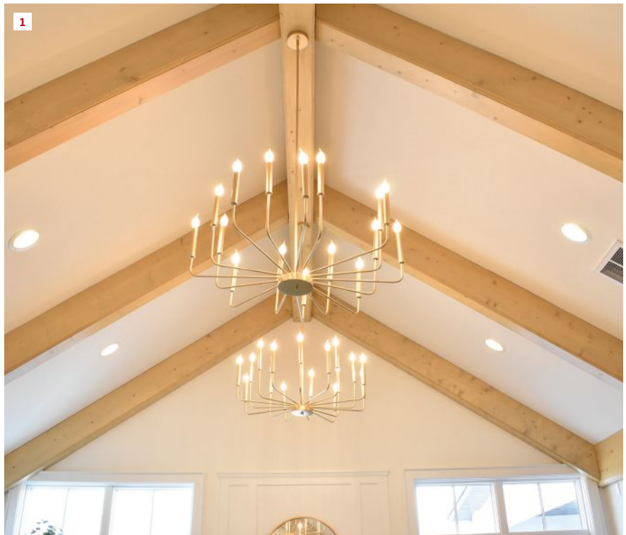
Box beams look like solid timbers but are less challenging to install (1).
