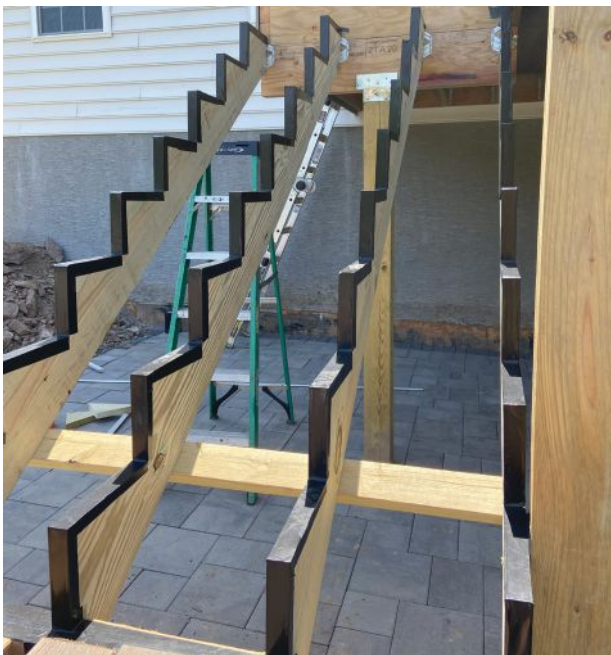
Cutting a stringer creates “end grain” at each stair tread and riser. End grain absorbs water up to 100 times faster than the sides of the lumber do. As such, cut edges of the 2x12 preservative-treated southern pine stringers are flashed.
