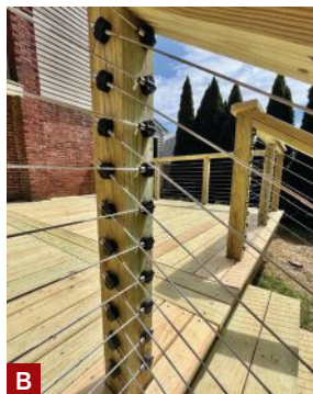
Figure 4. For stair rails, the bracket must be positioned on the post at the same angle as the railing. To accomplish this, the author cut a block at this angle, which he used to sight the angle of the bracket (A). Each angled stair-rail cable passes under the corresponding level cable on the deck (B).
