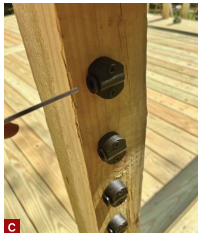
Figure 2. Following the template layout, the brackets are secured to the end posts with two screws per bracket. Next, a “threaded stud spacer” is inserted into each bracket (A). On a worktable, the author assembles a washer and nut on the threaded end of a cable (B). This assembly is fed through the “threaded stud spacer” (C). A flared, unidirectional “pull lock” (D) is then fit onto each cable and pushed into the bracket (E).
