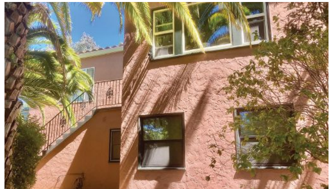
Bonded stucco. Seen above is a 1949 house with three-coat, bonded stucco applied over lumber sheathing.
