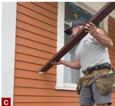
Figure 4. Where upper rails are fastened to the house, the author removed siding and cut back drainage mat, WRB, and board sheathing to install blocking (A). He reinstalled the siding and used a multi-tool to cut pockets for the rails (B), leaving a small gap below for drainage (later, he sealed the tops of the rails to the siding with sealant). The stair railing has similar details, but the nailers aren't beveled, and the rail width is 2 \frac{5}{8} inches for graspability; the ends of the rails and nailers are notched for drainage (D). The author fastened the baluster assemblies to the rails with trim screws driven through oversized pilot holes, which he later capped with Starborn PVC trim plugs (E).
