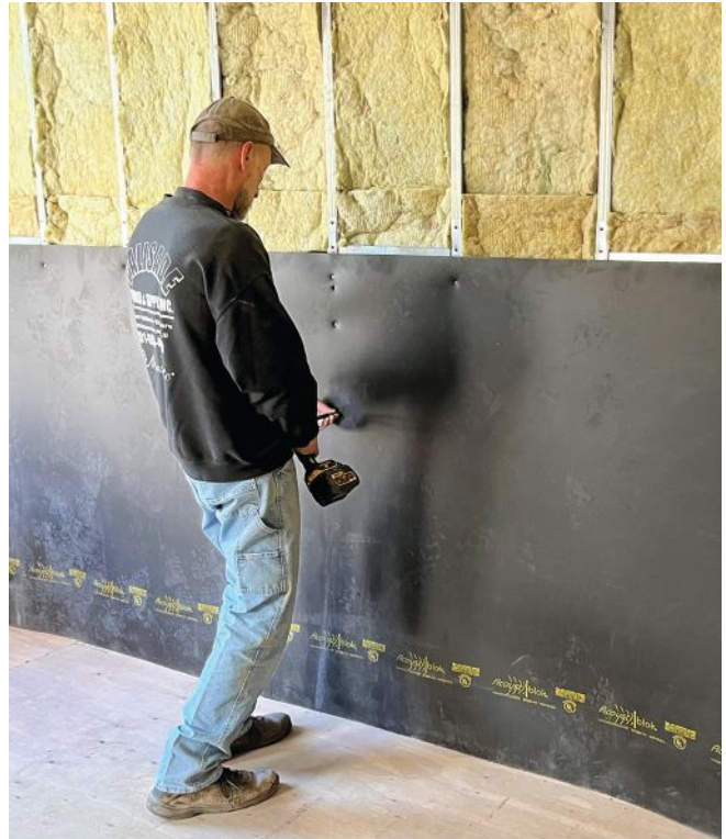
Mass-loaded vinyl is installed over a row-house party wall.
