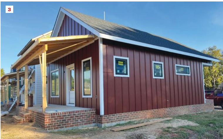
Rob Howard focused on offering high-performance (zero-energy ready) homes at an affordable price. The homes at Duke Street Cottages included a rainscreen on top of SIPs (1, 2) with Hardie fiber-cement trim and siding (3).
