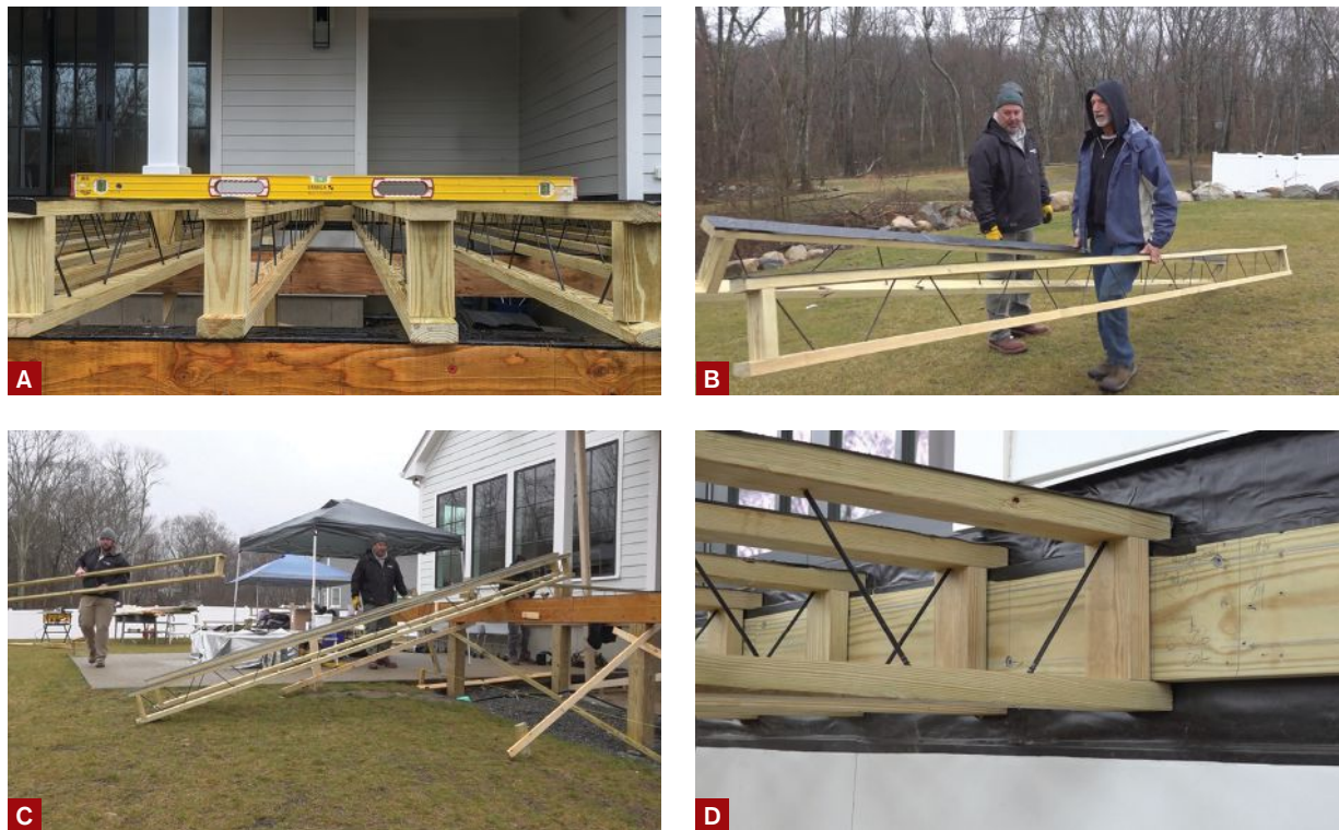
Figure 1. Icon ScrewJoists are fabricated with 2x4 pressure-treated top and bottom chords connected with structural screw webs and are designed to be straight and flat (A). They weigh about half as much as a comparable 2x10 PT joist (B), making them easy to move around a jobsite (C). Instead of requiring a joist hanger, the end of an Icon joist goes over and under the ledger and is fastened to it with pairs of structural screws driven down through the top chord and up through the bottom chord and into the ledger (D). The joists can be ordered with or without waterproofing applied to the top chord.
