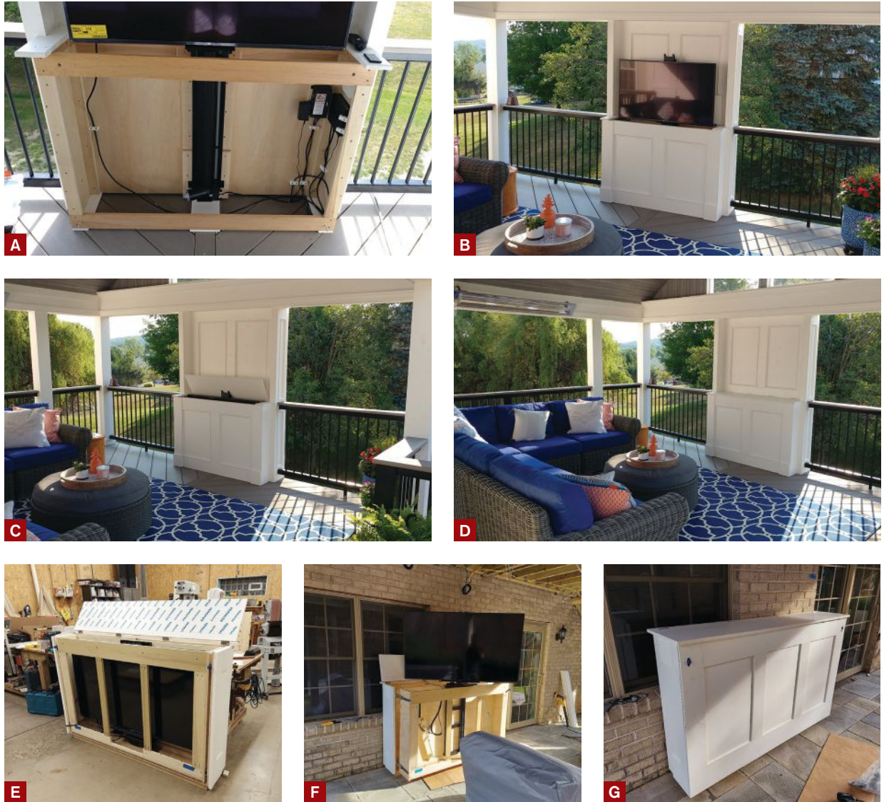
Figure 3. While manufactured outdoor TV cabinets are available, the author prefers to build custom units that he matches to the other finishes in the room and equips with a power pop-up actuator (A). These lifts (a good source is tvliftcabinet.com ) allow the TV to drop down out of sight when not being viewed, with the cabinet lid closing over it automatically (B, C, D). If the TV needs to be able to rotate, the lift can be installed in a cabinet with a pull-out drawer mounted with heavy-duty slides that allow the whole assembly to extend out away from the wall (E, F, G).
