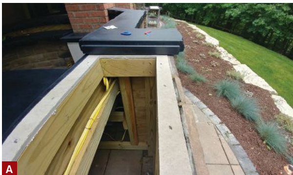
Figure 4. To install a pop-up style of TV lift in an outdoor bar located along the edge of the area that is protected by a roof, the author devised a gutter system to channel water away from the assembly (A). When the TV is retracted and the lid is closed, water is prevented from getting into the enclosure, while the lid lifts up and out of the way when the mechanism raises the TV into viewing position (B).
