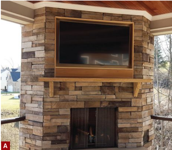
Figure 2. When you're installing an outdoor TV above a fireplace, the author recommends locating it close to a mantel that projects at least 10 inches to help divert heat away from the TV, with the mantel no higher than 5 feet above the floor to preserve viewing angles (A). Sometimes, an insulated flue runs behind the TV, so when building a recessed TV cabinet (B), the author will jog around the flue pipe and add fireproof rigid insulation about 2 inches thick for extra insurance (C).
