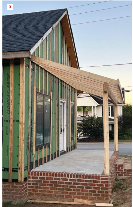
Rob Howard focused on offering high-performance (zero-energy ready) homes at an affordable price. The homes at Duke Street Cottages included a rainscreen on top of SIPs (1, 2) with Hardie fiber-cement trim and siding (3).
