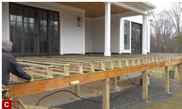
Figure 2. On this project, the Icon joists bear on a two-ply PT LVL dropped perimeter beam supported by PT 6x6 posts, with the top of the beam 1½ inches lower than the bottom of the ledger (A). Once a joist is positioned on the 16-inch-on-center layout, it's fastened to the beam with a pair of structural screws driven down through the bottom chord into the beam (B). Another intermediate dropped three-ply beam provides midspan support and carries point loads from the columns supporting the porch roof (C).
