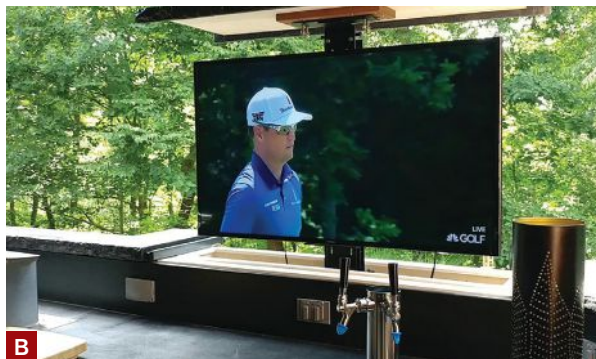
Figure 4. To install a pop-up style of TV lift in an outdoor bar located along the edge of the area that is protected by a roof, the author devised a gutter system to channel water away from the assembly (A). When the TV is retracted and the lid is closed, water is prevented from getting into the enclosure, while the lid lifts up and out of the way when the mechanism raises the TV into viewing position (B).
