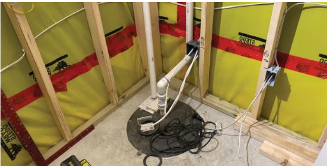
Water management typically includes both protection from groundwater seeping through the foundation (in this case, 15-mil Stego Wrap secured by a termination bar, as shown at top) and interior drains running to a sump pump (above).
