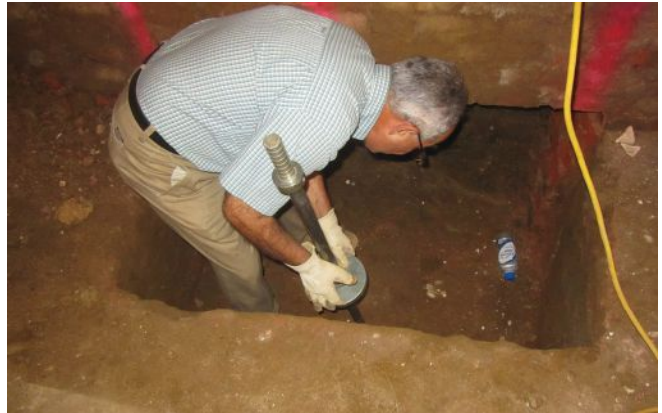
Soil bearing is evaluated at the bottom of one pit by conducting a Dynamic Cone Penetration test.
