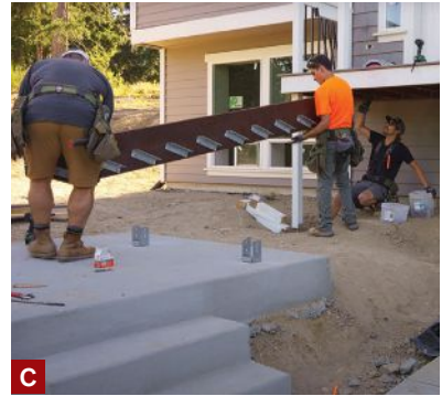
Figure 2. The author clamped the template to each stringer and used it as a guide to drill pilot holes for the mounting brackets (A), which were fastened to the stringers with \frac{3}{8} -inch-diameter lag screws (B). The stringers bear on brackets bolted to the concrete landing (C) and are fastened to the porch with structural screws driven through a doubled rim joist (D). Here, the author is using an impact driver to tighten one of the bottom tread brackets (E).
