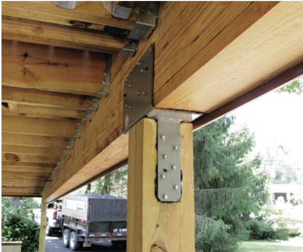
Figure 5. Metal connectors help keep posts and beams aligned at this critical load-path connection but also play an overlooked role in resisting uplift loads (photo, left). The fasteners should be checked per Figure R507.5.1(2) in the 2021 IRC for a covered-deck uplift load (illustration, right).
