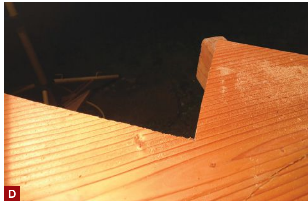
Figure 4. To avoid overcutting the notches, which would weaken the stringer, the author starts the cuts with a circular saw (A, B), and finishes the cuts with either a handsaw or a jigsaw (C). Marking the diagonal increments on the stringer before laying out and cutting the notches ensures that tread and riser dimensions vary by no more than \frac{1}{8} inch (D).
