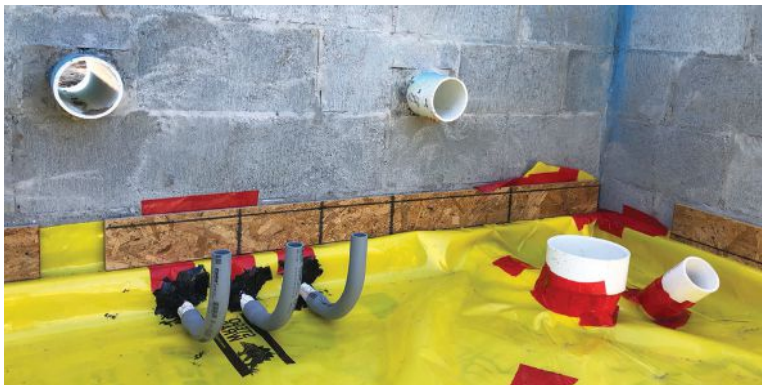
Stego Mastic (black goop around penetrations) and Stego Tape (red) prove effective for sealing Stego Wrap—a thick, polyolefin plastic specifically designed as a subslab vapor retarder.
