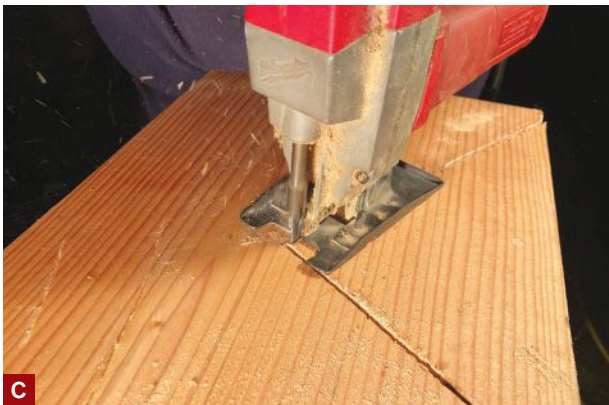
Figure 4. To avoid overcutting the notches, which would weaken the stringer, the author starts the cuts with a circular saw (A, B), and finishes the cuts with either a handsaw or a jigsaw (C). Marking the diagonal increments on the stringer before laying out and cutting the notches ensures that tread and riser dimensions vary by no more than \frac{1}{8} inch (D).
