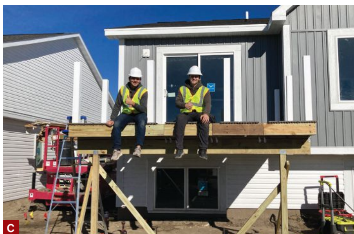
Figure 3. The deck ledger is precut and fitted with double joist hangers off site (A). After the ledger is screwed to the house framing, the crew installs Diamond Pier pin-pile footings, support posts, and the preassembled beam and knee braces needed to support the modules. Workers then use an articulated loader to lift the modules into position (B). The partially completed deck shown here took 15 man hours in the shop and four man hours on site to install (C).
