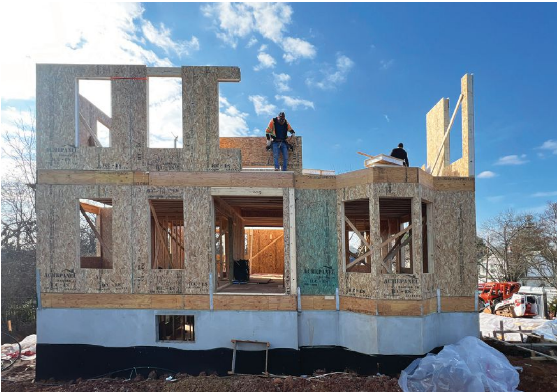
The Queen of Zero framing crew installs SIPs on the second story of this Net Zero Ready Home in Maryland.
