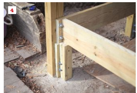
The Rockler portable drill guide has a \frac{1}{2} -inch Jacobs chuck with a \frac{1}{4} -inch hex shank on top that works easily with most drills (1, 2). To accurately drill \frac{5}{8} -inch-diameter holes through a 4x4 post and 2x10 ledger, the author first drilled \frac{1}{4} -inch-diameter pilot holes (3), then switched to a \frac{5}{8} -inch-diameter bit to finish the holes (4).
