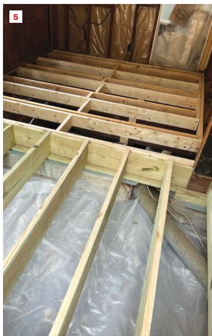
Floors out of level by 1 inch or more typically need to be reframed. Here, a new kitchen floor is being framed in an older home; the original floor was 3 inches out of level (5). The author installs blocking between existing floor trusses under a barrier-free shower to prevent flexing of the subfloor (6, 7). He checks the subfloor for level prior to installing a pre-pitched shower pan (8).
