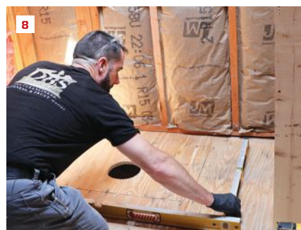
Floors out of level by 1 inch or more typically need to be reframed. Here, a new kitchen floor is being framed in an older home; the original floor was 3 inches out of level (5). The author installs blocking between existing floor trusses under a barrier-free shower to prevent flexing of the subfloor (6, 7). He checks the subfloor for level prior to installing a pre-pitched shower pan (8).
