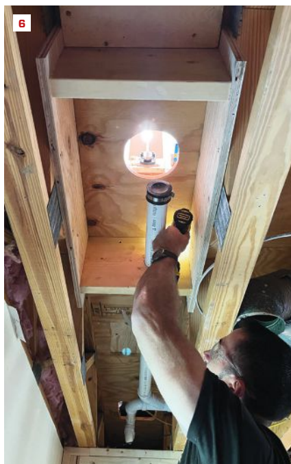
Floors out of level by 1 inch or more typically need to be reframed. Here, a new kitchen floor is being framed in an older home; the original floor was 3 inches out of level (5). The author installs blocking between existing floor trusses under a barrier-free shower to prevent flexing of the subfloor (6, 7). He checks the subfloor for level prior to installing a pre-pitched shower pan (8).
