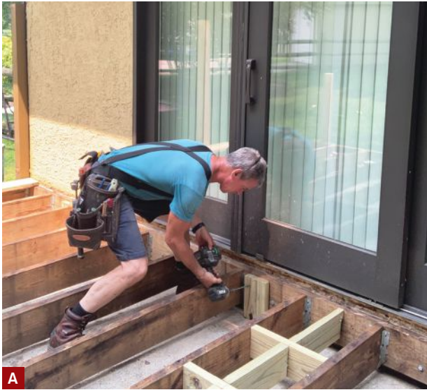
Figure 2. Once the existing framing is exposed, the author reinforces it with structural screws driven through the ledger into the rim joist and blocking as needed (A). To extend the life of the PT framing, the author inserts Post Proservative rods containing a fungicide and wood preservative into holes bored into the wood (B).
