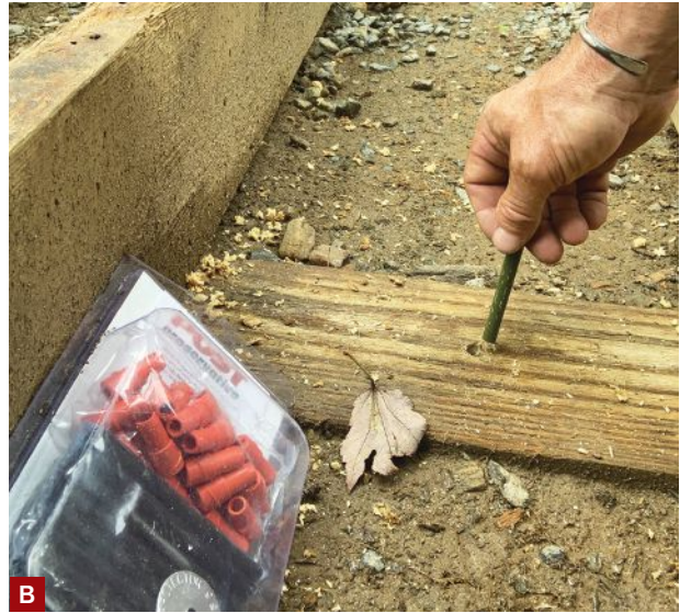
Figure 2. Once the existing framing is exposed, the author reinforces it with structural screws driven through the ledger into the rim joist and blocking as needed (A). To extend the life of the PT framing, the author inserts Post Proservative rods containing a fungicide and wood preservative into holes bored into the wood (B).
