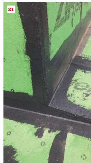
Roof-to-wall seal. For an effective air seal around rafters, the crew cuts the sheathing to fit around the rafters, and the joint between the sheathing and the rafter tails is carefully filled with fluid-applied (19). Similarly, the spaces between outlookers on the rake ends (20) and any roof transitions (21) are filled with a bed of fluid-applied sealant.
