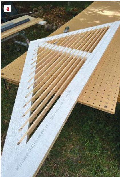
After routing the mortises, the author ripped louvers so they are flush to the back (4), providing a flat surface to which bug screen can be attached. A steeper mortise angle and wider louvers would provide more weather protection, but in this case the finished vent (5) would be installed under a wide rake overhang, which offered enough protection from the elements.
