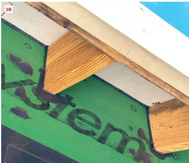
Roof-to-wall seal. For an effective air seal around rafters, the crew cuts the sheathing to fit around the rafters, and the joint between the sheathing and the rafter tails is carefully filled with fluid-applied (19). Similarly, the spaces between outlookers on the rake ends (20) and any roof transitions (21) are filled with a bed of fluid-applied sealant.
