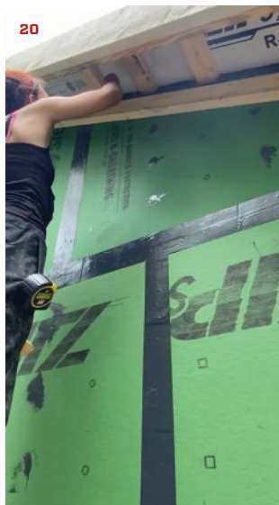
Roof-to-wall seal. For an effective air seal around rafters, the crew cuts the sheathing to fit around the rafters, and the joint between the sheathing and the rafter tails is carefully filled with fluid-applied (19). Similarly, the spaces between outlookers on the rake ends (20) and any roof transitions (21) are filled with a bed of fluid-applied sealant.
