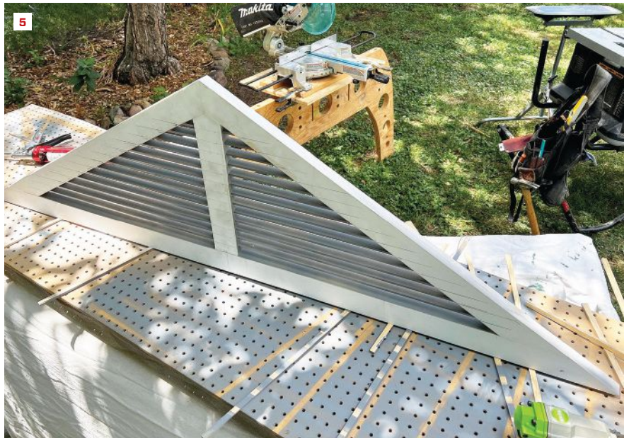
After routing the mortises, the author ripped louvers so they are flush to the back (4), providing a flat surface to which bug screen can be attached. A steeper mortise angle and wider louvers would provide more weather protection, but in this case the finished vent (5) would be installed under a wide rake overhang, which offered enough protection from the elements.
