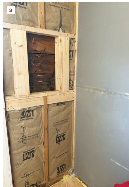
On a bathroom remodel, the author began with demolishing the existing shower (1). To correct a sagging floor, he had to reframe it (2). An out-of-plumb wall also needed to be reframed (3).
