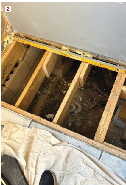
On a bathroom remodel, the author began with demolishing the existing shower (1). To correct a sagging floor, he had to reframe it (2). An out-of-plumb wall also needed to be reframed (3).
