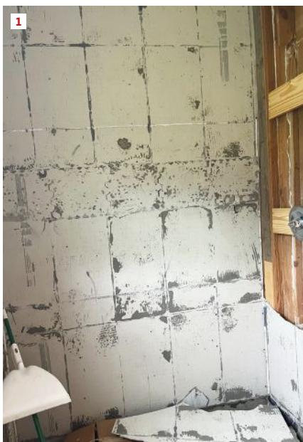
On a bathroom remodel, the author began with demolishing the existing shower (1). To correct a sagging floor, he had to reframe it (2). An out-of-plumb wall also needed to be reframed (3).
