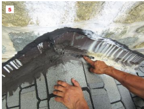
In the attic above the damage, IR imaging (inset) shows wet chimney block (3). An M & J trade partner inspects the chimney's base; roofing cement covers its shingle-to-flashing juncture (4, 5).
