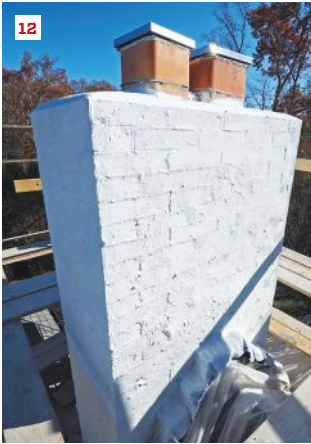
A waterproof cement-based coating (MasterSeal 581) is applied up and over the block chimney core (12). The stepped, 16-ounce copper through-flashings are fabricated and soldered on site (13). The large pieces are tacked in place with masonry anchors, and the edges sealed with polyurethane caulk (14).
