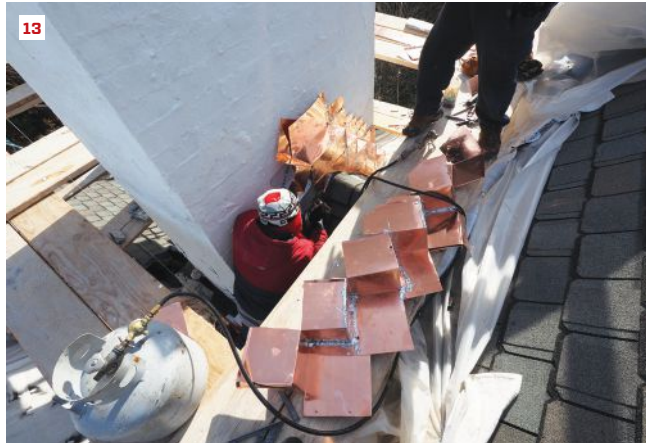
A waterproof cement-based coating (MasterSeal 581) is applied up and over the block chimney core (12). The stepped, 16-ounce copper through-flashings are fabricated and soldered on site (13). The large pieces are tacked in place with masonry anchors, and the edges sealed with polyurethane caulk (14).
