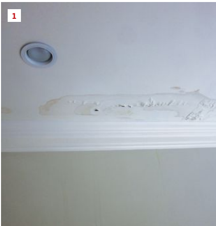
Water damage is evident on a ceiling above a second-floor fireplace (1). Infrared imaging confirms that the area is wet after rainstorms (2).
