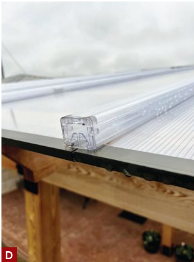
Figure 2. Angle brackets are used to fasten the rafters to the beams, along with structural screws driven down through the tops of the rafters (A). The roof panels are supported by 2x4 purlins and are fastened to them with special metal clips (B). Friction-fit connector caps are tapped into place with a mallet to cover the raised seams between panels and prevent leakage (C), then plugged with matching end caps (D). The ends of the hollow panels are covered with a special vent tape followed by a flute cover, allowing for ventilation while blocking access to insects (E). The outside edge of the last panel is cut to fit, then covered with a metal U-edge profile that is screwed to the purlins (F).
