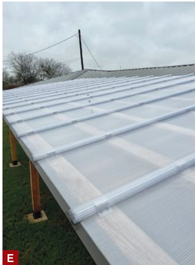
Figure 2. Angle brackets are used to fasten the rafters to the beams, along with structural screws driven down through the tops of the rafters (A). The roof panels are supported by 2x4 purlins and are fastened to them with special metal clips (B). Friction-fit connector caps are tapped into place with a mallet to cover the raised seams between panels and prevent leakage (C), then plugged with matching end caps (D). The ends of the hollow panels are covered with a special vent tape followed by a flute cover, allowing for ventilation while blocking access to insects (E). The outside edge of the last panel is cut to fit, then covered with a metal U-edge profile that is screwed to the purlins (F).
