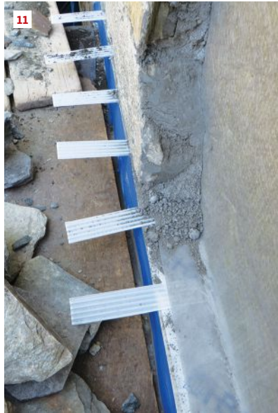
After the self-adhering membrane backup flashing was installed, the metal through-wall flashing was installed over it (seen here on an adjacent roof) (9). The exposed face of coated copper flashing was protected with blue tape, then the water management layers were installed on the wall (10). Self-spaced corrugated plastic weeps provided enhanced draining (11, 12).
