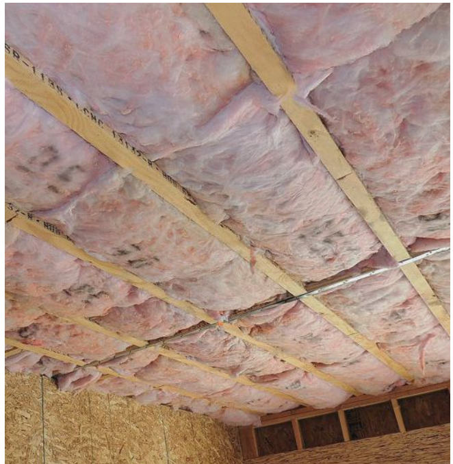
Use full-width batts for insulating between I joists.
