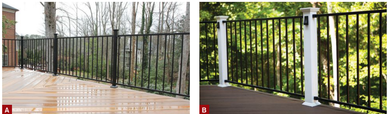
Figure 4. Another way the author streamlines the design and estimating process is by offering a limited number of railing options. Here, the same black aluminum railing panel is shown with two different post styles (A, B).
