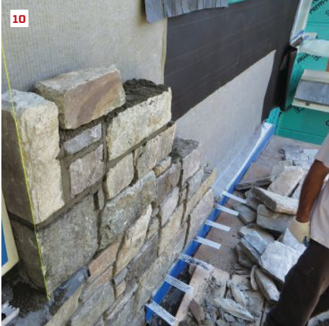
After the self-adhering membrane backup flashing was installed, the metal through-wall flashing was installed over it (seen here on an adjacent roof) (9). The exposed face of coated copper flashing was protected with blue tape, then the water management layers were installed on the wall (10). Self-spaced corrugated plastic weeps provided enhanced draining (11, 12).
