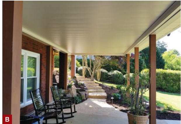
Figure 5. Under-deck ceiling options can also be standardized. The author's premium waterproofing package includes column wraps, wood ceiling, and crown molding (A). The basic package uses an aluminum under-deck system and costs considerably less.
