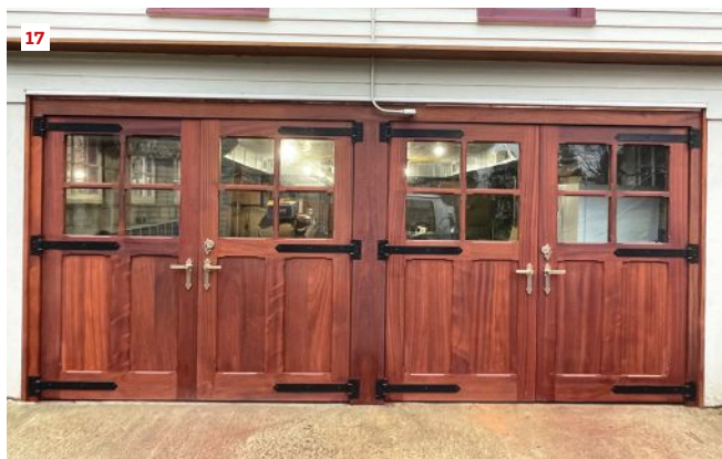
The hinge leaves were attached to the rebuilt framed openings with galvanized lag bolts (15). From the interior, the hinge hardware included metal back plates, which were through-bolted to hinge straps (16). The panes of 1/4-inch tempered glass were set in a small bead of silicone sealant (17). The finish door hardware was made by Rocky Mountain Hardware (18).
