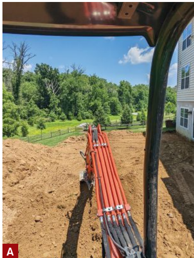
Figure 1. The author uses a bulldozer, a skid steer, and a small tractor for general site work, as well as a Kubota KX040 compact excavator (A). After the site was leveled, the excavator was used to dig for footings for the deck and storage-room walls, and for the sitting walls at the corners of the patio (B).
