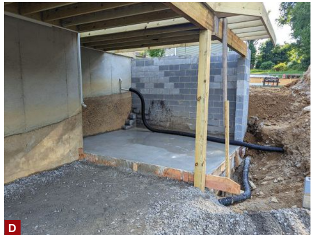
Figure 2. Shown here is the formwork for the footings (A) that support the engineered block retaining wall (B) built to partially enclose a dry storage area underneath the deck. After the retaining wall was built, the author's Kubota SSV65 skid loader was used to lift the heavy deck beam into position (C). The storage room has a concrete slab floor (D).
