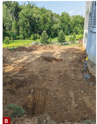
Figure 1. The author uses a bulldozer, a skid steer, and a small tractor for general site work, as well as a Kubota KX040 compact excavator (A). After the site was leveled, the excavator was used to dig for footings for the deck and storage-room walls, and for the sitting walls at the corners of the patio (B).
