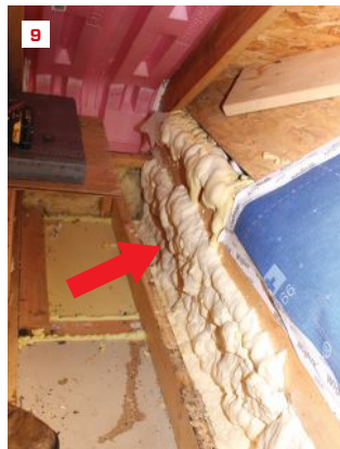
Exposed batts were covered with Majvest membrane where the garage wing and main house intersect (8). The exposed, "cold" end of the LVL is foamed with froth pack to stop condensation from forming and leaking into the house (9).
