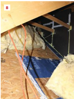
Exposed batts were covered with Majvest membrane where the garage wing and main house intersect (8). The exposed, "cold" end of the LVL is foamed with froth pack to stop condensation from forming and leaking into the house (9).
