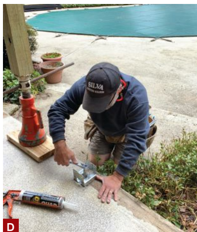
Figure 3. At each post location, the author traced the post's footprint onto the slab (A), then recut the post to fit the metal post base and traced again around the post base (B). Next, he drilled a 1/2-inch-diameter hole for the 1/2-inch-diameter wedge anchor that he used to fasten the metal base to the slab (C). As he tightened down the nut (D), he checked the base for level and used metal washers to shim between the slab and the base as needed; a dab of adhesive sealant on the washers ensured that they'd stay put under the weight of the post during assembly (E). Then he inserted the post and fastened it to the metal hardware with structural screws (F).
