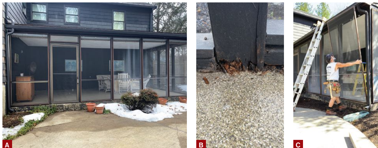
Figure 1. The roof of the existing screen porch was structurally sound (A), but the fir posts and sill plates were rotting where they were in direct contact with the porch's concrete slab floor and needed to be replaced (B). The aluminum screening in the aluminum-framed panels also needed replacement (C).
