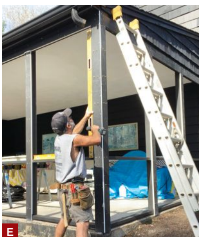
Figure 5. After cutting the PVC post claddings to size, the author used a router to relieve the backs to fit over the metal post bases (A). He also routed \frac{1}{4} -inch square grooves down their backs to create a drainage channel (B). The long fascia was joined together from several pieces with half-lap joints, a configuration that allows the PVC to move with changes in temperature without opening up the joints (C). The author prefabricated the corner from two pieces of PVC joined together with PVC glue and Cortex screws (D). Cortex screws were used to fasten the PVC trim to the framing (E). Scribing the bottom rails to the irregular concrete slab ensured a tight fit (F).
