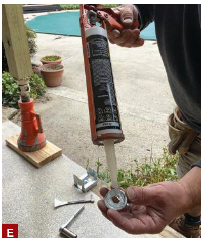
Figure 3. At each post location, the author traced the post's footprint onto the slab (A), then recut the post to fit the metal post base and traced again around the post base (B). Next, he drilled a 1/2-inch-diameter hole for the 1/2-inch-diameter wedge anchor that he used to fasten the metal base to the slab (C). As he tightened down the nut (D), he checked the base for level and used metal washers to shim between the slab and the base as needed; a dab of adhesive sealant on the washers ensured that they'd stay put under the weight of the post during assembly (E). Then he inserted the post and fastened it to the metal hardware with structural screws (F).
