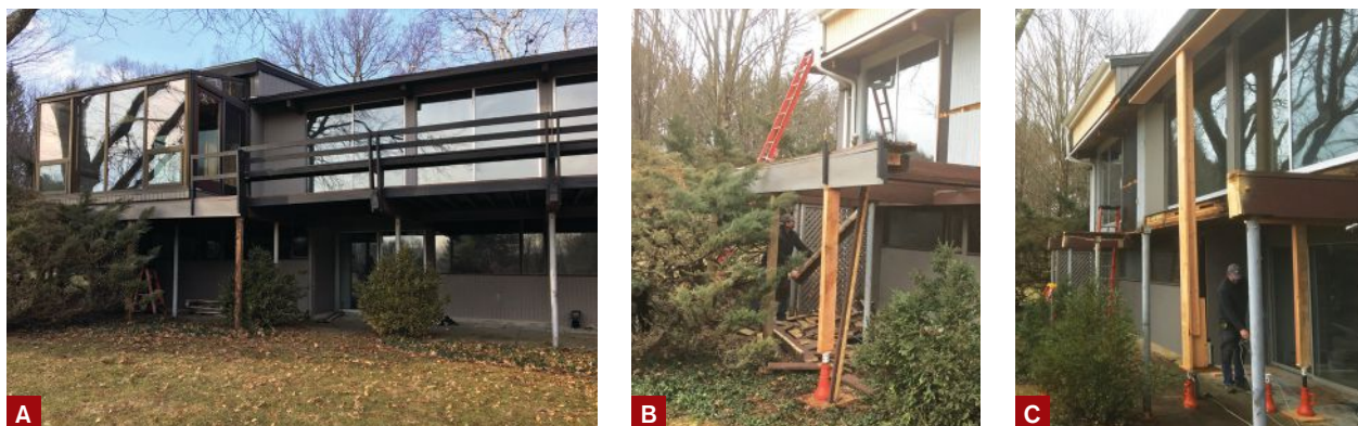
Figure 3. An ill-suited sunroom, not in keeping with the home's style, that had been built on the deck (A) was removed (B), as well as the bump-up transition on the main roof. During the project, workers posted up the cantilevered floor and roof as necessary (C).
