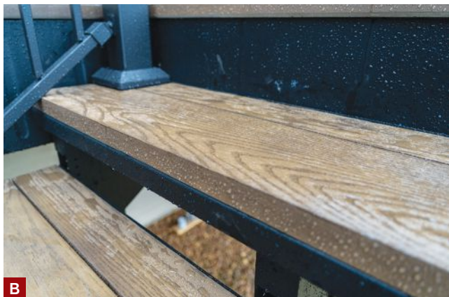
The enhanced grain of Millboard decking offers good slip resistance (A). While bullnose boards are available for stair treads, the author typically uses standard square-edged boards with Fortress's steel stair framing (B).
