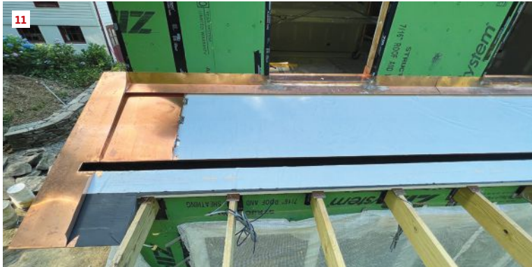
Copper windowsill pan flashing is soldered to continuous apron flashing at the roof-to-wall junction. Standing-seam panels are locked into drip-edge flashing along the upslope edge of the built-in (11).
