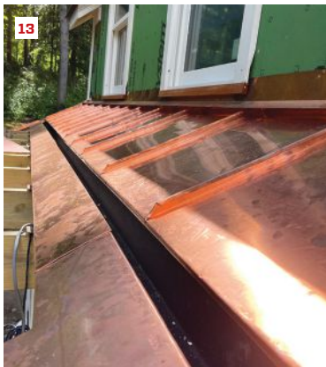
The completed standing-seam copper roof (13). Copper downspouts will be installed later (14), as well as a copper gutter and downspout on the shed-dormer roof above.
