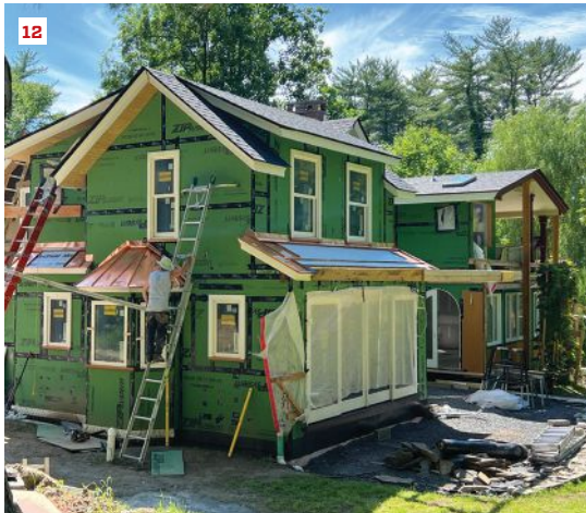
Copper windowsill pan flashing is soldered to continuous apron flashing at the roof-to-wall junction. Standing-seam panels are locked into drip-edge flashing along the upslope edge of the built-in (11).
