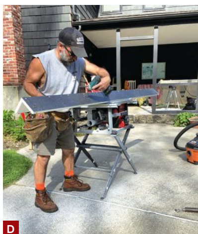
Figure 5. After cutting the PVC post claddings to size, the author used a router to relieve the backs to fit over the metal post bases (A). He also routed \frac{1}{4} -inch square grooves down their backs to create a drainage channel (B). The long fascia was joined together from several pieces with half-lap joints, a configuration that allows the PVC to move with changes in temperature without opening up the joints (C). The author prefabricated the corner from two pieces of PVC joined together with PVC glue and Cortex screws (D). Cortex screws were used to fasten the PVC trim to the framing (E). Scribing the bottom rails to the irregular concrete slab ensured a tight fit (F).
