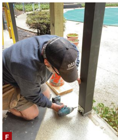
Figure 3. At each post location, the author traced the post's footprint onto the slab (A), then recut the post to fit the metal post base and traced again around the post base (B). Next, he drilled a 1/2-inch-diameter hole for the 1/2-inch-diameter wedge anchor that he used to fasten the metal base to the slab (C). As he tightened down the nut (D), he checked the base for level and used metal washers to shim between the slab and the base as needed; a dab of adhesive sealant on the washers ensured that they'd stay put under the weight of the post during assembly (E). Then he inserted the post and fastened it to the metal hardware with structural screws (F).
