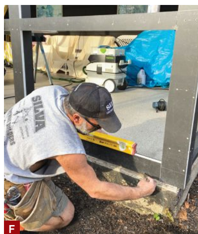
Figure 5. After cutting the PVC post claddings to size, the author used a router to relieve the backs to fit over the metal post bases (A). He also routed \frac{1}{4} -inch square grooves down their backs to create a drainage channel (B). The long fascia was joined together from several pieces with half-lap joints, a configuration that allows the PVC to move with changes in temperature without opening up the joints (C). The author prefabricated the corner from two pieces of PVC joined together with PVC glue and Cortex screws (D). Cortex screws were used to fasten the PVC trim to the framing (E). Scribing the bottom rails to the irregular concrete slab ensured a tight fit (F).
