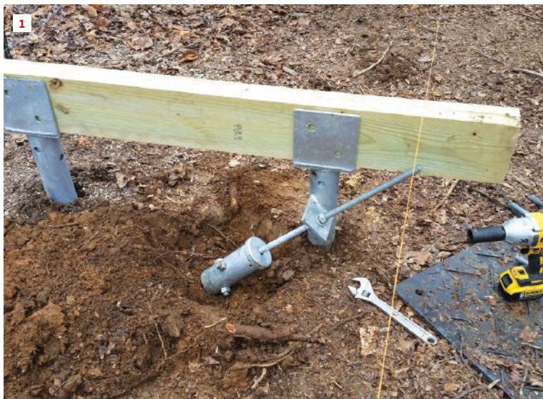
In this photo showing the framing for a commercial elevated walkway, one of the vertical helical piles is reinforced by a batter pile installed at an angle to limit lateral movement caused by foot traffic on the walkway. A threaded rod bolted to a plate that's welded to the vertical pile connects the two piles (1).
