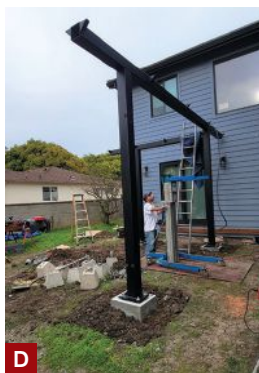
Figure 3. The homeowner (at center in photo) helps wrangle the first beam into place with the help of a Genie lift (A). The beam is bolted to the posts (B), then the second, longer beam is hoisted into place and secured (C, D).
