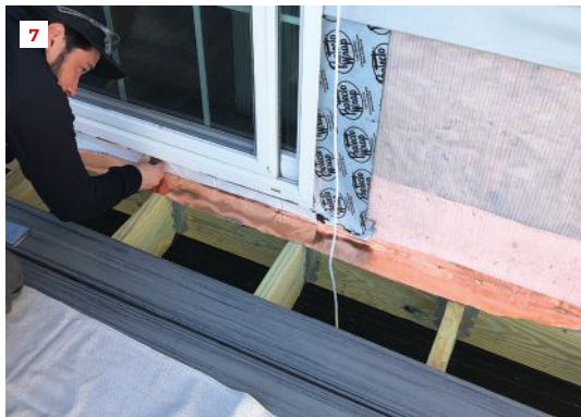
After re-insulating (5) and resheathing the walls, workers installed a peel-and-stick membrane in the ledger area (6), running the membrane 6 inches above the new deck elevation and behind the WRB.
