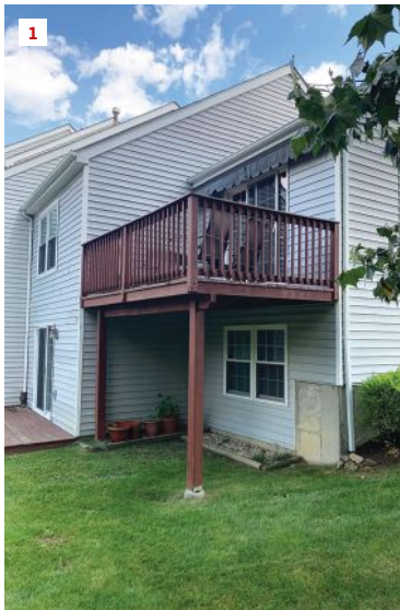
While the existing deck displayed no outward signs of instability (1) , the ledgers had not been properly flashed and the underlying OSB sheathing was revealed to be water damaged upon removal (2) .
