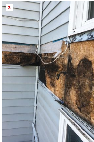
While the existing deck displayed no outward signs of instability (1) , the ledgers had not been properly flashed and the underlying OSB sheathing was revealed to be water damaged upon removal (2) .
