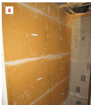
Enclosures for steam showers need to be fully water- and vapor-proofed on all sides. Surfaces, including ceilings, are typically tiled, and large areas of glass (door, side, and top wall panels) are used to let in outside light and increase ambiance (1). Here, insulated Kerdi Board is installed on an exterior wall, keeping the shower side warmer and providing a more comfortable bathing experience (2). A soffit hides the sloped ceiling on an in-progress installation (3). Curved ceilings are nice design features that allow for steeper sloping (4, 5).
