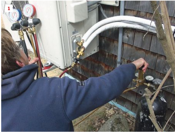
Failure to charge an air-source heat pump to 100% has a severe impact on not only the unit's rated capacity but also on power draw, as shown in the graph at right. Pressure testing (1) ensures a leak-free refrigerant line.
