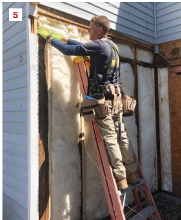
After re-insulating (5) and resheathing the walls, workers installed a peel-and-stick membrane in the ledger area (6), running the membrane 6 inches above the new deck elevation and behind the WRB.
