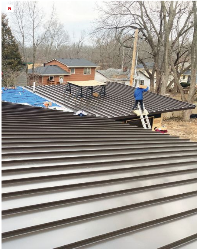
The author uses commodity OSB to sheathe the overroof. Once covered with a peel-and-stick synthetic underlayment and metal roofing, the assembly is sound (5). The truss-frame underroof was insulated with R-38 stone wool batts (6), resulting in a nominal R-58 for the lid of the home. Combined with the rigorous air barrier, the assembly avoids any condensation risk.
