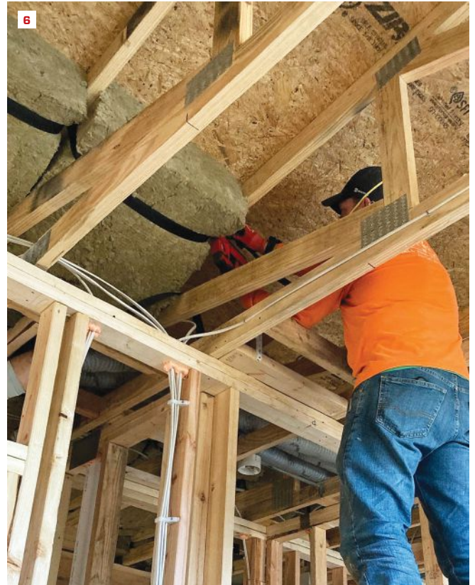
The author uses commodity OSB to sheathe the overroof. Once covered with a peel-and-stick synthetic underlayment and metal roofing, the assembly is sound (5). The truss-frame underroof was insulated with R-38 stone wool batts (6), resulting in a nominal R-58 for the lid of the home. Combined with the rigorous air barrier, the assembly avoids any condensation risk.
