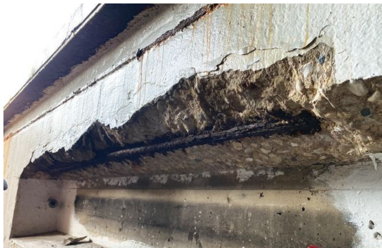
Rebar encased in concrete can still corrode, but the process is typically very slow. The surface corrosion shown here doesn't affect the steel's structural integrity and can be cleaned off prior to repriming and concrete repair work.
