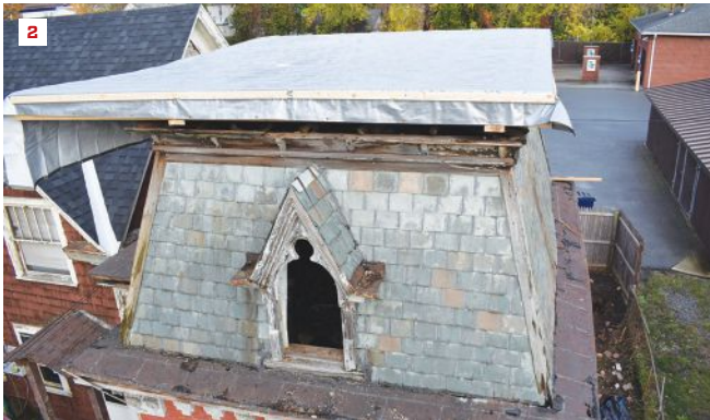
The existing roof was funneling water into the building (1), so the author covered it with a temporary roof framed with 2x10s, sheathed, and topped with a heavy tarp (2). Temporary 2-by bracing around the perimeter helped the roof support snow loads over the winter months (3).
