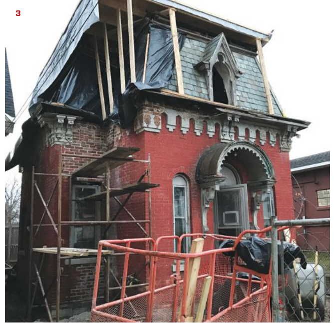
The existing roof was funneling water into the building (1), so the author covered it with a temporary roof framed with 2x10s, sheathed, and topped with a heavy tarp (2). Temporary 2-by bracing around the perimeter helped the roof support snow loads over the winter months (3).
