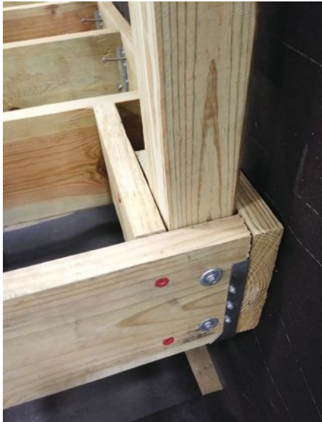
Figure 8. Where a corner post at the ledger can't be screwed through the sheathing into wall framing, the author reinforces the connection of the end joist to the deck framing with blocking as shown, then fastens the post to the end joist and 4x4 blocking with a pair of ThruLok screws.
