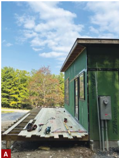
Figure 2. To ensure that the visible fastener heads would be aligned, the author snapped chalk lines on top of the pressure treated decking to mark the joist layout (A). The width of the deck was planned so that there would be no ripped deck boards; decking was installed from the ledger out toward the rim joist. All the end cuts on the decking were eased with a router (B).
