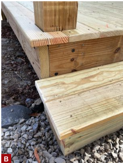
Figure 2. To ensure that the visible fastener heads would be aligned, the author snapped chalk lines on top of the pressure treated decking to mark the joist layout (A). The width of the deck was planned so that there would be no ripped deck boards; decking was installed from the ledger out toward the rim joist. All the end cuts on the decking were eased with a router (B).
