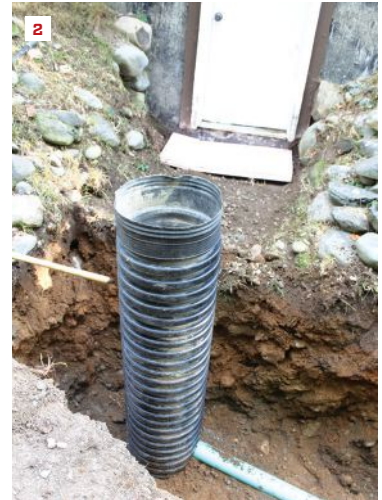
Excavation begins at the basement walkout (1). A length of 15-inch-diameter HDPE culvert installed vertically acts as a catch basin; 4-inch SDR-35 pipe inserted into the culvert's base serves as an outlet (2).
