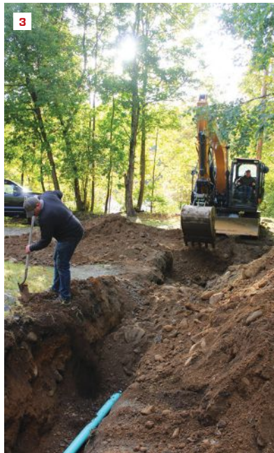
The 75-foot run to daylight is excavated in two sections: first, the walkout end, then the daylight end (3). A crew member joins lengths of SDR-35 with PVC cement (4). The daylight-side piping is complete and ready for backfilling (5).
