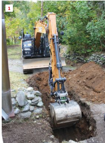
Excavation begins at the basement walkout (1). A length of 15-inch-diameter HDPE culvert installed vertically acts as a catch basin; 4-inch SDR-35 pipe inserted into the culvert's base serves as an outlet (2).
