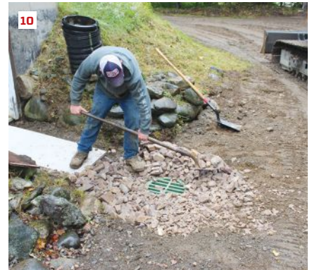
After the HDPE pipe is trimmed closer to grade, the basin's heavy-duty HDPE grate is dryfit to prevent dirt and stone from entering the basin (6) during backfilling (7). The pipe is cut to its finished height, a few inches below slab height (8), and clay soils are used to create a slope away from the house toward the basin (9). Ditch stone is applied around the finished basin (10).
