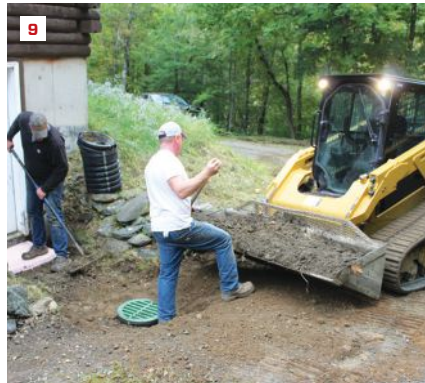
After the HDPE pipe is trimmed closer to grade, the basin's heavy-duty HDPE grate is dryfit to prevent dirt and stone from entering the basin (6) during backfilling (7). The pipe is cut to its finished height, a few inches below slab height (8), and clay soils are used to create a slope away from the house toward the basin (9). Ditch stone is applied around the finished basin (10).
