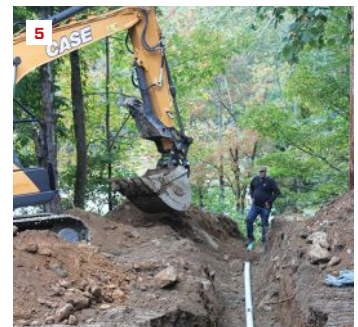
The 75-foot run to daylight is excavated in two sections: first, the walkout end, then the daylight end (3). A crew member joins lengths of SDR-35 with PVC cement (4). The daylight-side piping is complete and ready for backfilling (5).
