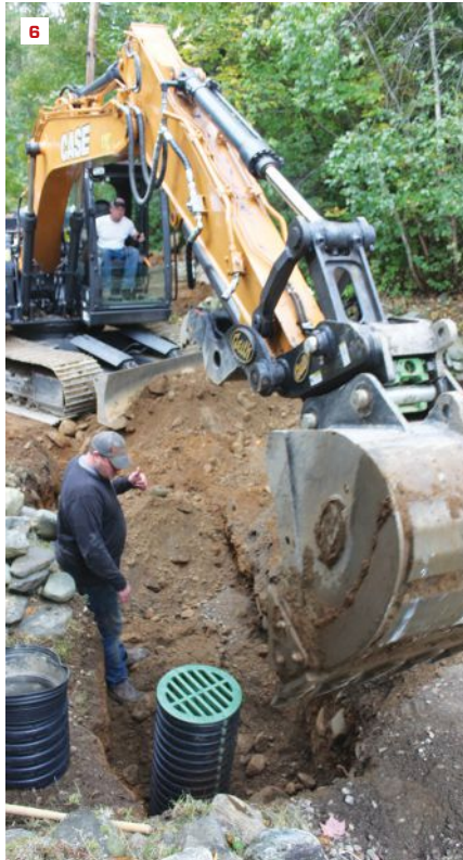
After the HDPE pipe is trimmed closer to grade, the basin's heavy-duty HDPE grate is dryfit to prevent dirt and stone from entering the basin (6) during backfilling (7). The pipe is cut to its finished height, a few inches below slab height (8), and clay soils are used to create a slope away from the house toward the basin (9). Ditch stone is applied around the finished basin (10).
