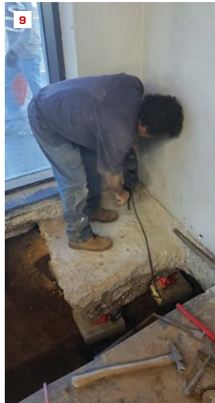
Moment frame. A 1/8-inch-thick steel template (10) made to correspond to the steel bottom plate (8) is used to lay out the drilled anchor bolt locations (9). The template holds the all-thread bolts in alignment (10) during the concrete pour (11).
