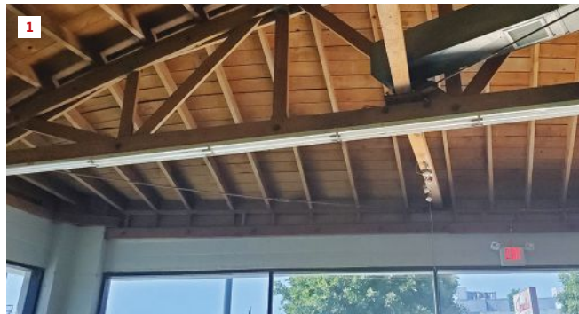
The 2-by rafters transition from a bowstring truss to a ledger above a wall-to-wall storefront entry (1).
