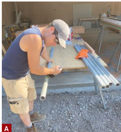
Figure 2. Before sliding the 2-inch hot-dipped galvanized piping into the cedar posts, workers brushed Gorilla glue onto the pipe ends (A). With the post assemblies standing up against a wall, gravity did the work of settling the wood onto the steel (B).
