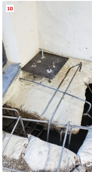
Moment frame. A 1/8-inch-thick steel template (10) made to correspond to the steel bottom plate (8) is used to lay out the drilled anchor bolt locations (9). The template holds the all-thread bolts in alignment (10) during the concrete pour (11).
