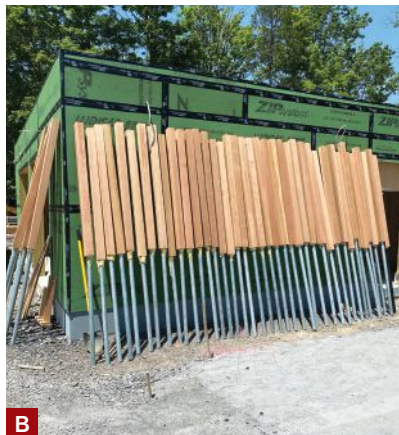
Figure 2. Before sliding the 2-inch hot-dipped galvanized piping into the cedar posts, workers brushed Gorilla glue onto the pipe ends (A). With the post assemblies standing up against a wall, gravity did the work of settling the wood onto the steel (B).
