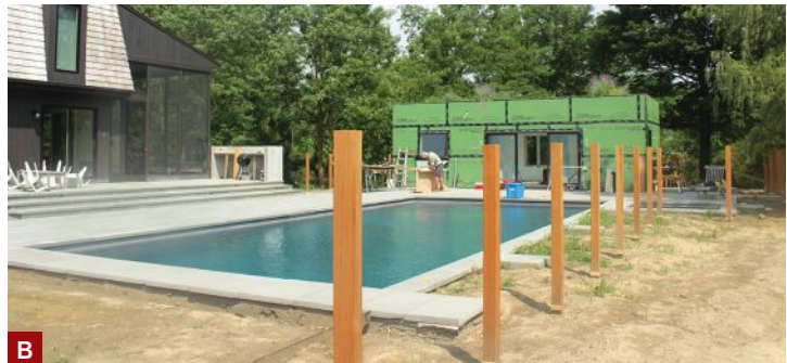
Figure 3. A Toro Dingo with an auger powerhead (A, at left) bored 8-inch holes for the post footings. After installation, the posts were trimmed level with a portable 6-inch battery-powered band saw (B).
