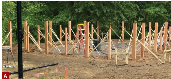
Figure 3. A Toro Dingo with an auger powerhead (A, at left) bored 8-inch holes for the post footings. After installation, the posts were trimmed level with a portable 6-inch battery-powered band saw (B).
