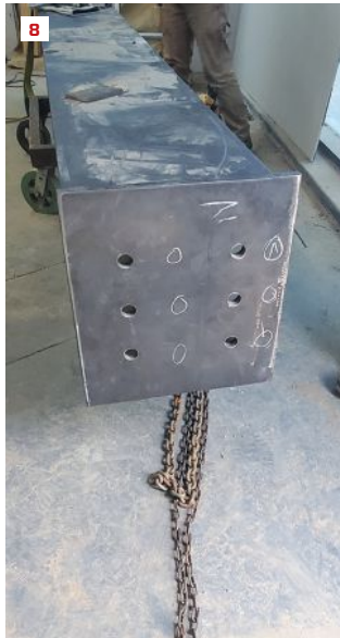
Moment frame. A 1/8-inch-thick steel template (10) made to correspond to the steel bottom plate (8) is used to lay out the drilled anchor bolt locations (9). The template holds the all-thread bolts in alignment (10) during the concrete pour (11).
