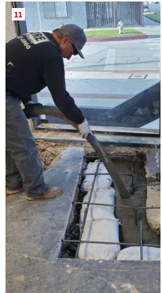
Moment frame. A 1/8-inch-thick steel template (10) made to correspond to the steel bottom plate (8) is used to lay out the drilled anchor bolt locations (9). The template holds the all-thread bolts in alignment (10) during the concrete pour (11).
