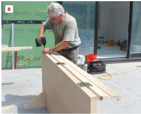
The author installs the door hinges on the routed hinge-side door frame (7) and fastens the frame to the door (8). Working inside, he and Brady position the door and frame assembly in place hands-free using a pair of Door Studs (9).
