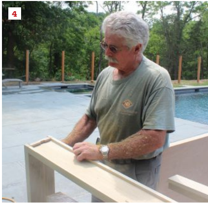
The head piece laps over the jambs (4). Ed Brady uses a multi-tool to notch out material on the head piece to create 1/2-inch returns, which will allow it to slip around the wall (5). After setting the door upright on its side in custom-built door stands, the author routs the hinge locations using a Porter-Cable hinge butt template kit (6).
