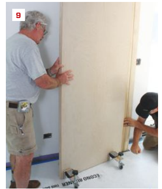
The author installs the door hinges on the routed hinge-side door frame (7) and fastens the frame to the door (8). Working inside, he and Brady position the door and frame assembly in place hands-free using a pair of Door Studs (9).
