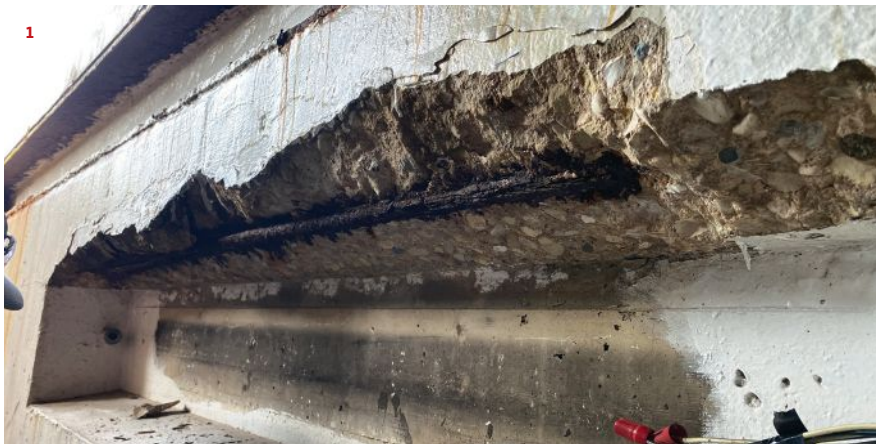
The outside corner of this lighting niche in a mechanic's well had become unstable (1). Repair work began by chipping out the corner (2) and removing enough material that new mortar could fully encase the existing rebar (3). In addition, the crew used a grinder to remove the old paint in the area where the new concrete meets the existing surface (4). This way, when the new concrete work is painted, you won't see where the new concrete meets the old.
