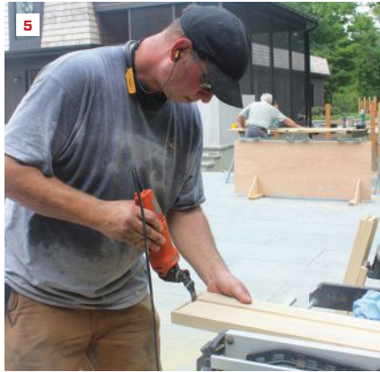
The head piece laps over the jambs (4). Ed Brady uses a multi-tool to notch out material on the head piece to create 1/2-inch returns, which will allow it to slip around the wall (5). After setting the door upright on its side in custom-built door stands, the author routs the hinge locations using a Porter-Cable hinge butt template kit (6).
