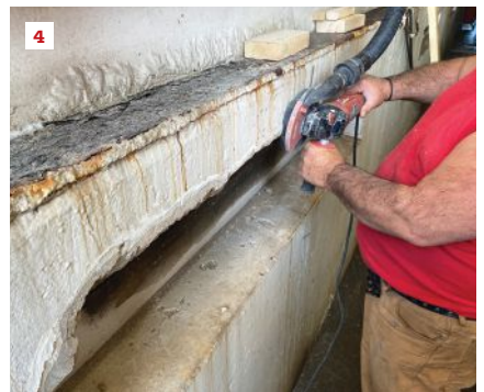
The outside corner of this lighting niche in a mechanic's well had become unstable (1). Repair work began by chipping out the corner (2) and removing enough material that new mortar could fully encase the existing rebar (3). In addition, the crew used a grinder to remove the old paint in the area where the new concrete meets the existing surface (4). This way, when the new concrete work is painted, you won't see where the new concrete meets the old.
