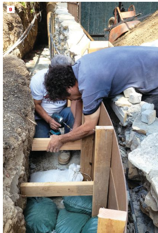
The collapsed portion of the wall was rebuilt using salvaged and new stone (8). Sheets of 1/4-inch-thick Masonite, 2x4 horizontal blocks, and sandbags were used as wall forms on the shorter curved wall sections (9).
