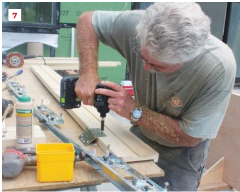
The author installs the door hinges on the routed hinge-side door frame (7) and fastens the frame to the door (8). Working inside, he and Brady position the door and frame assembly in place hands-free using a pair of Door Studs (9).
