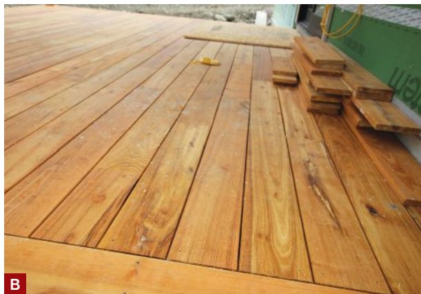
Figure 2. Known more as a “fence post” wood because of its strength and rot-resistance, black locust can also be milled into decking (A). It features a prominent grain and golden color (B), which will eventually develop a silvery gray patina.
