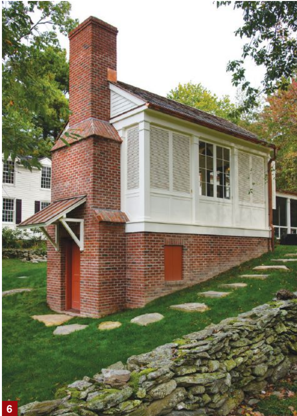
The exterior brickwork for the wood-fired pizza oven is a major feature on the building's north-facing façade. The wine cellar has an inswing door covered with a Craftsman-style copper roof, allowing sheltered access to wine during snowy Taconic mountain weather (6).
