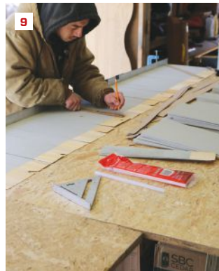
The template has a wave pattern with a 2\frac{9}{16} -inch wave height (6) and a 2\frac{1}{2} -inch frequency (7); vertical lines represent the 2\frac{11}{16} -inch wave offsets between courses. With the base course butted to a straightedge (8), a worker marks the shingles for two rows of drywall shims (9) and glues them on (10). Applying pressure with a roller improves adhesion (11).
