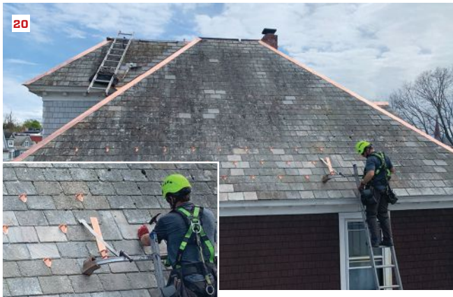
Copper snow guards (inset photo) applied on the north side of the roof will help keep ice from falling into the neighbor's driveway below (20).
