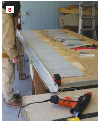
The template has a wave pattern with a 2\frac{9}{16} -inch wave height (6) and a 2\frac{1}{2} -inch frequency (7); vertical lines represent the 2\frac{11}{16} -inch wave offsets between courses. With the base course butted to a straightedge (8), a worker marks the shingles for two rows of drywall shims (9) and glues them on (10). Applying pressure with a roller improves adhesion (11).
