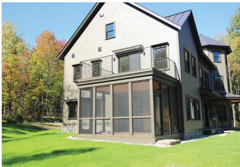
Figure 5. The rooftop deck has a custom-fabricated iron railing with a dark finish to match the home's color scheme.
