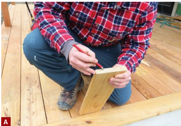
Figure 2. Known more as a “fence post” wood because of its strength and rot-resistance, black locust can also be milled into decking (A). It features a prominent grain and golden color (B), which will eventually develop a silvery gray patina.
