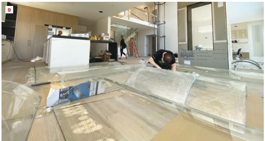
The shaftway frame is installed and secured to the basement (6) and first-floor framing (7) before the cab is wired up (8). The installation was managed by Savaria, the manufacturer, freeing the author from the delivery and long-term service of the unit. On this install, it helped that the jobsite had ample room to lay out the curved glass panels for the walls of the shaftway (9).
