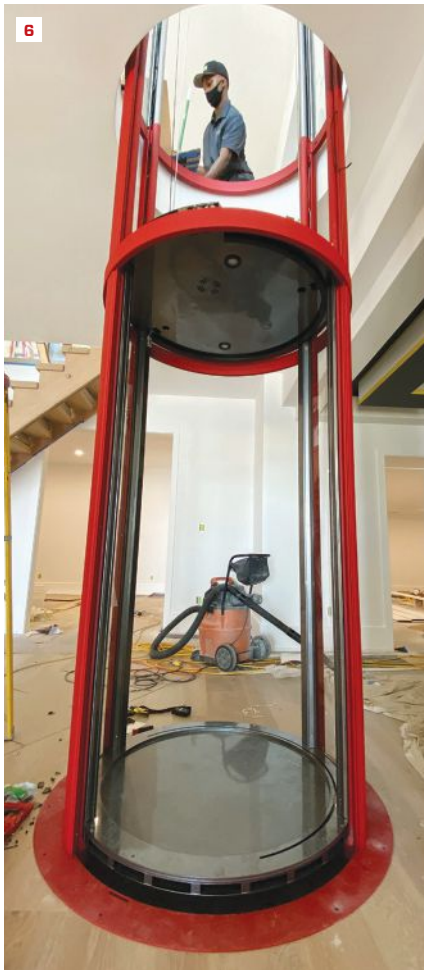
The shaftway frame is installed and secured to the basement (6) and first-floor framing (7) before the cab is wired up (8). The installation was managed by Savaria, the manufacturer, freeing the author from the delivery and long-term service of the unit. On this install, it helped that the jobsite had ample room to lay out the curved glass panels for the walls of the shaftway (9).
