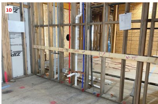
In this shower area, the green paint marked on the subfloor indicates the location for a linear drain; it overlaps the yellow marking for a shade pocket that was later eliminated from the plans (9). In the kitchen, a 2x4 fastened to the wall at countertop height and marked with the cabinet layout provides a convenient visual reference for clients and a precise layout reference for tradespeople (10). A free-standing full-scale mockup of the planned tub was built to help the homeowners visualize different locations for the tub within the bathroom space prior to plumbing rough-in (11).
