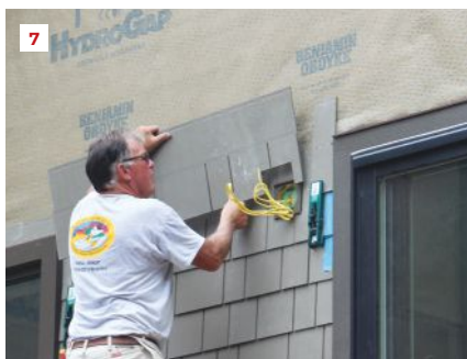
Co-author Carl Dudley measures from the butt end of the shingle (4) and carries the 48-inch-based panel pattern over the slider door (5); the remaining piece maintains the 16-inch offset (6). Thinner pieces need to be predrilled and nailed off by hand. The next panel is installed around a build-out block needed for a light fixture (7).
