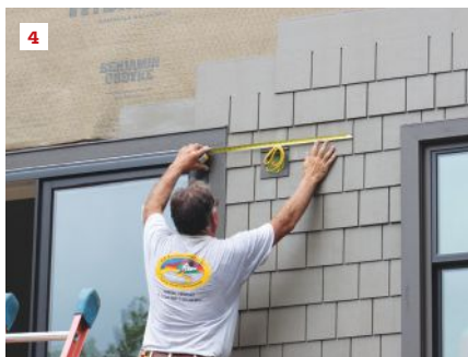
After the general contractor installed the Boral trim, the shingle panels were applied starting on garage wall façade (shown above on the far right). The installers clad the house clockwise, lining up the coursing around corners and eventually finishing up back at the garage façade (3).
