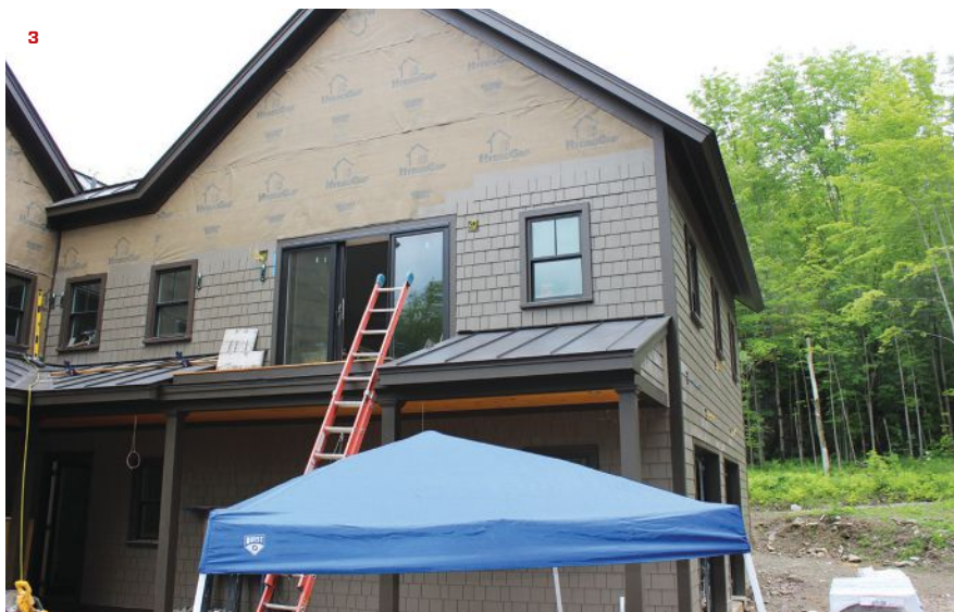
After the general contractor installed the Boral trim, the shingle panels were applied starting on garage wall façade (shown above on the far right). The installers clad the house clockwise, lining up the coursing around corners and eventually finishing up back at the garage façade (3).
