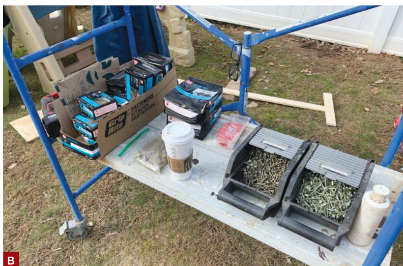
Figure 2. Horizontal surfaces invite being loaded up with random stuff, but a site-built miter saw stand can also double as a valuable work table (A). Even if not needed for working at height, a rolling scaffold offers a convenient spot for storing fasteners and other small items, and it can be rolled to where those items are needed (B).
