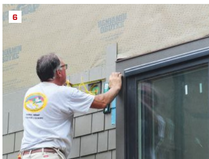
Co-author Carl Dudley measures from the butt end of the shingle (4) and carries the 48-inch-based panel pattern over the slider door (5); the remaining piece maintains the 16-inch offset (6). Thinner pieces need to be predrilled and nailed off by hand. The next panel is installed around a build-out block needed for a light fixture (7).
