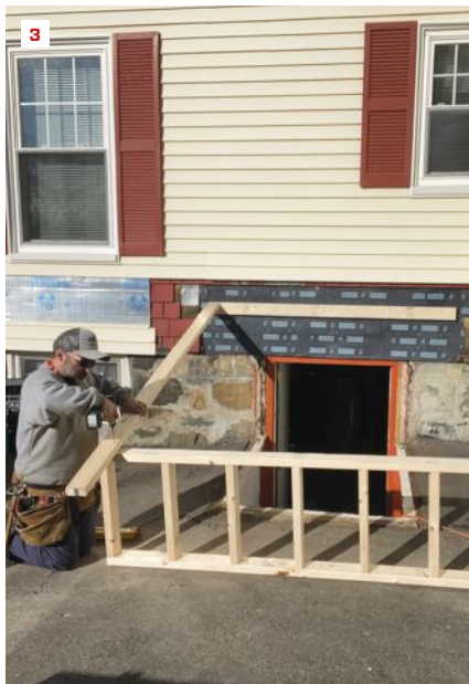
The author started by demolishing the bulkhead entry's existing stone steps (1) and clearing out the rubble (2). Next, he removed the vinyl siding and some underlying cedar shingles around the metal bulkhead door and framed a temporary shelter (3), then drilled holes in the old concrete and stonework for epoxied rebar dowels (4).
