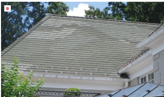
On a 10-year-old EcoStar slate installation, slates were mixed from different bundles per the manufacturer's instructions. Although the slates all looked the same upon installation, the color varied over time, appearing more natural (8).
