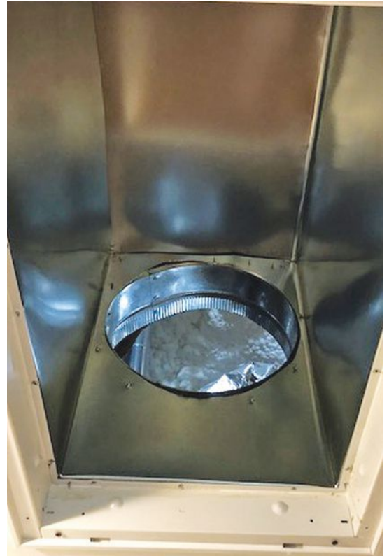
A shallow return (above) filter grille box results in a higher pressure drop across the filter. Replacing it with a deeper box (right) behind the filter succeeded in reducing the filter pressure drop by 30%.
