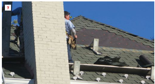
Snow guards with slim, sheet-metal legs are easier to install than traditional guards with heavy bars. Here, the individual stainless steel snow guards do not lift the shingles high (7).
