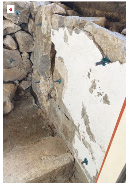
The author started by demolishing the bulkhead entry's existing stone steps (1) and clearing out the rubble (2). Next, he removed the vinyl siding and some underlying cedar shingles around the metal bulkhead door and framed a temporary shelter (3), then drilled holes in the old concrete and stonework for epoxied rebar dowels (4).
