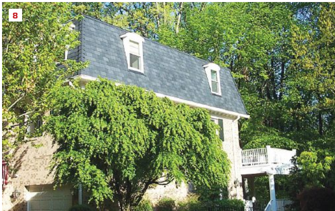
On a 10-year-old EcoStar slate installation, slates were mixed from different bundles per the manufacturer's instructions. Although the slates all looked the same upon installation, the color varied over time, appearing more natural (8).
