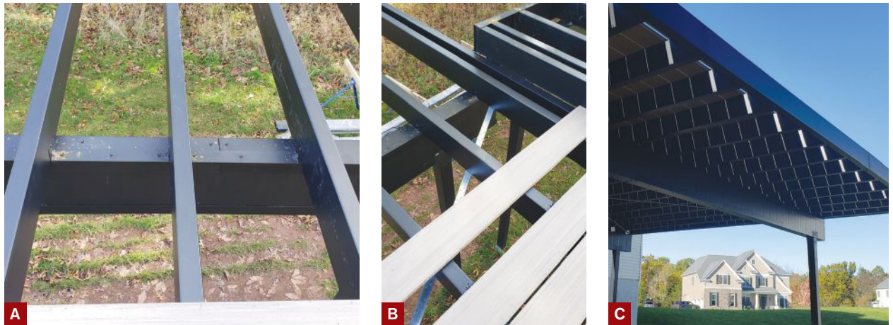
Figure 3. Evolution joists measure 2 inches by 6 inches and can be fastened to dropped beams either with 12- or 16-inch-on-center blocking brackets (A) or with F10 angle brackets (B). Cantilevers of up to 5 feet are possible with the steel joists, which here are capped at the ends with U-Rim Joist material (C). The maximum beam cantilever is 24 inches.
