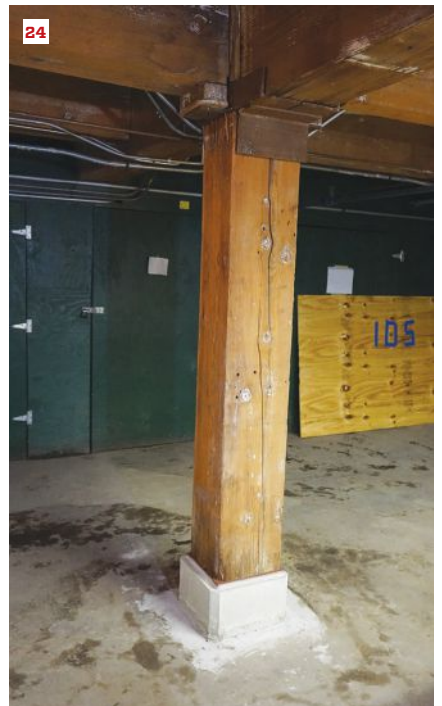
A 4x4 steel shim (19) sits in the middle of the new pier as the crew slides the cut post into position (20). The gap between the top of the pier and the setting plate (21) is soaked with water (22) before being filled with non-shrinking grout (23). Then all that's left to do is to remove the shoring around the completed post (24).
