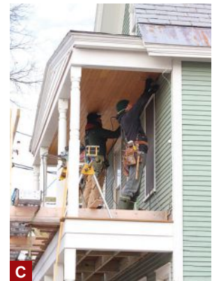
Figure 3. Per local code, the pressure-treated framing was covered with painted wood trim to help maintain the original look of the house; blocking between the framing and wood trim allows moisture to escape from the assembly (A). A local craftsman turned the custom 6x6 Douglas fir posts (B), which the author primed and painted prior to installation (C).
