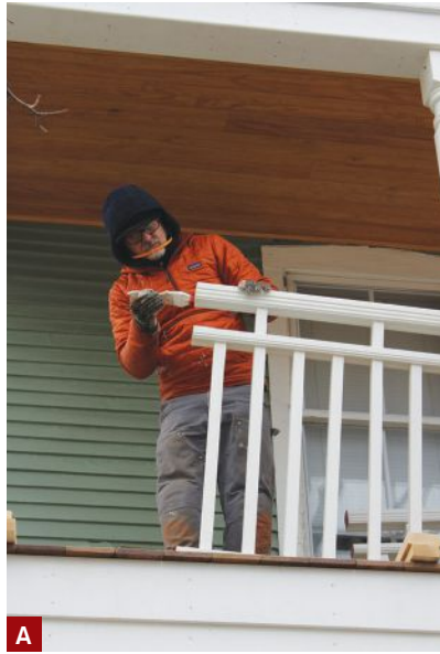
Figure 6. After cutting the rail sections on site to fit, Sean Laughlin sealed the end grain with primer (A) and then fastened the rails to the posts with structural screws (B). Making the railing connection at the house was complicated by the existing siding and trim (C).
