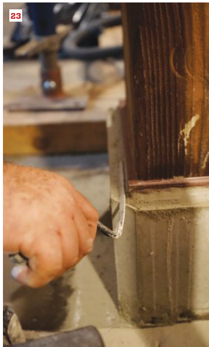
A 4x4 steel shim (19) sits in the middle of the new pier as the crew slides the cut post into position (20). The gap between the top of the pier and the setting plate (21) is soaked with water (22) before being filled with non-shrinking grout (23). Then all that's left to do is to remove the shoring around the completed post (24).
