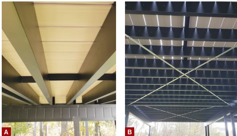
Figure 4. Where joist spans exceed 8 feet, midspan blocking is required, typically with Evolution prenotched 12- or 16-inch-on-center straps. Here, the straps simply lie across the tops of the joists and don't require fasteners (A), but they could be fastened to the underside of joists. Diagonal strapping was also added to the deck framing to reduce lateral movement (B).
