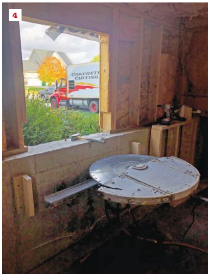
A typical occurrence at “grade floor openings” is that an existing window doesn’t meet minimum opening area requirements. Here, an existing double-hung window was removed and the opening enlarged (4). The author recommends erring on the side of caution when going to the expense of cutting concrete, with a maximum sill height of 42 inches off the finish floor (5, 6).
