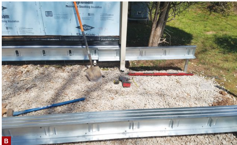
Figure 1. In the Evolution system, ledger brackets are screwed to the S-ledge, or fit into punched openings in the S-ledge without requiring additional fasteners (A). In comparison, an LGS ledger track has bent tabs for fastening the joists to the ledger (B) and requires five or more fasteners per joist-to-ledger connection. Evolution joists just slip over the brackets, and are held in place with a pair of screws per bracket (C).
