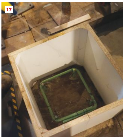
The crew drills into the existing footing for rebar pins (13). A vacuum, a wire brush, and a blow-out pump (14) are used to clean the holes before the pins are set with epoxy (15). The pier elevation is marked on the form with a combination square (16) and the form sprayed with water (17). Tapping the form with a dead-blow mallet settles the concrete and helps eliminate voids (18).
