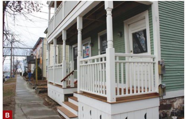
Figure 7. Post sleeves were fabricated from 1x6 stock using glued T&G box joints, which didn't require fasteners that would interfere with cutting the corner chamfers (A). The skirt around the base of the porch has screened cutouts that allow for ventilation while blocking out insects, cats, skunks, and other neighborhood pests (B).
