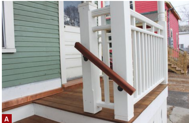
Figure 7. Post sleeves were fabricated from 1x6 stock using glued T&G box joints, which didn't require fasteners that would interfere with cutting the corner chamfers (A). The skirt around the base of the porch has screened cutouts that allow for ventilation while blocking out insects, cats, skunks, and other neighborhood pests (B).
