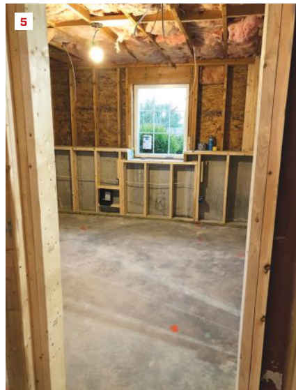
A typical occurrence at “grade floor openings” is that an existing window doesn’t meet minimum opening area requirements. Here, an existing double-hung window was removed and the opening enlarged (4). The author recommends erring on the side of caution when going to the expense of cutting concrete, with a maximum sill height of 42 inches off the finish floor (5, 6).
