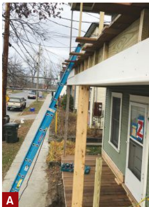
Figure 3. Per local code, the pressure-treated framing was covered with painted wood trim to help maintain the original look of the house; blocking between the framing and wood trim allows moisture to escape from the assembly (A). A local craftsman turned the custom 6x6 Douglas fir posts (B), which the author primed and painted prior to installation (C).
