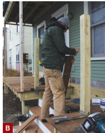
Figure 2. The author installed dense tropical hardwood decking, orienting the boards perpendicular to the house to mimic the traditional look of tongue-and-groove porch flooring (A). While the decking was left unfinished to reduce maintenance costs, the ends were treated with a wax sealer (B).
