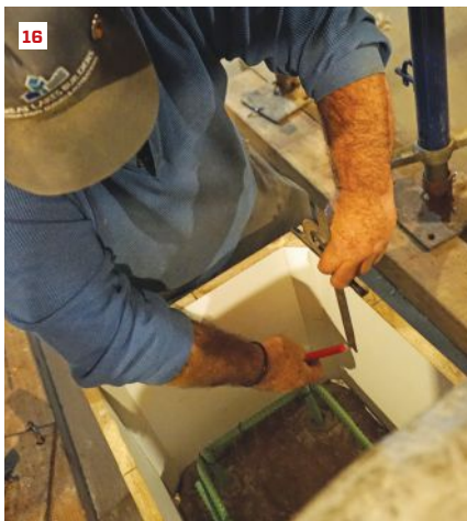
The crew drills into the existing footing for rebar pins (13). A vacuum, a wire brush, and a blow-out pump (14) are used to clean the holes before the pins are set with epoxy (15). The pier elevation is marked on the form with a combination square (16) and the form sprayed with water (17). Tapping the form with a dead-blow mallet settles the concrete and helps eliminate voids (18).
