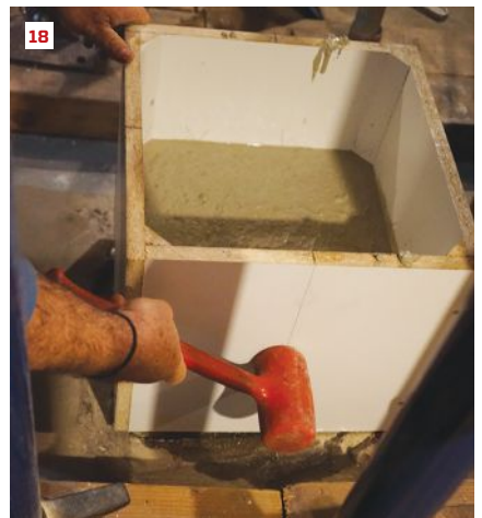
The crew drills into the existing footing for rebar pins (13). A vacuum, a wire brush, and a blow-out pump (14) are used to clean the holes before the pins are set with epoxy (15). The pier elevation is marked on the form with a combination square (16) and the form sprayed with water (17). Tapping the form with a dead-blow mallet settles the concrete and helps eliminate voids (18).
