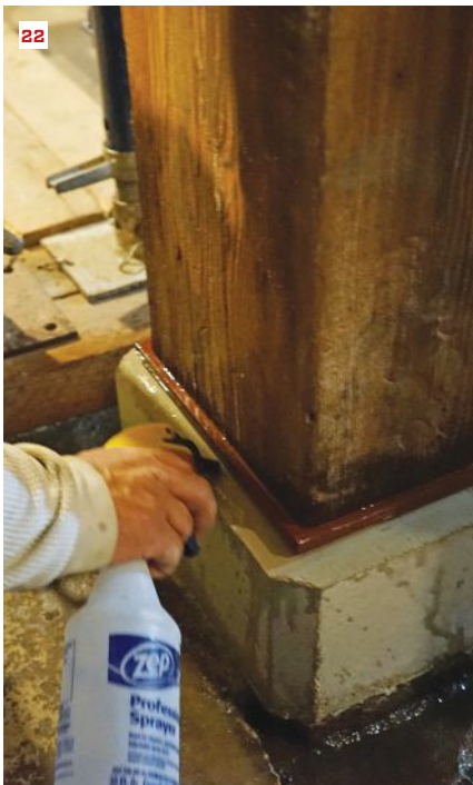
A 4x4 steel shim (19) sits in the middle of the new pier as the crew slides the cut post into position (20). The gap between the top of the pier and the setting plate (21) is soaked with water (22) before being filled with non-shrinking grout (23). Then all that's left to do is to remove the shoring around the completed post (24).
