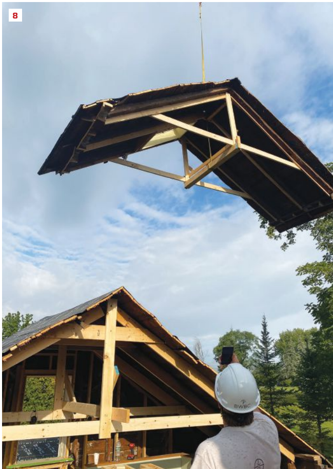
On the day of the lift, workers cut the old roof into three sections, which they had reinforced with truss-like framing prior to removal (8). The lifting straps were threaded through small openings cut into the roof sheathing at the ridge (9). With the roof removed and the balloon-framed gable end walls exposed, the structure was ready for its new roof (10).
