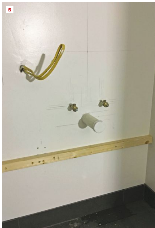
The existing conditions are precisely plotted on the wall (5). Layout marks include the cabinet's centerline, the top of the vanity, and plumbing and electrical centerlines (see illustration, above).
