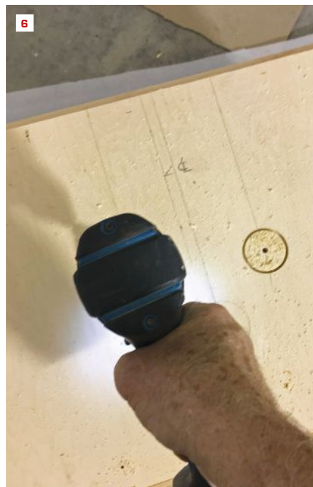
The existing conditions are precisely plotted on the wall (5). Layout marks include the cabinet's centerline, the top of the vanity, and plumbing and electrical centerlines (see illustration, above).
