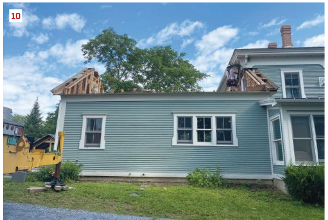
On the day of the lift, workers cut the old roof into three sections, which they had reinforced with truss-like framing prior to removal (8). The lifting straps were threaded through small openings cut into the roof sheathing at the ridge (9). With the roof removed and the balloon-framed gable end walls exposed, the structure was ready for its new roof (10).
