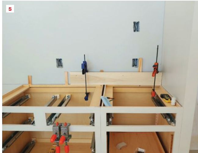
Where base cabinets terminate at a wall or tall cabinet, the author shims them as needed up to the level line (4). Preassembling runs of cabinets where possible and using plenty of clamps during installation helps keep the cabinets square to one another (5), while a string line stretched across the faces of the cabinets helps keep them aligned as they are shimmed to the wall (6).
