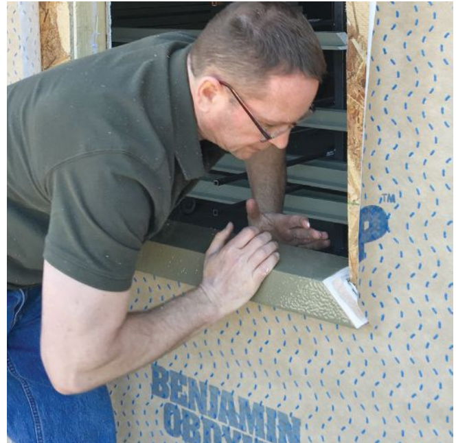
Sheathing can be applied outboard of the foam (above left). This lets the sheathing dry to the outside. ThermalBuck (above right), an insulated window mounting system, creates a positive attachment for the window while limiting thermal bridging.
