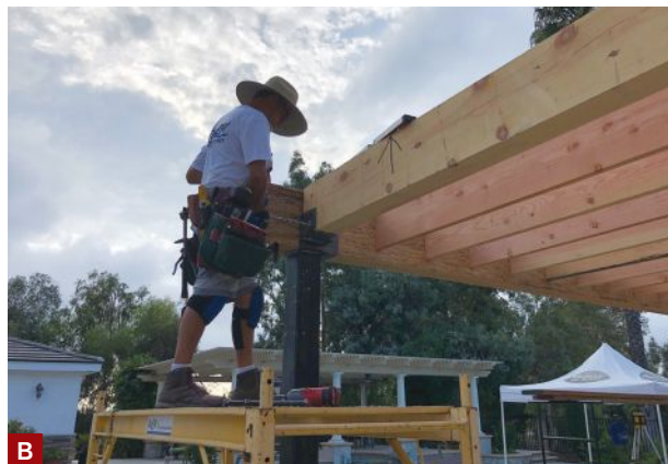
Figure 3. Instead of a ledger, a 7x14 PSL flush carrying beam (one was also installed at the outside edge of the deck) provided support for the freestanding deck at the house (A). To complete the seismic design, the inside and outside carrying beams were connected to each other with 6x12 Doug fir beams, which were fastened with \frac{3}{4} -inch-diameter through-bolts to brackets welded to the steel columns (B). 2x12 Doug fir joists were hung from the carrying beams, which were blocked out with 2x12s sandwiched around the 4x4 deck posts bolted to the framing (C). Because the entire deck would be protected by a waterproofing system, non-PT-treated material and engineered lumber was used in its construction.
