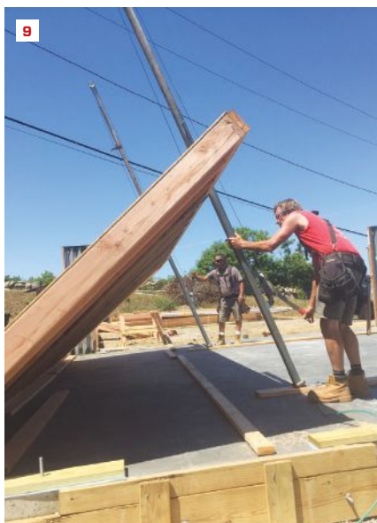
After the wall sheathing is nailed off, the wall can be lifted into place on top of the sill plate (here, the author is using wall jacks) (9); leaving the anchor bolts loose allows for adjustment as the remaining walls are raised. Diagonal bracing holds the walls in position (10) as the project moves into the next phase: roof framing (11).
