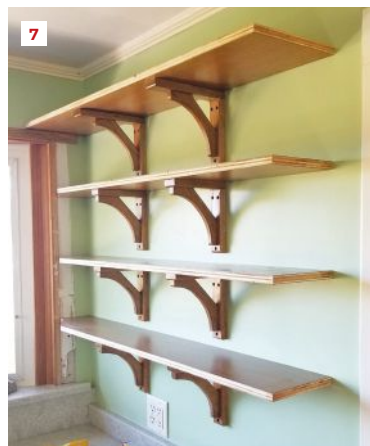
The vintage, glass-front metal cabinet in the original kitchen (6) was relocated and replaced with shop-built oak shelves (shown here without the edging or wall cleats installed) in the remodel (7).
