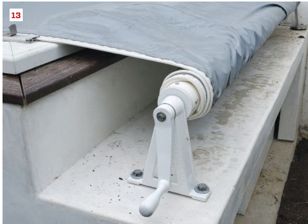
An abutting deck with bench seating was installed, with an access panel to the hydrotherapy jets built into the seating (11). A floating skimmer for the filter intake is housed next to the propulsion fan unit (12). The hand crank for the manually operated security pool cover was mounted to the mechanical equipment housing (13). The finished modular-style Endless Pool (14).
