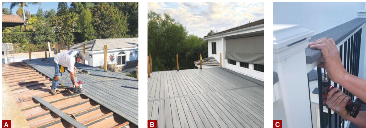
Figure 6. The Trex decking was fastened down with FusionLoc fasteners, installed with FastenMaster's FiveShot collated nail gun (A). To provide extra clearance between the underside of the decking and the RainEscape troughs and to improve drainage, 1-by-PT rippings were installed on top of the butyl tape used to seal the troughs where they lapped over the joists. Note that the worker is standing on a double joist, the location of a seam board in the middle of the 37-foot-wide deck that provides a transition point for the decking (B). After the post sleeves and railing system were installed, workers screwed on sections of drink rail fabricated from the same decking, which span between posts (C). The screws thread into inserts installed on the underside of the drink rail.
