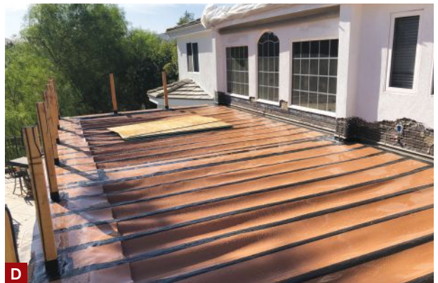
Figure 4. Water collected by the under-deck drain system flows toward the outside edge of the deck, where it empties into a one-piece gutter (A). The gutter slopes toward a corner column, where it is drained by a 3-inch-diameter downspout concealed within the boxed column (B). Trex RainEscape downspouts (C) empty the water collected by the troughs, which are draped over the tops of the joists (D). At the house, a custom-fabricated flashing and weep screed tie the WRB behind the stucco to the deck waterproofing system.
