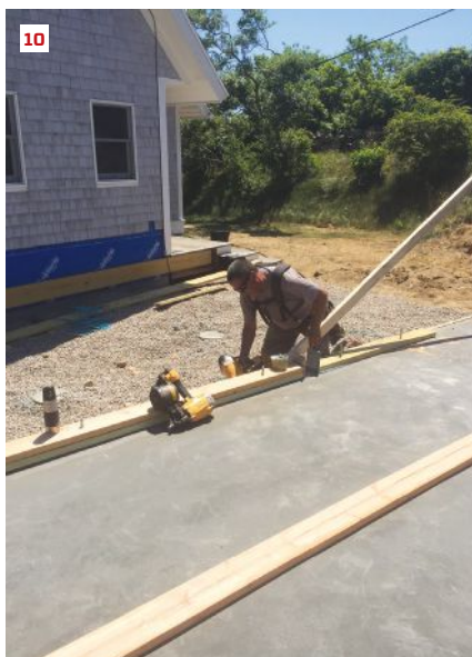
After the wall sheathing is nailed off, the wall can be lifted into place on top of the sill plate (here, the author is using wall jacks) (9); leaving the anchor bolts loose allows for adjustment as the remaining walls are raised. Diagonal bracing holds the walls in position (10) as the project moves into the next phase: roof framing (11).
