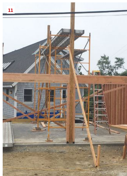
After the wall sheathing is nailed off, the wall can be lifted into place on top of the sill plate (here, the author is using wall jacks) (9); leaving the anchor bolts loose allows for adjustment as the remaining walls are raised. Diagonal bracing holds the walls in position (10) as the project moves into the next phase: roof framing (11).
