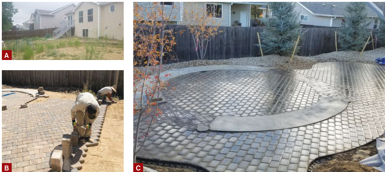
Figure 1. The barren backyard once had a small deck and an above-ground pool, which had long since been retired (A). The outdoor environment that the author designed featured a paver patio (B) and a new, larger deck. A pair of semi-circular concrete pads (C) mark the location of the grain silo pergola, the centerpiece of the project.
