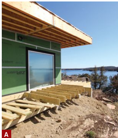
Figure 3. In the slab-on-grade areas, the wider grade-level deck section was framed with beefier 2-by stock (A). Threaded rod set in adhesive attached the ledgers to the top of the frost walls (B). Peel-and-stick capped the 2-by stock.
