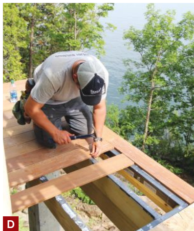
Figure 4. The ipe decking was installed on the elevated deck area first (A). Cut ends were sealed (B) and the decking was predrilled for stainless steel trim screws (C). A couple of 8d nails helped uniformly gap the boards (D).
