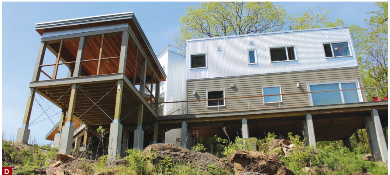
Figure 6. A custom-built guardrail with cable railing was installed (A). The deck was temporarily treated as two separate decks with code-approved guardrails (B, C). Guardrails and decking were reconfigured during the pavilion work (D).
