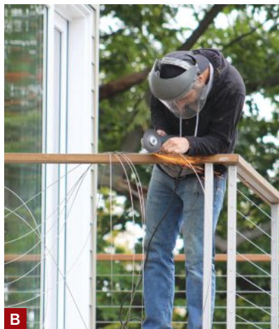
Figure 6. A custom-built guardrail with cable railing was installed (A). The deck was temporarily treated as two separate decks with code-approved guardrails (B, C). Guardrails and decking were reconfigured during the pavilion work (D).
