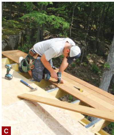
Figure 4. The ipe decking was installed on the elevated deck area first (A). Cut ends were sealed (B) and the decking was predrilled for stainless steel trim screws (C). A couple of 8d nails helped uniformly gap the boards (D).
