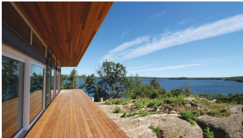
Figure 5. The south elevation was 80% glass. Large high-performance European-style lift-and-slide glass doors set in a steel moment frame (left exposed as an architectural feature) opened onto the ipe deck.
