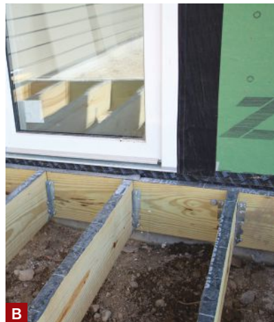
Figure 3. In the slab-on-grade areas, the wider grade-level deck section was framed with beefier 2-by stock (A). Threaded rod set in adhesive attached the ledgers to the top of the frost walls (B). Peel-and-stick capped the 2-by stock.
