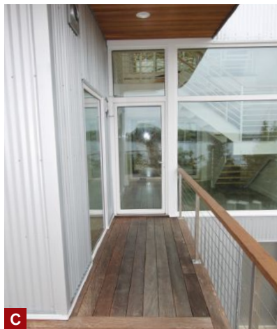
Figure 6. A custom-built guardrail with cable railing was installed (A). The deck was temporarily treated as two separate decks with code-approved guardrails (B, C). Guardrails and decking were reconfigured during the pavilion work (D).
