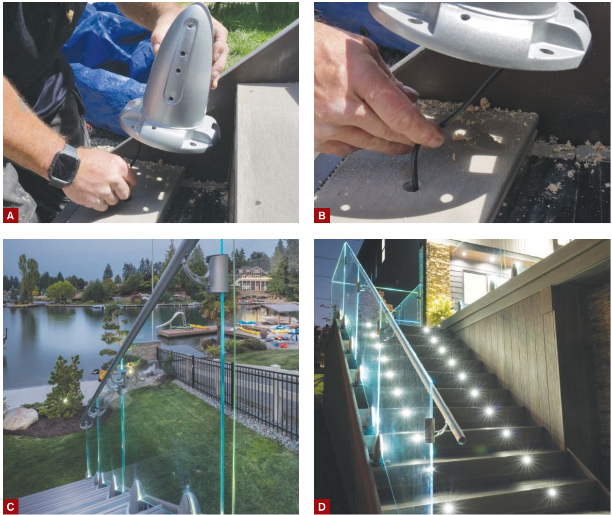
Figure 5. One of the most striking lighting fixtures that the author has used on his projects is the CrystalRail system, from Regal Ideas, which consists of aluminum mounting brackets (A) with built-in LED lighting that connects to the deck's low-voltage system (B). The LED fixtures in the mounting bases illuminate tempered-glass panels that are part of the system, providing a dramatic nighttime look to the deck from all directions (C, D).
