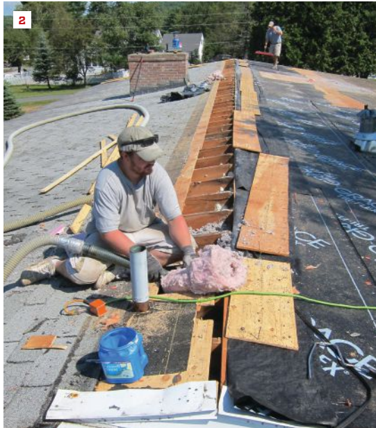
Where access from below is impractical, cellulose can be dense-packed into existing rafter bays from the roof ridge (2) . In new construction, the author recommends packing the material behind strapped Insulweb fabric (3) .
