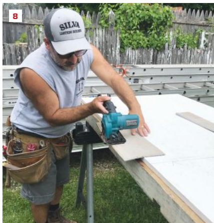
The author trims enough of the first inside corner shingle so that the edge is flush with the wall (5, 6), tacks the shingle in place, and uses a compass to scribe the flare on the opposing shingle (7). Then he cuts (8) and planes (9) the shingle to the scribe line before tacking it to the furring strips with 2-inch ring-shank siding nails (10).
