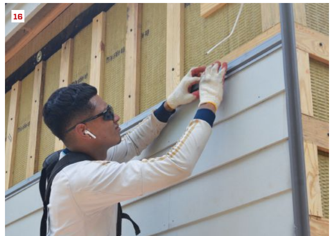
The shell has a continuous blanket of Rockwool (13). Strapping holds the insulation in place and provides nailing for the siding. The roofers install standing-seam metal roofing (14, 15). The siding crew installs Fry Reglet metal trim pieces (16).
