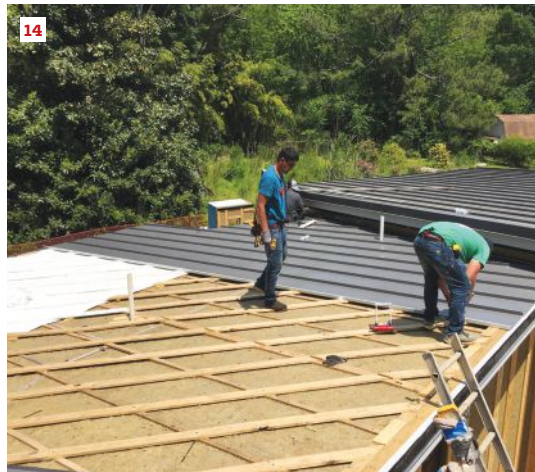
The shell has a continuous blanket of Rockwool (13). Strapping holds the insulation in place and provides nailing for the siding. The roofers install standing-seam metal roofing (14, 15). The siding crew installs Fry Reglet metal trim pieces (16).
