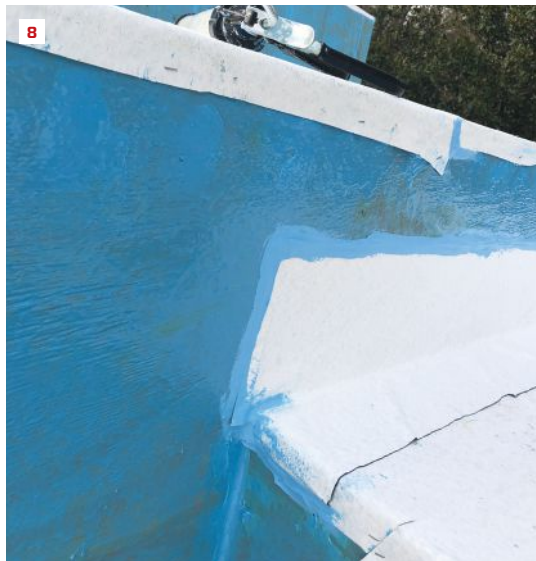
The painters apply Blue Barrier Flash 'N Wrap 2400 to a window rough opening (5), roll Liquid Wrap 2300 onto the field of the wall (6), and detail a window flange with Joint Filler 2200 (7). At the wall top, the overhanging peel-and-stick underlayment is sealed to the wall with Joint Filler 2200 and Liquid Wrap 2300 (8).
