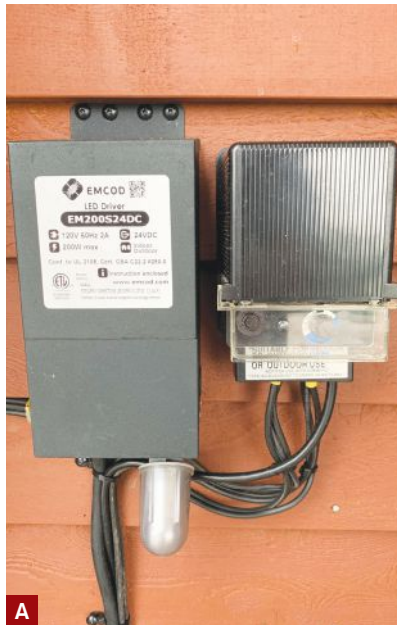
Figure 1. Most LED lighting systems can be powered by a 12-volt DC transformer, but some systems are designed to operate at 24 volts DC (A). This 24-volt DC unit has an external programmable photoelectric sensor (B).
