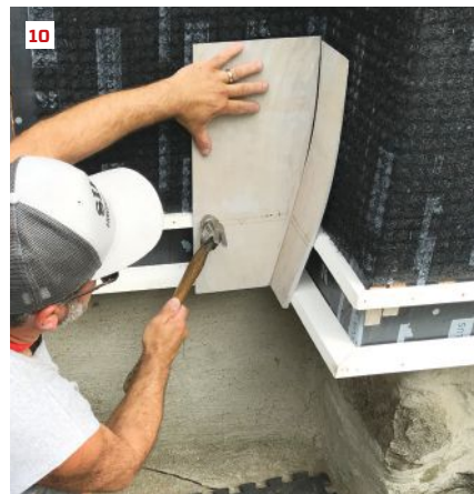
The author trims enough of the first inside corner shingle so that the edge is flush with the wall (5, 6), tacks the shingle in place, and uses a compass to scribe the flare on the opposing shingle (7). Then he cuts (8) and planes (9) the shingle to the scribe line before tacking it to the furring strips with 2-inch ring-shank siding nails (10).
