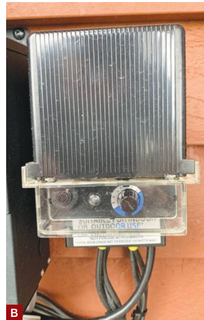
Figure 1. Most LED lighting systems can be powered by a 12-volt DC transformer, but some systems are designed to operate at 24 volts DC (A). This 24-volt DC unit has an external programmable photoelectric sensor (B).
