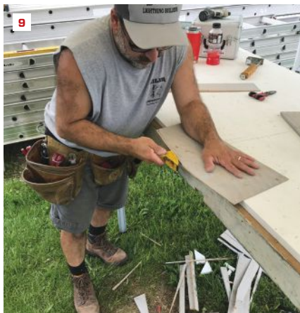
The author trims enough of the first inside corner shingle so that the edge is flush with the wall (5, 6), tacks the shingle in place, and uses a compass to scribe the flare on the opposing shingle (7). Then he cuts (8) and planes (9) the shingle to the scribe line before tacking it to the furring strips with 2-inch ring-shank siding nails (10).
