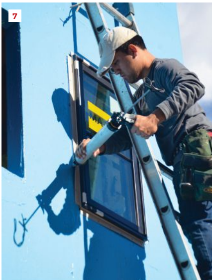
The painters apply Blue Barrier Flash 'N Wrap 2400 to a window rough opening (5), roll Liquid Wrap 2300 onto the field of the wall (6), and detail a window flange with Joint Filler 2200 (7). At the wall top, the overhanging peel-and-stick underlayment is sealed to the wall with Joint Filler 2200 and Liquid Wrap 2300 (8).
