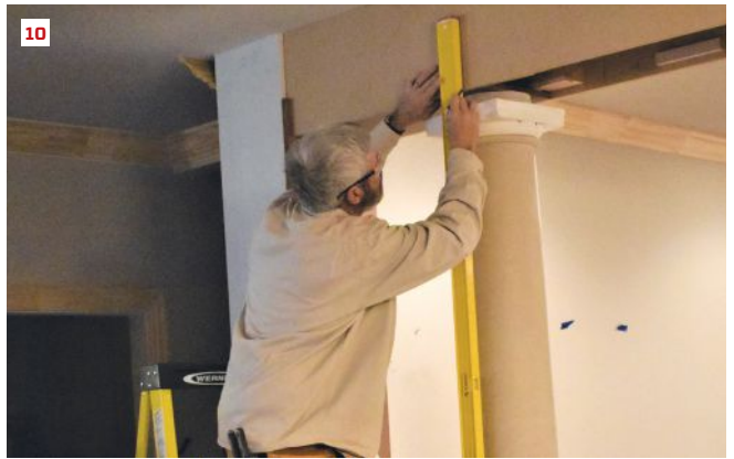
The author used a flexible wood batten to mark the cut lines on the round columns (9). To help ensure that the tapered columns were installed plumb, he used a spirit level to align the centerlines that he marked on the columns' capitals and bases (10).
