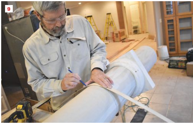
The author used a flexible wood batten to mark the cut lines on the round columns (9). To help ensure that the tapered columns were installed plumb, he used a spirit level to align the centerlines that he marked on the columns' capitals and bases (10).
