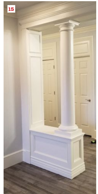
Panel molding was also used to create the simple frame-and-panel detail on the pilasters (13). Once completed (14) and painted (15), the classic room divider helps define the transition between the entry foyer and the living room.
