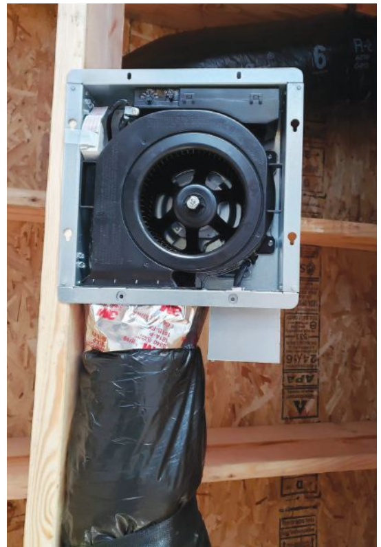
The author places a Panasonic WhisperValue fan, one of seven in the 3,800-square-foot house (above left). A look inside the housing shows the controls inside the fan that allow the installer to select an exhaust airflow of 50, 80, or 100 cfm (above right). The relative humidity set point of the room can also be dialed in for the condensation sensor.
