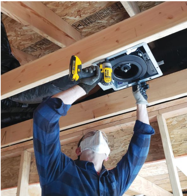
The author places a Panasonic WhisperValue fan, one of seven in the 3,800-square-foot house (above left). A look inside the housing shows the controls inside the fan that allow the installer to select an exhaust airflow of 50, 80, or 100 cfm (above right). The relative humidity set point of the room can also be dialed in for the condensation sensor.
