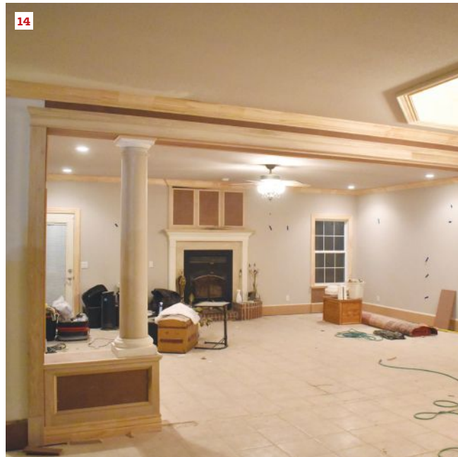
Panel molding was also used to create the simple frame-and-panel detail on the pilasters (13). Once completed (14) and painted (15), the classic room divider helps define the transition between the entry foyer and the living room.
