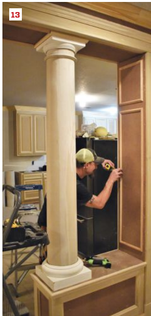
Panel molding was also used to create the simple frame-and-panel detail on the pilasters (13). Once completed (14) and painted (15), the classic room divider helps define the transition between the entry foyer and the living room.
