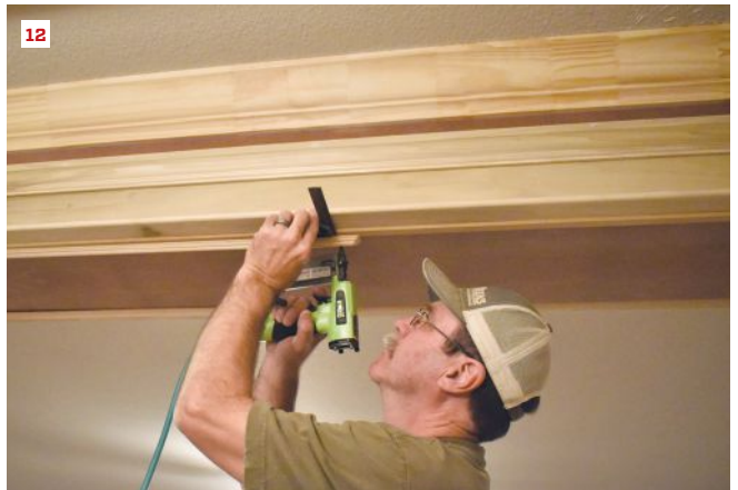
A number of different elements were used to trim out the false beam, starting with another wide MDF band applied to the sides of the beam, followed by a 1/2-inch-by-2-inch bead (11) and other panel and crown molding profiles (12).
