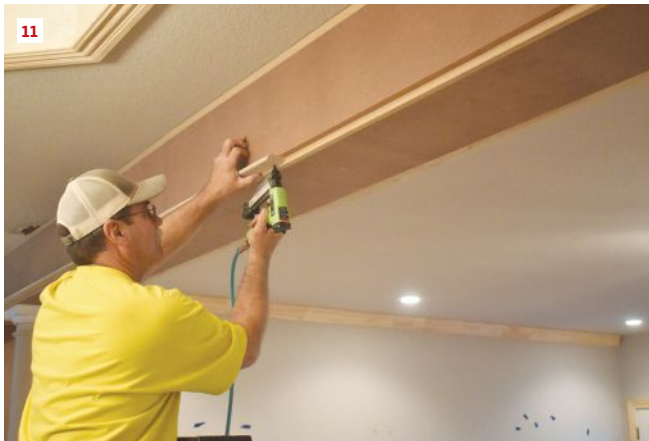
A number of different elements were used to trim out the false beam, starting with another wide MDF band applied to the sides of the beam, followed by a 1/2-inch-by-2-inch bead (11) and other panel and crown molding profiles (12).
