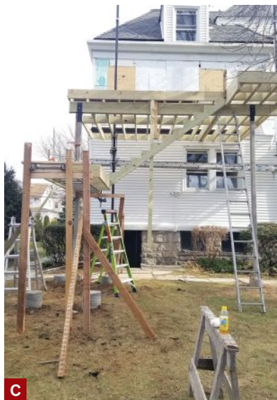
Figure 1. The second-story deck is supported by a double 2x12 steel-reinforced beam that bears on 4x4 steel columns (A). After cutting the first stringer, the author used it to determine the elevation of the midpoint landing (B), which was framed on the ground, then lifted into position on temporary supports (C). The outside stringer was then used to fine-tune the orientation of the landing (D).
