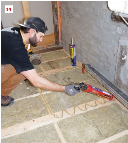
Hovious cuts Rockwool insulation to fit a cavity (11), splits a batt for thickness (12), and installs a batt into the cavity (13). He applies subfloor adhesive to a reinforced joist (14), slides the AdvanTech subfloor into place (15), and fastens the AdvanTech down to the floor framing with 2 1 / 2 -inch GRK screws (16).
