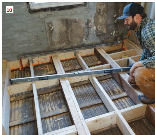
The circular-saw blade did not cut all the way through the 3-inch joist. Here, Warren O'Shea finishes the cut with a recip saw (5). O'Shea applies construction adhesive to a ledger header (6) and screws the header to the existing joist (7). Hovious scribes a 2x8 sister along the existing joist (8). Carpenter Mike Raulston attaches the sister (9). Hovious checks the framing for flatness (10).
