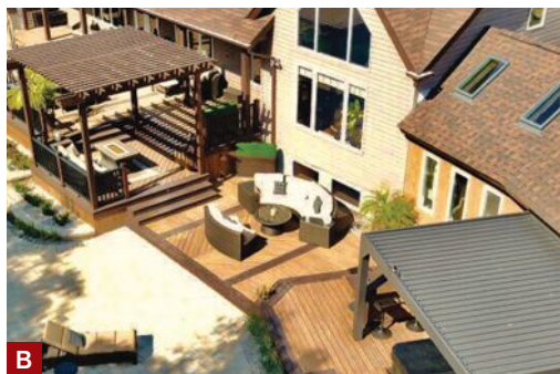
Figure 2. A herringbone pattern formed by decking installed on the diagonal helps define a sitting area on a large composite deck (A). On a deck with multiple levels, contrasting borders, seam boards, and treads can be used to define transitions between areas and make the deck safer (B).
