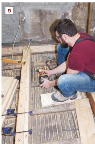
The circular-saw blade did not cut all the way through the 3-inch joist. Here, Warren O'Shea finishes the cut with a recip saw (5). O'Shea applies construction adhesive to a ledger header (6) and screws the header to the existing joist (7). Hovious scribes a 2x8 sister along the existing joist (8). Carpenter Mike Raulston attaches the sister (9). Hovious checks the framing for flatness (10).
