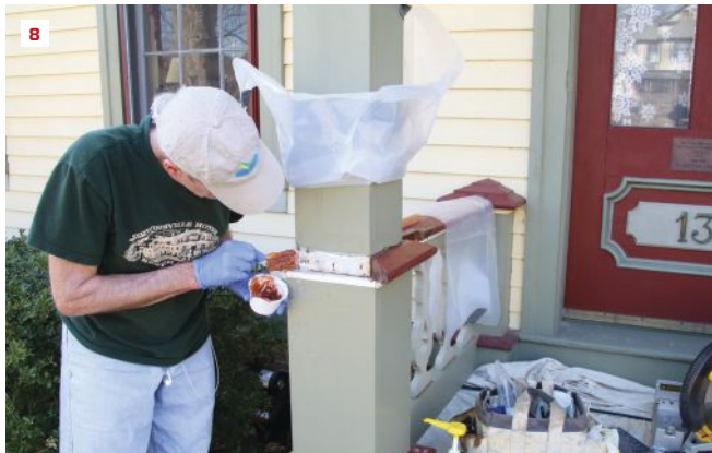
Marine epoxy adhesive ensures that miter joints that are exposed to the elements won't separate (8).
