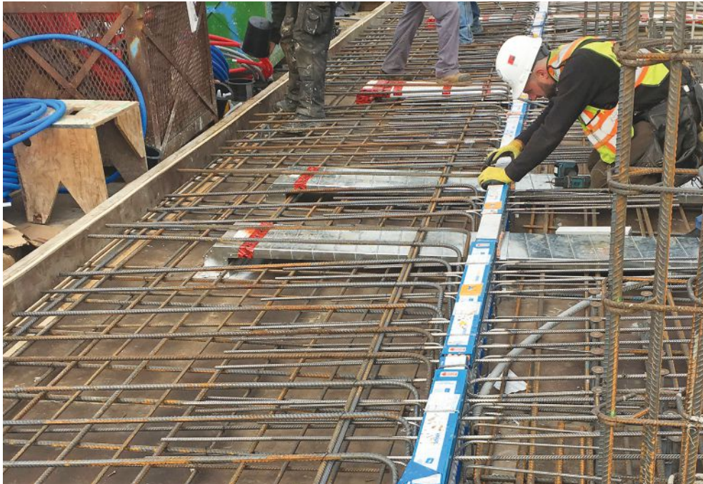
The Isokorb thermal break from Schöck creates an insulated structural connection between a balcony and the main floor slab of the building. The engineered connection is installed before concrete is poured, and it's integrated into the rebar mat of the slab.
