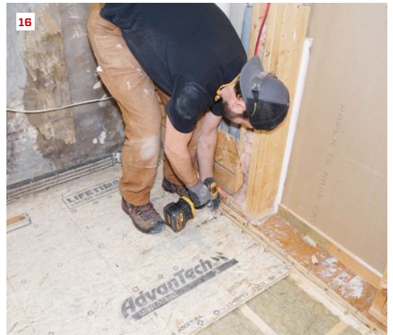
Hovious cuts Rockwool insulation to fit a cavity (11), splits a batt for thickness (12), and installs a batt into the cavity (13). He applies subfloor adhesive to a reinforced joist (14), slides the AdvanTech subfloor into place (15), and fastens the AdvanTech down to the floor framing with 2 1 / 2 -inch GRK screws (16).
