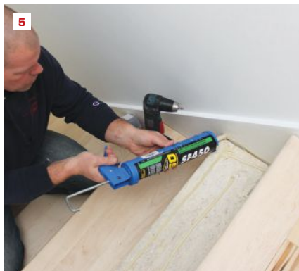
The author applies gel-foam adhesive on both sides of the 2x4 stringer spacer (1). He uses the same adhesive on the carriage (2) to secure subreads before nailing them off (3). A Stair Wizard proves essential for laying out custom-cut treads between finish stringers (4). Working from the top, he applies construction adhesive to the subread (5), and then clamps the finish treads (6).
