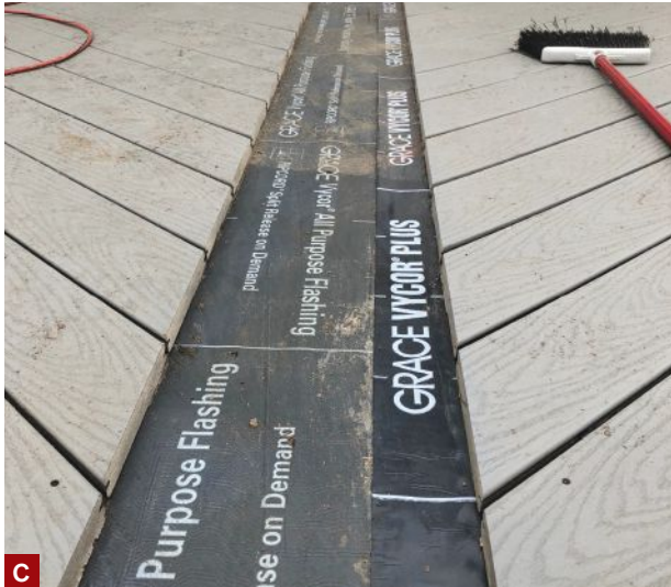
Figure 3. Blocking installed on the flat (A) doesn't drain as well as vertical blocking, so it should be protected with self-sealing flashing. When you're trimming the ends of decking installed on the diagonal (B), the depth of cut should be slightly less than the thickness of the decking to avoid cutting through the flashing membrane (C). By installing a seam board and chevron pattern, builder Mike Valente was able to avoid butt joints in the decking (D).
