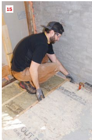
Hovious cuts Rockwool insulation to fit a cavity (11), splits a batt for thickness (12), and installs a batt into the cavity (13). He applies subfloor adhesive to a reinforced joist (14), slides the AdvanTech subfloor into place (15), and fastens the AdvanTech down to the floor framing with 2 1 / 2 -inch GRK screws (16).
