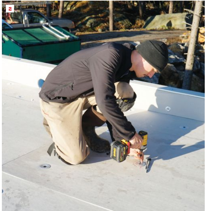
The crew builds the roof up with tapered sheets of foam, constructing valleys that lead to scupper locations in the downslope parapet wall (1). The foam buildup is fastened down with long FastenMaster screws (2).
