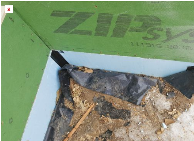
Continuous exterior insulation protects against thermal bridging at studs (1). Bumping the sill plate out allows thick foundation insulation to align with the wall's face, simplifying drainage, air-sealing, and exterior finishes (2). These clad vinyl-frame windows (3, 4) have an integral flange that allows for standard installation: no need for window bucks or elaborate flashing.
