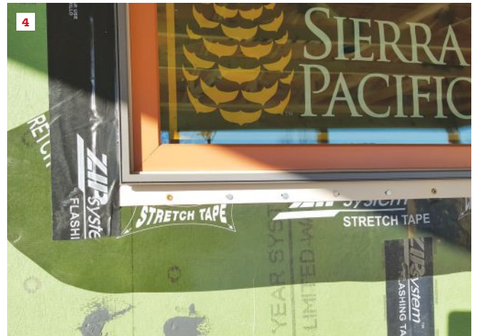
Continuous exterior insulation protects against thermal bridging at studs (1). Bumping the sill plate out allows thick foundation insulation to align with the wall's face, simplifying drainage, air-sealing, and exterior finishes (2). These clad vinyl-frame windows (3, 4) have an integral flange that allows for standard installation: no need for window bucks or elaborate flashing.
