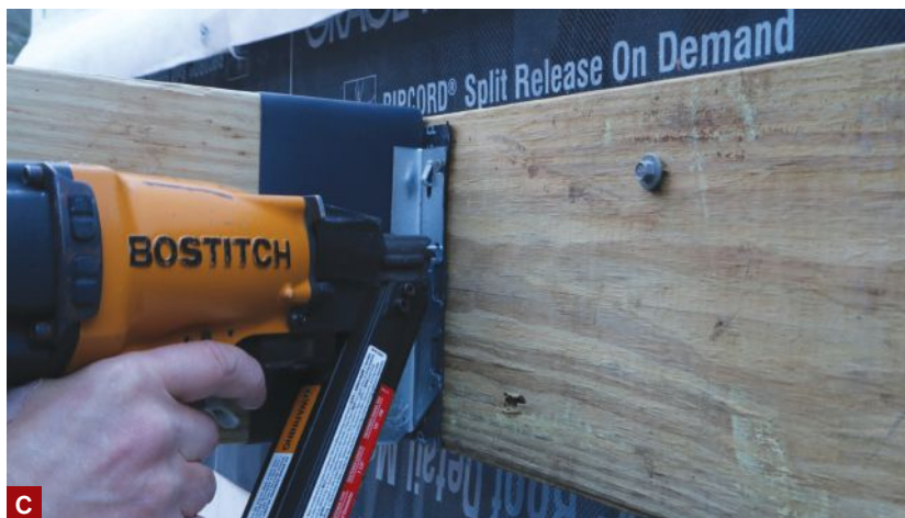
Figure 6. Paslode's pneumatic metal-connector nailer (A) and DeWalt's battery-powered nailer (B) have probe tips to guide nails into the hardware holes. Bostitch's pneumatic nailer (C) exposes the nail tip, which is placed in the hole before the gun is fired. Placement is critical since a misfire can damage the joist hanger or send a nail hurling back towards the operator.
