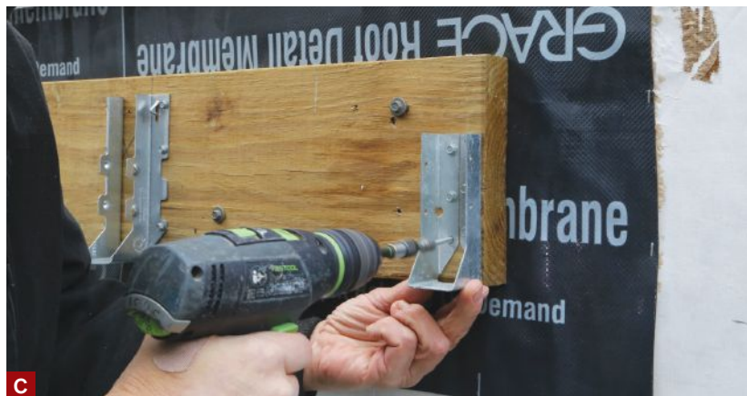
Figure 1. Hangers can be used with both their matching nominal joist size and the next size up—2x10 hangers are approved for use with 2x10s and 2x12s, for example (A). Concealed-flange hangers (B) are designed for use at the end of a ledger (C) but can also be used to avoid conflicts with lateral load hardware.
