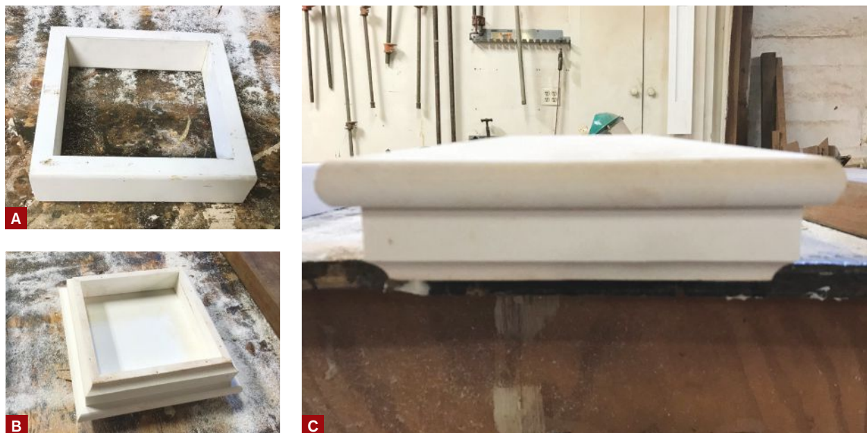
Figure 3. Cut from \frac{3}{4} -inch-by-1 \frac{1}{2} -inch PVC, the sleeve bases (A) and cap trim (B) were sized to fit snugly over the post sleeves. The cap trim boxes were nailed and glued to the caps, which were cut from 1 \frac{1}{4} -inch-thick PVC stock (C).
