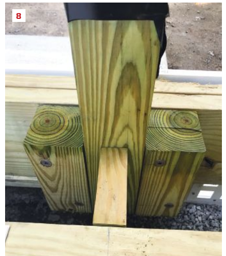
The author applies strips of flashing membrane to PT framing before installing joist hangers and other hardware (5). Self-adhering flashing protects the top edge of doubled beams (6), while shims create drainage gaps between trim and framing, or between some framing members (7). Blocking strengthens the connection between guard posts and the framing (8).
