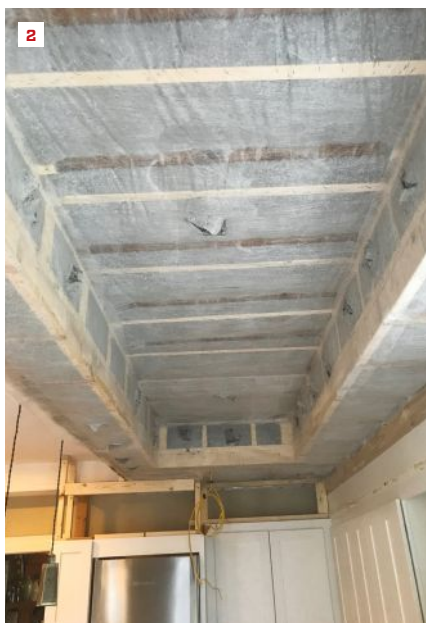
After removing the water-damaged kitchen ceiling, the author framed the structure for the tray ceiling (1). To hold the blown-in insulation in the cramped “attic” above the tray, the insulation sub attached netting to the underside of the frame (2). After installing plywood to the top and sides of the tray for attaching the tin veneer, the crew drywalled and taped off the ceiling (3).
