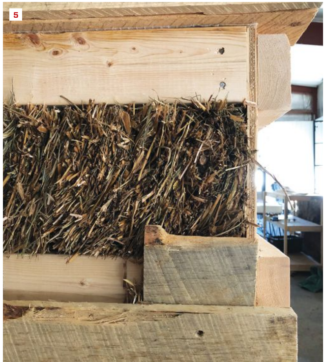
Panel assembly takes place on tables at a convenient working height (4). This panel has Gutex fiberboard insulation, rainscreen strapping, and corner protection applied. Above, a closeup of the panel in cross section (5).
