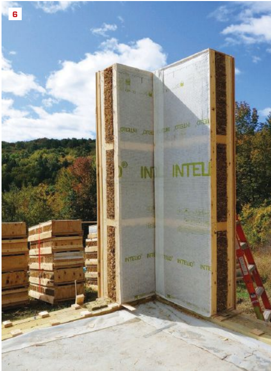
Panels are set on site using telehandler forklifts. Above, a corner has been assembled from two panels on site (6). The completed walls of the house sit ready for roof trusses (7).
