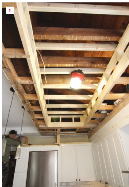
After removing the water-damaged kitchen ceiling, the author framed the structure for the tray ceiling (1). To hold the blown-in insulation in the cramped “attic” above the tray, the insulation sub attached netting to the underside of the frame (2). After installing plywood to the top and sides of the tray for attaching the tin veneer, the crew drywalled and taped off the ceiling (3).
