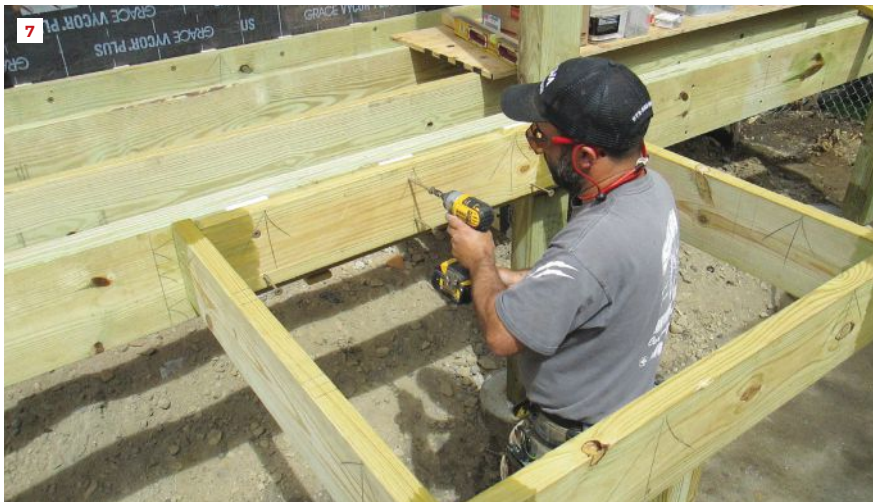
The author applies strips of flashing membrane to PT framing before installing joist hangers and other hardware (5). Self-adhering flashing protects the top edge of doubled beams (6), while shims create drainage gaps between trim and framing, or between some framing members (7). Blocking strengthens the connection between guard posts and the framing (8).
