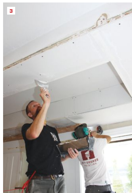
After removing the water-damaged kitchen ceiling, the author framed the structure for the tray ceiling (1). To hold the blown-in insulation in the cramped “attic” above the tray, the insulation sub attached netting to the underside of the frame (2). After installing plywood to the top and sides of the tray for attaching the tin veneer, the crew drywalled and taped off the ceiling (3).
