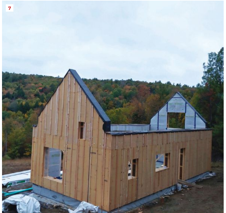
Panels are set on site using telehandler forklifts. Above, a corner has been assembled from two panels on site (6). The completed walls of the house sit ready for roof trusses (7).
