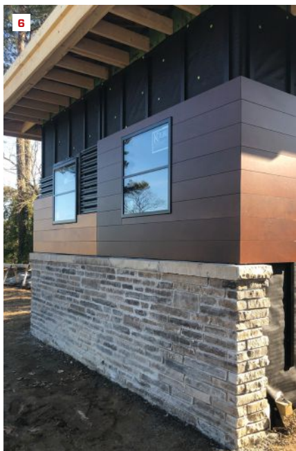
A full-scale mockup allows clients to visualize the difference between raked and full mortar joints in the stone cladding and the mitered Parklex cladding corner detail (6), and the effect of using a narrower, 4-inch version of the cladding for the soffit (7).
