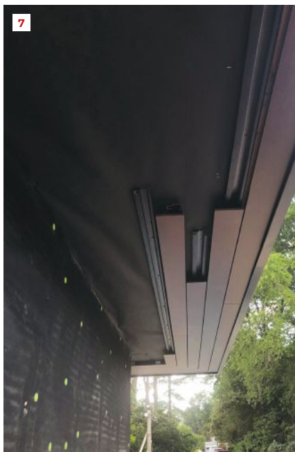
A full-scale mockup allows clients to visualize the difference between raked and full mortar joints in the stone cladding and the mitered Parklex cladding corner detail (6), and the effect of using a narrower, 4-inch version of the cladding for the soffit (7).
