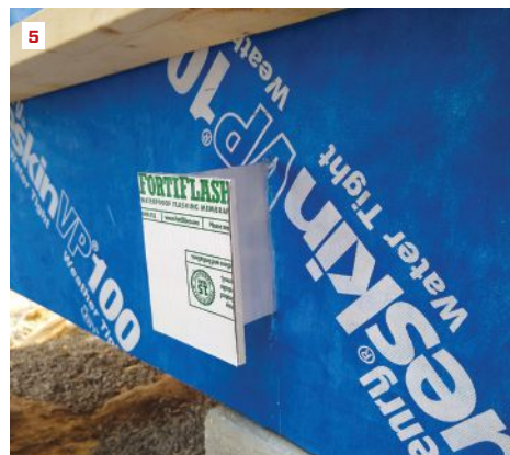
Deck brackets are bolted to the floor frame (1) through protective patches of FortiFlash Butyl membrane (2). The brackets and sheathing edges are sealed with Henry Air-Bloc LF (3, 4). The bracket faces are isolated from treated framing with FortiFlash (5).
