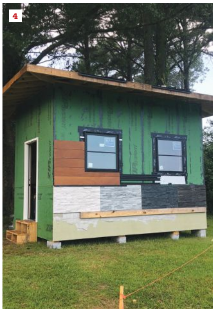
This small structure started out as a jobsite office (4) but soon became a perfect place to test different combinations of windows and claddings, including a thin adhered stone veneer in various colors and a rainscreen cladding system (5).
