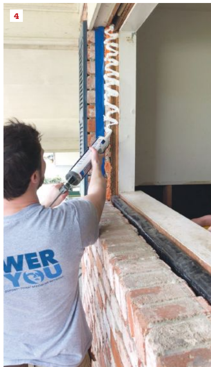
Some openings were prepped by filling the gap between the brick and the wall framing with gun foam (3), and caulking over the rough jambs (4). Site-bent coil stock was used at the head and sill of the openings (5) to direct water out to the face of the exterior.
