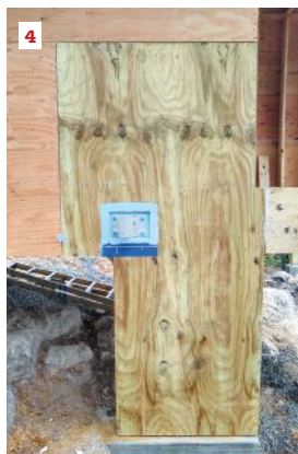
Deck brackets are bolted to the floor frame (1) through protective patches of FortiFlash Butyl membrane (2). The brackets and sheathing edges are sealed with Henry Air-Bloc LF (3, 4). The bracket faces are isolated from treated framing with FortiFlash (5).
