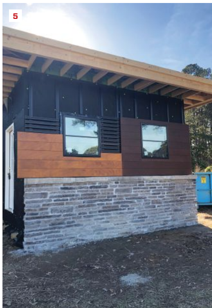
This small structure started out as a jobsite office (4) but soon became a perfect place to test different combinations of windows and claddings, including a thin adhered stone veneer in various colors and a rainscreen cladding system (5).
