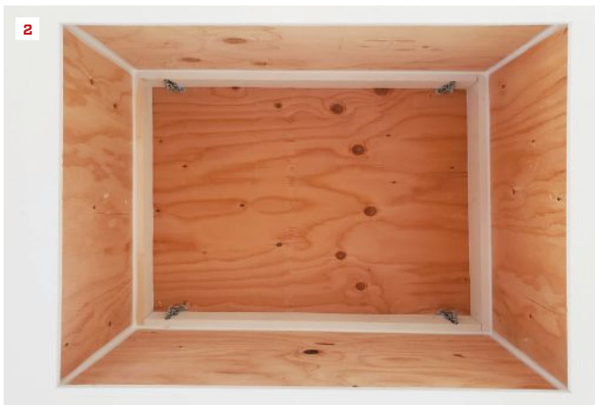
Viewed from below with the ceiling panel removed, the walls of the access extend far enough up to retain the blown-in insulation (1). With the airtight panel in place and all the corners sealed, the access completes the air barrier of the house (2).
