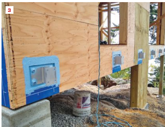
Deck brackets are bolted to the floor frame (1) through protective patches of FortiFlash Butyl membrane (2). The brackets and sheathing edges are sealed with Henry Air-Bloc LF (3, 4). The bracket faces are isolated from treated framing with FortiFlash (5).
