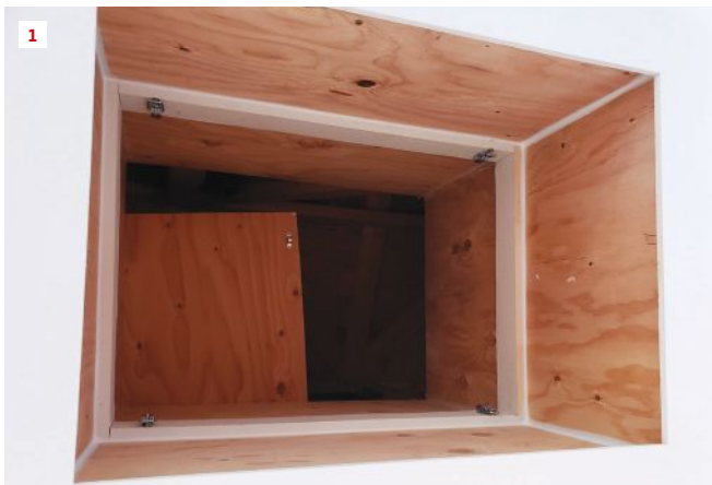
Viewed from below with the ceiling panel removed, the walls of the access extend far enough up to retain the blown-in insulation (1). With the airtight panel in place and all the corners sealed, the access completes the air barrier of the house (2).
