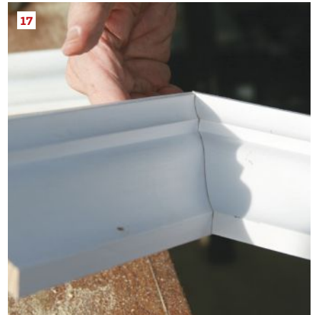
A coping foot mounts on a jigsaw in place of the footplate. The top three photos (12-14) show a typical sequence. For a mitered look, cut the angled sliver (15) and make a relief cut in the mating piece (16) so the two sides fit together (17).
