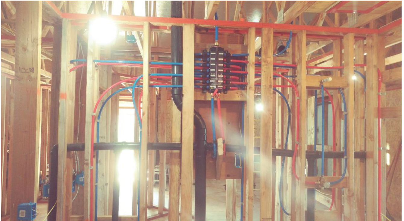
A view of the rough plumbing in a house under construction by the Habitat for Humanity affiliate in San Joaquin County, Calif. A short plumbing chase located in the double-wall partition between back-to-back bathrooms serves baths, toilets, and sinks in both bathrooms, as well as a kitchen sink at one end and a laundry at the other. Hot water is delivered to fixtures in seconds.
