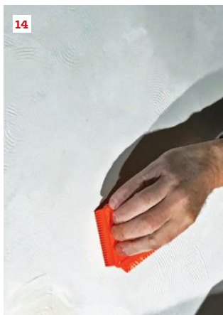
On this small crack, helper Derek Dawson uses a putty knife to flatten the new plaster and push it in along the edges (11). The electrical box is set at the proper depth to avoid interfering with the new finish (12). The lime-putty coat is applied in two passes; here, the first pass is made (13). Ron Bisson uses a texture comb to mimic an existing swirl pattern (14, 15).
