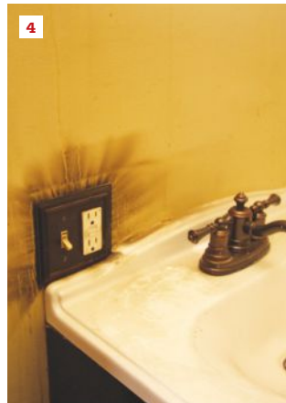
The fire started in an attached carriage barn (1), destroying stored family belongings (2). Abutting the barn, a butler's pantry was severely damaged as well (3). Smoke found its way into the main home via wall framing cavities (4).
