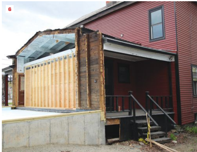
The demo work was completed within a week, with an excavator doing the bulk of the work in one morning (5). After gutting the home's one-story connector and sealing the framing with primer (6), the crew poured a new garage foundation.
