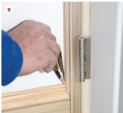
For small, straight line gaps, scribe with a pencil (5), and remove waste with a belt sander (6). Use a compass scribe for wider gaps (7) or for more finicky profiles (8).
