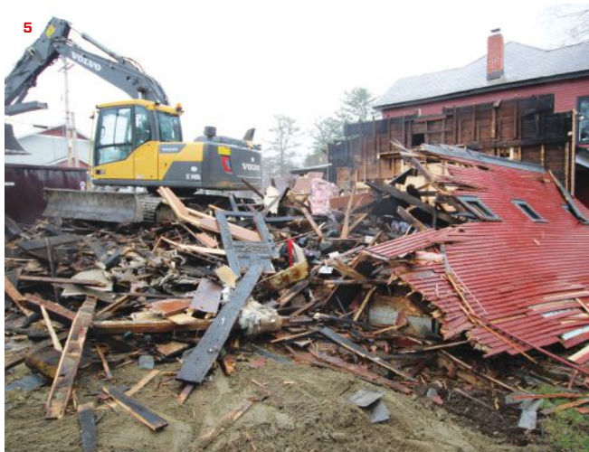
The demo work was completed within a week, with an excavator doing the bulk of the work in one morning (5). After gutting the home's one-story connector and sealing the framing with primer (6), the crew poured a new garage foundation.
