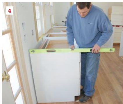
Common scribes are fitting baseboard to a floor (1) , scribing a cabinet to a wall (2) , and scribing to an irregular surface (3) . Shim cabinets level before scribing (4) .
