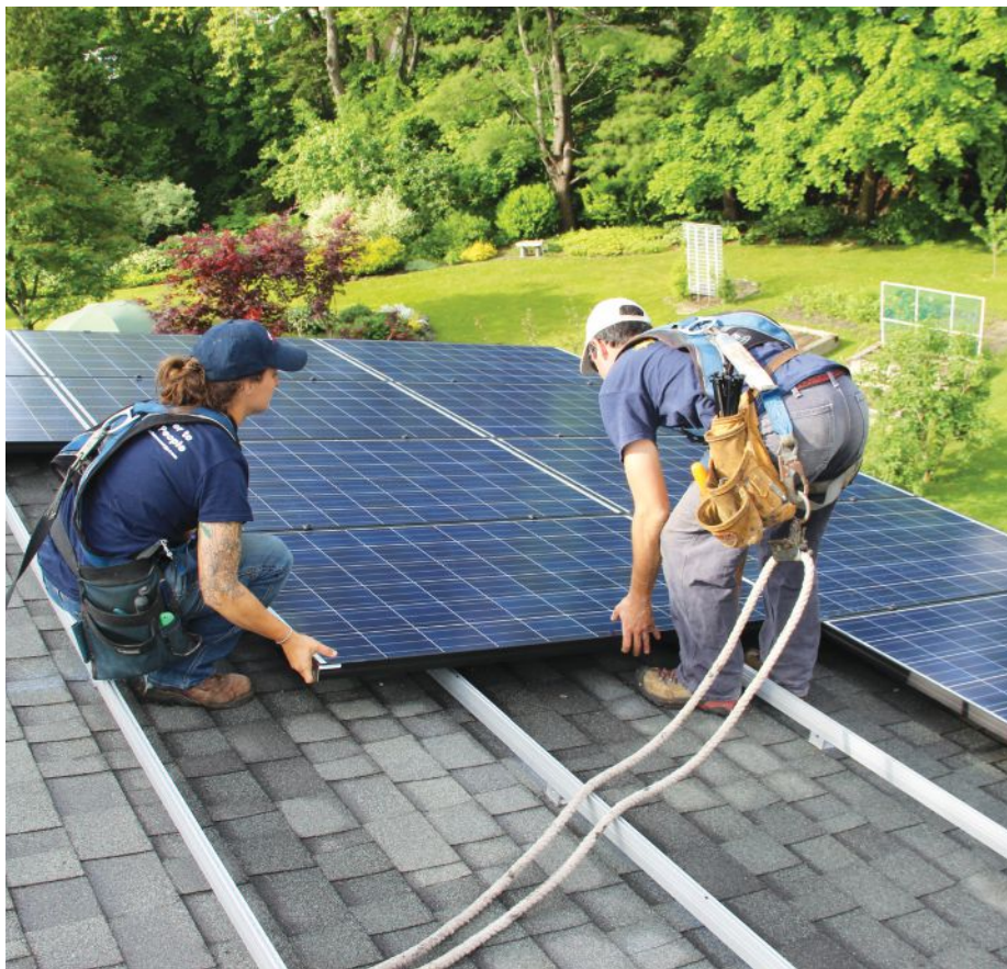
Low-pitched roofs such as this one are less sensitive to compass orientation than steeper roofs.
