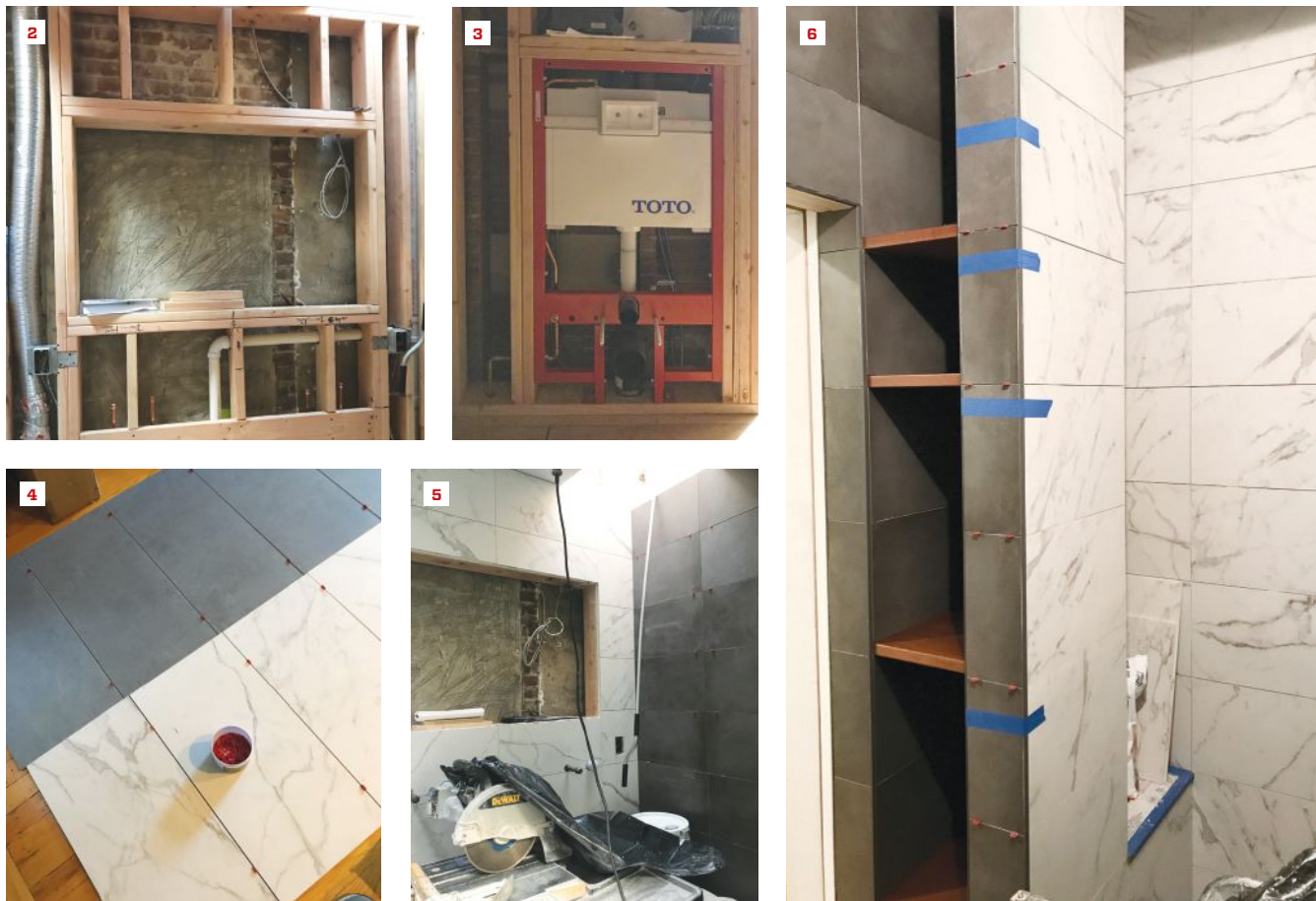
New 2x6 wall framing and solid blocking were needed for the wall-hung vanity and recessed cabinet above (2) and for the toilet's in-wall tank and mounting system (3). The two wall-tile selections were slightly different sizes (4), requiring different-sized grout joints to ensure that they lined up in the corners where they met (5, 6).
