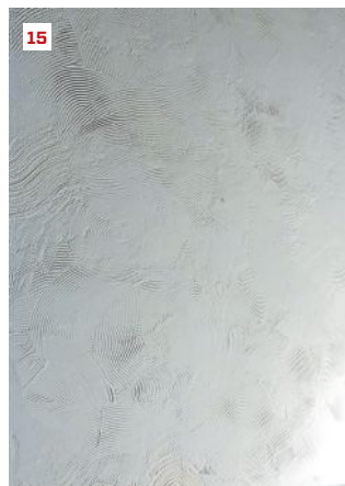
On this small crack, helper Derek Dawson uses a putty knife to flatten the new plaster and push it in along the edges (11). The electrical box is set at the proper depth to avoid interfering with the new finish (12). The lime-putty coat is applied in two passes; here, the first pass is made (13). Ron Bisson uses a texture comb to mimic an existing swirl pattern (14, 15).
