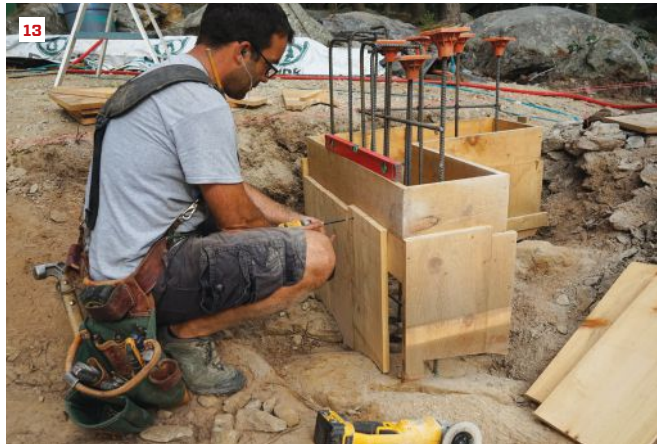
Pollard scribes a form board to the irregular rock using a compass (11), then cuts the outline with a jigsaw (12). He assembles the form using screws (13).
