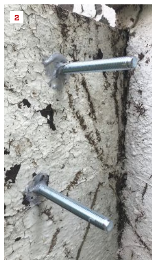
Three anchoring options: Epoxy, hammer-drive anchor, and wedge anchor (1). Bolts epoxied into concrete (2). Post attached with epoxied bolts and a hammer-drive anchor (3).
