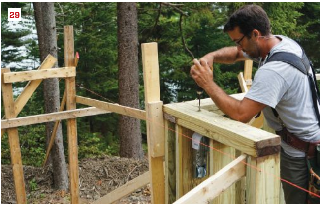
Pollard installs the top plate on a stem wall (27), then bolts a hold-down into place (28). He drills a hole in the top plate for the hold-down's threaded rod (29). Bradenday nails off the sheathing on a stem wall at 2 inches on-center, as specified by the engineer (30).
