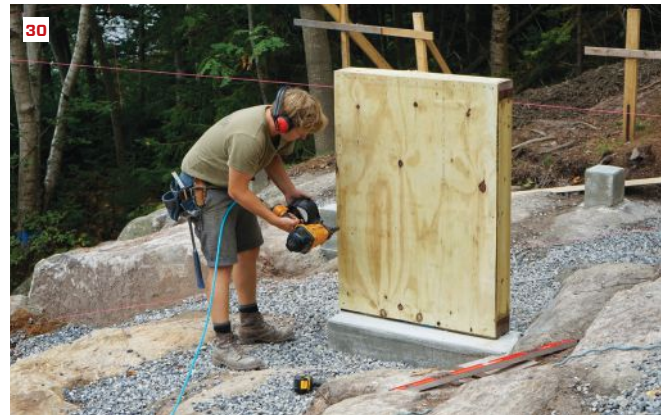
Pollard installs the top plate on a stem wall (27), then bolts a hold-down into place (28). He drills a hole in the top plate for the hold-down's threaded rod (29). Bradenday nails off the sheathing on a stem wall at 2 inches on-center, as specified by the engineer (30).
