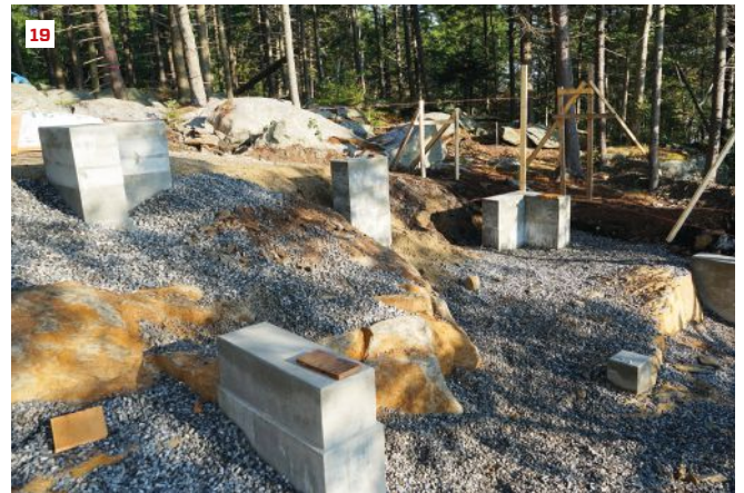
The crew fills forms with site-mixed bagged concrete, one bucketful at a time (14). Pollard vibrates a form using a recip saw (15) to consolidate the concrete. He strikes off the concrete level with the top of a form (16). After the concrete has set sufficiently, Wood tools the edge of a pier (17) and trowels the top (18). After forms are stripped, the piers stand ready for framing stem walls (19).
