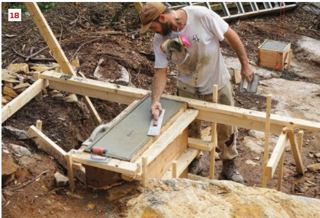
The crew fills forms with site-mixed bagged concrete, one bucketful at a time (14). Pollard vibrates a form using a recip saw (15) to consolidate the concrete. He strikes off the concrete level with the top of a form (16). After the concrete has set sufficiently, Wood tools the edge of a pier (17) and trowels the top (18). After forms are stripped, the piers stand ready for framing stem walls (19).
