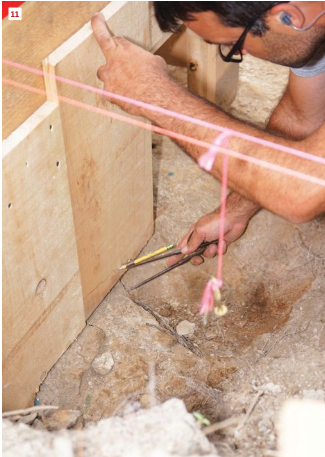
Pollard scribes a form board to the irregular rock using a compass (11), then cuts the outline with a jigsaw (12). He assembles the form using screws (13).
