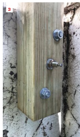
Three anchoring options: Epoxy, hammer-drive anchor, and wedge anchor (1). Bolts epoxied into concrete (2). Post attached with epoxied bolts and a hammer-drive anchor (3).
