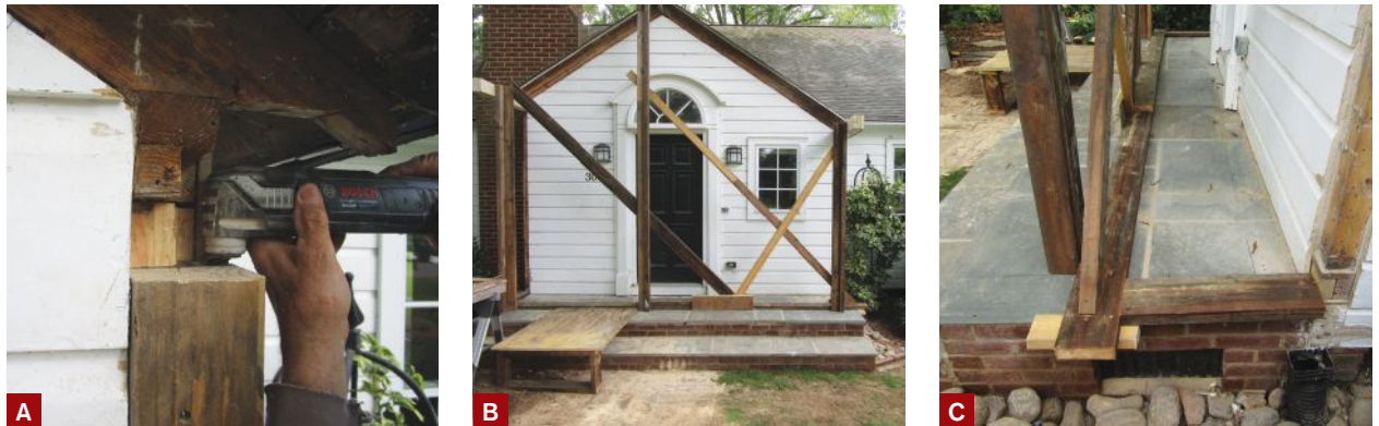
Figure 3. After removing the trim at the house corners and eaves, the author used a multitool and sharp chisel to cut pockets in the solid 4x6 corners for the beams that would support the new portico roof (A). To accurately lay out and support the triple 2x6 beams and 2x8 ridge, he installed vertical posts and diagonal bracing fastened to a temporary plate on top of the new masonry stoop (B). The plate was held in position with strategically positioned blocking (C).
