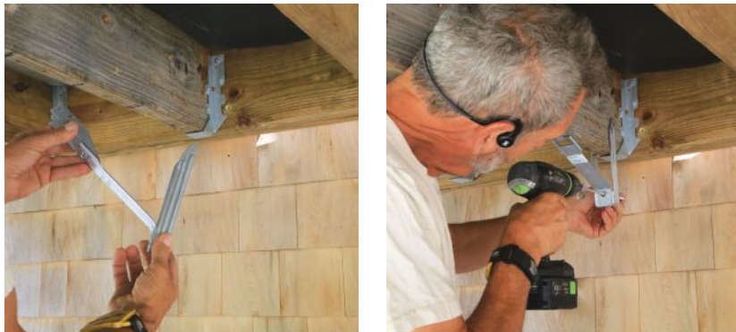
Figure 11. MiTek/USP's ADTT hardware can be adjusted to match the height of the wall plate (above left). The legs screw to the sides of the deck joist to form a triangle; the plate screw can be driven afterward (above right).
