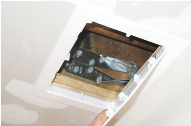
Figure 4. When there's a finished ceiling, cut a hole to match the size of the planned access panel and bore the rod hole through the ledger and rim joist from the outside. A right-angle drill/driver may be needed to screw the anchor to the side of the joist.
