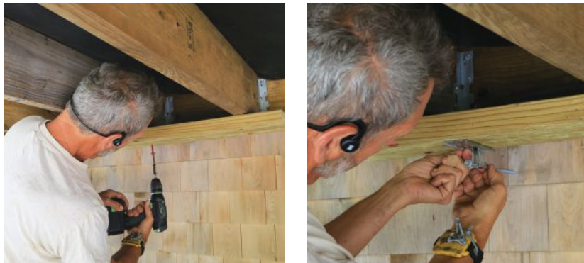
Figure 12. To fasten ties to wall studs rather than a plate, the author installs 2x8 blocking across the bottom of the deck joists (above left). The lateral-load hardware—FastenMaster LTS in this case—can then be accurately positioned for the \frac{3}{8} -inch lag screws to penetrate the studs (above right).
