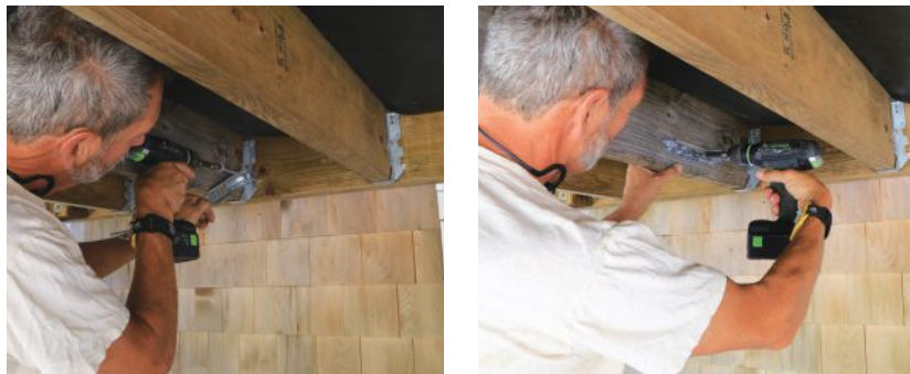
Figure 9. When installing the SST DTT1, slip the plate screw through the hole in the tie before driving it to the proper depth into the house framing (above left). Then fasten the tie to the joist (above right).
