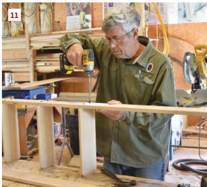
After predrilling for the screws, the author attaches one rail to the treads and the top rung (11). He then flips the assembly over and attaches the other rail (12).
