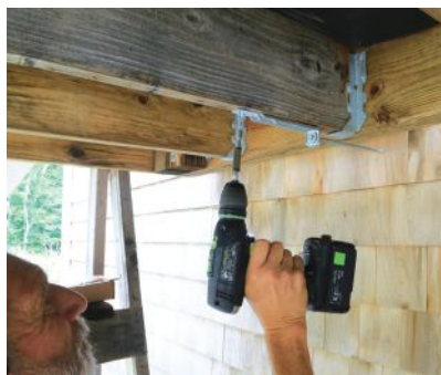
Figure 7. The IRC 4x750-lb. lateral-load detail is well suited for retrofits, since it doesn't require access to the house interior; here, an SST DTT1 tie connected to a \frac{3}{8} -inch lag screw embedded at least 3 inches into house framing is being fastened to the bottom of a deck joist (above left). Examples of hardware that meets the 750-lb. requirement include (above right, from left to right in photo) MiTek/USP ADTT, MiTek/LTS19, Simpson Strong-Tie DTT1, and FastenMaster LTS.
