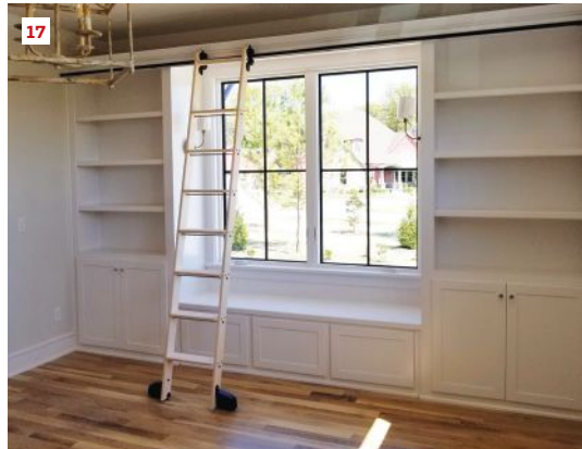
The cylindrical track came in sections that were cut to fit the built-in shelves. Brackets slide into the track on the first side and attach to the shelves. The ladder then slides onto the track. After inserting the splice hardware into the track (16), the second section attaches to the first, installed in similar fashion. The finished ladder is handsome and useful for accessing the bookshelves (17).
