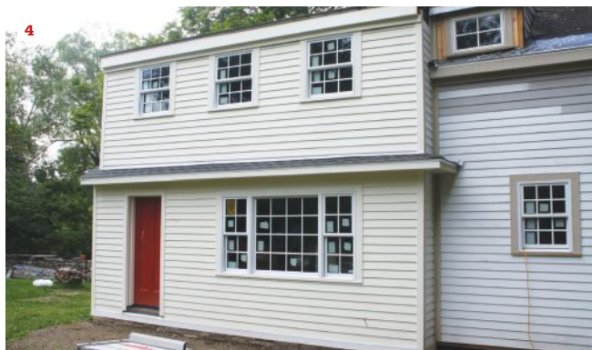
The original sagging dormer and roof-soffit assembly below revealed the building’s out-of-whack nature to the eye (1). The crew packed out the wall with Gutex insulation and strapping, then fastened on a new, tapered roof-and-soffit frame (2, 3). The finished facade blends the upper and lower structures together more harmoniously (4).
