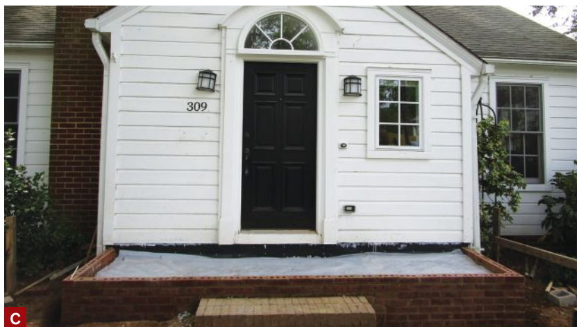
Figure 1. To expand the original front entry (A), the author removed its concrete slab deck and laid up a pair of block walls faced with brick on either side of the masonry stoop (B). Before pouring a new slab flush with the brickwork, he installed vinyl flashing to serve as a vapor barrier between the concrete and the mudd sill and primed the cut edges of the siding and trim (C).
