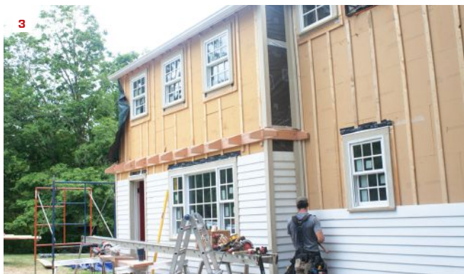
The original sagging dormer and roof-soffit assembly below revealed the building’s out-of-whack nature to the eye (1). The crew packed out the wall with Gutex insulation and strapping, then fastened on a new, tapered roof-and-soffit frame (2, 3). The finished facade blends the upper and lower structures together more harmoniously (4).
