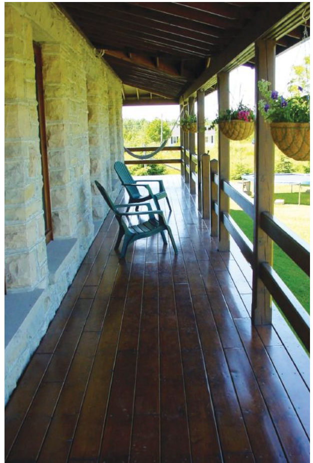
Figure 6. After being refinished with two coats of Cetol Dek, this decking has the patina of fine furniture. The first coat was with dark oak, while the second coat was a natural finish.
