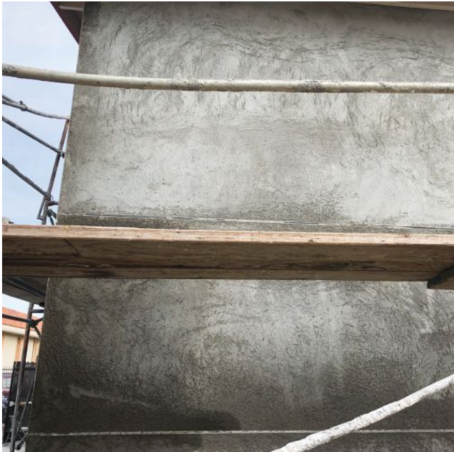
Above left, a well-applied brown coat has been smoothed flat with a straightedge (“rodded”) and floated with a green sponge trowel to bring out the sand aggregate. Above right, a brown coat has been scratched by a penny, indicating that the cure is incomplete. Curing should continue until a penny will not scratch the cured cement plaster.
