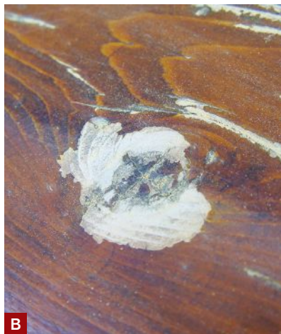
Figure 1. The film-forming finish on this white-cedar decking and PT rim joist is starting to fail (A), particularly around knots (B). After removing the old finish and refinishing with Cetol Dek, the cedar decking looks just like new (C).
