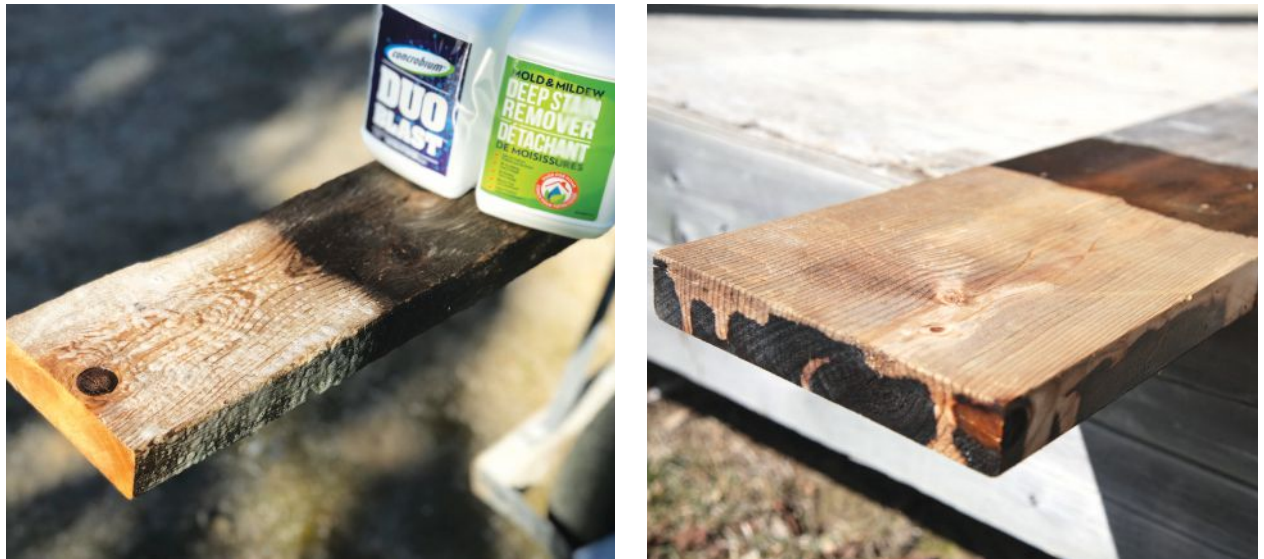
Figure 3. After removing the old finish, you may need to use a deck brightener to return color to weathered, gray decking. Some brighteners contain oxalic acid and need to be neutralized afterward, but the author recommends Duo Blast, which isn't harmful to plants and requires only a water rinse.
