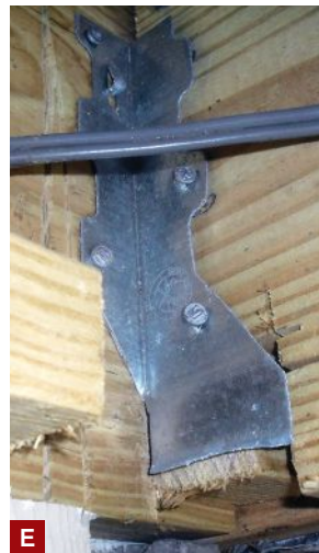
Figure 3. White rust is already forming on this joist hanger, which is only approved for interior use (A). Metal-roofing screws aren't approved joist-hanger fasteners (B), nor are roofing nails (C). All of the holes in metal hardware should be filled with approved hanger nails or structural screws, and the hanger flanges should fit snugly against the joist (D). Metal hardware shouldn't be field-modified; with its seat removed, this hanger provides minimal joist support (E).
