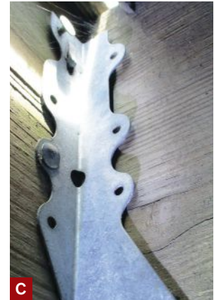
Figure 3. White rust is already forming on this joist hanger, which is only approved for interior use (A). Metal-roofing screws aren't approved joist-hanger fasteners (B), nor are roofing nails (C). All of the holes in metal hardware should be filled with approved hanger nails or structural screws, and the hanger flanges should fit snugly against the joist (D). Metal hardware shouldn't be field-modified; with its seat removed, this hanger provides minimal joist support (E).
