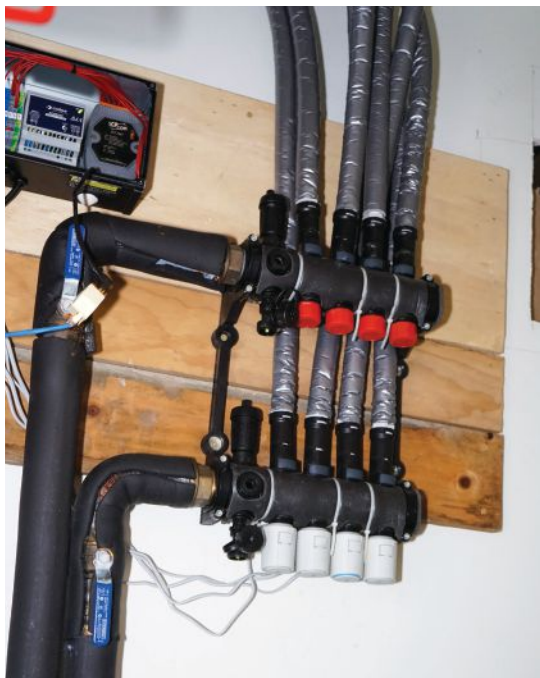
A manifold (above, left) allows the system to be zoned room by room. In a lower-floor mechanical room (above, right), a buffer tank isolates the indoor side of the system from the outdoor side, allowing the heat pump that powers the system to run efficiently without having to directly answer calls for cooling from the occupied space.
