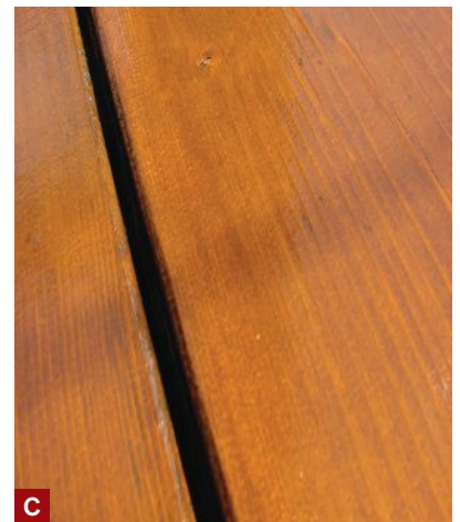
Figure 1. The film-forming finish on this white-cedar decking and PT rim joist is starting to fail (A), particularly around knots (B). After removing the old finish and refinishing with Cetol Dek, the cedar decking looks just like new (C).
