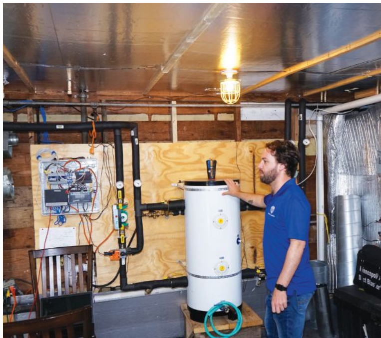
A manifold (above, left) allows the system to be zoned room by room. In a lower-floor mechanical room (above, right), a buffer tank isolates the indoor side of the system from the outdoor side, allowing the heat pump that powers the system to run efficiently without having to directly answer calls for cooling from the occupied space.
