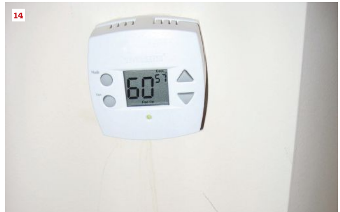
Moisture had soaked insulation above the poly vapor barrier of this wine room (11). The author vacuumed up puddles of water from on top of the poly (12). Bulk water was leaking into the room through a light fixture (13) and around a thermostat (14).
