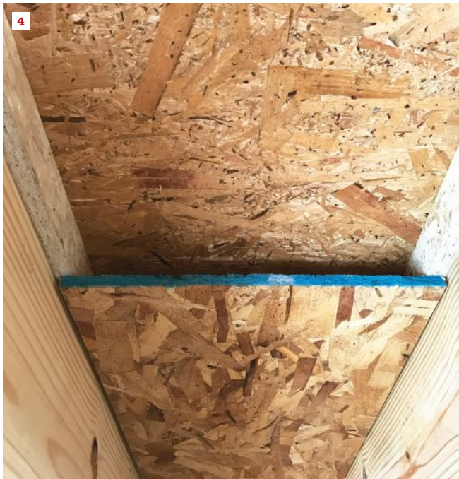
The 1½-inch vent channel terminates in the vented attic of the building (4). Spray foam is applied to the underside of the vent channel (5). If there are imperfections in the spray-foam application, the vent provides backup to clear any moisture.
