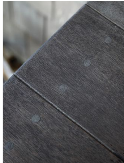
Matching the variable grain of the native pine shelving on the left would have been difficult; instead, mahogany plugs were used to create a contrasting accent. In the even-grained outdoor mahogany plank table on the right, plugs made from the same boards fill the fastener holes almost invisibly.
