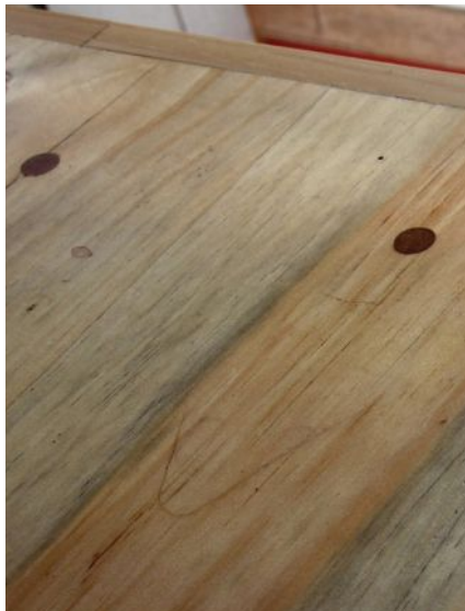
Matching the variable grain of the native pine shelving on the left would have been difficult; instead, mahogany plugs were used to create a contrasting accent. In the even-grained outdoor mahogany plank table on the right, plugs made from the same boards fill the fastener holes almost invisibly.
