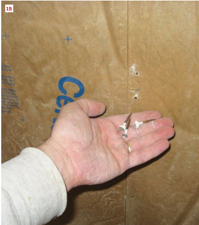
The author has seen more than one case of vapor drive through walls from the outside in. In one case, drywall screws were rusted by condensation (15). In another, mildew formed on the painted walls of the room (16).
