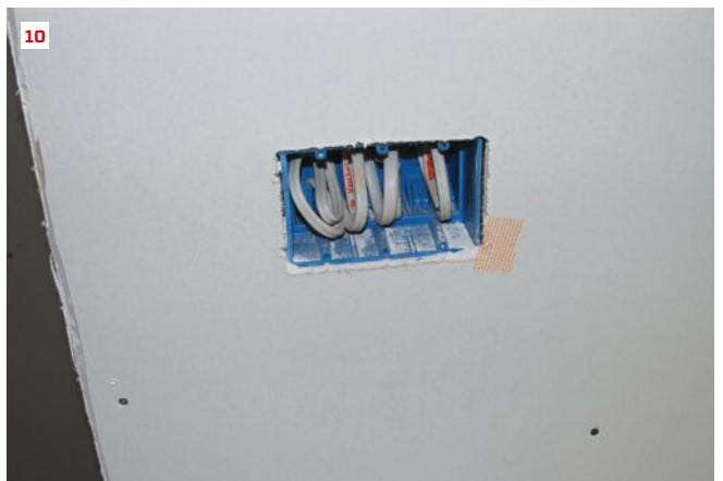
Repairing a damaged edge begins with slicing the paper around the damage (6) and removing the debris (7). The author then fills the hole (8) and covers it with mesh tape (9). Damage from cutting around electrical boxes also needs to be repaired (10).
