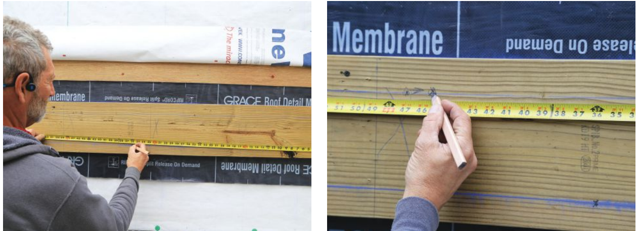
Figure 3. Fasteners are laid out on the ledger in two rows, starting approximately 3 inches in from one end, with the on-center spacing from the code table staggered in a “W” pattern between the two rows. Since bolt and lag heads can’t be countersunk into the ledger, the fastener can be moved left or right up to 3 inches to avoid conflicting with joist location or the hanger flange, provided the rest of the fasteners remain on the same layout.
