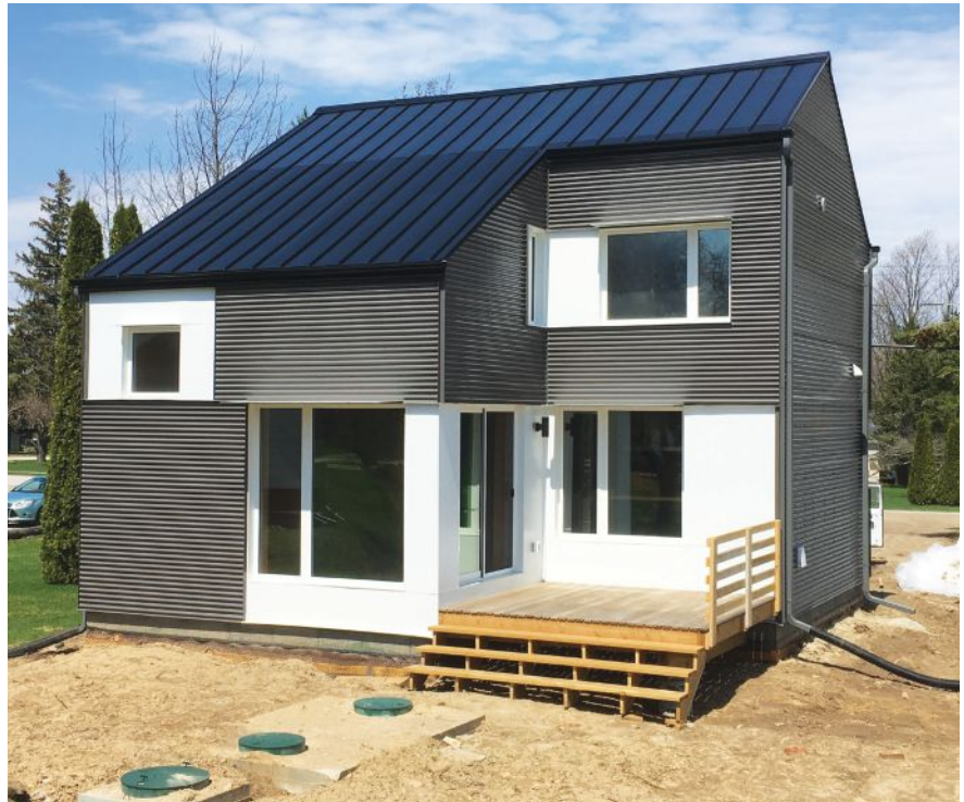
Built by Chris Magwood's Endeavour Centre in Clarksburg, Ont., this 1,100-square-foot zero-energy house cost $254 per square foot and stores 24 tons of CO 2 .
