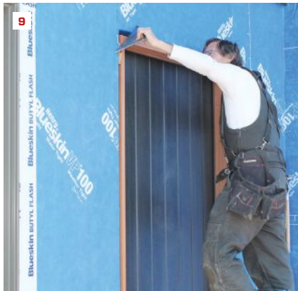
When the door is in position, shim behind the jamb at the bottom hinge (5) and on the opposite side as well (6). Check the sill for level (7), and shim if needed (8). Hold the door in plane with the wall (9), and shim both sides at the top (10).
