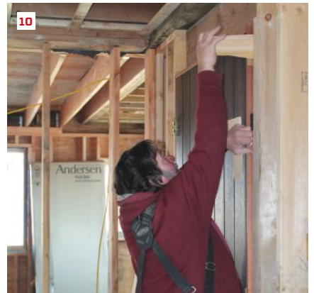
When the door is in position, shim behind the jamb at the bottom hinge (5) and on the opposite side as well (6). Check the sill for level (7), and shim if needed (8). Hold the door in plane with the wall (9), and shim both sides at the top (10).
