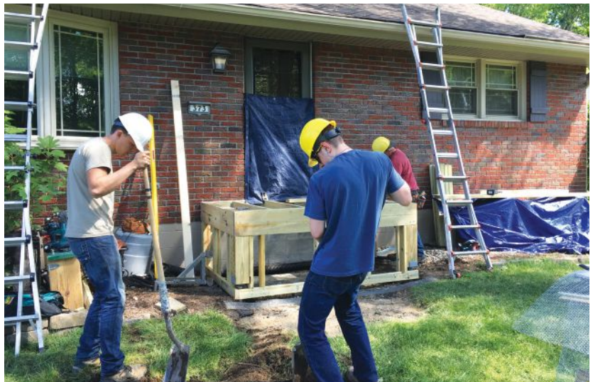
Figure 1. After the existing precast concrete stairway was removed, the author prepped the framing under the entry door to receive the new ledger (top). To keep rodents from burrowing under the enclosed porch, 12-inch-wide strips of diamond lath were nailed to the bottom of the framing and buried in the ground before the plywood sheathing was installed (bottom).
