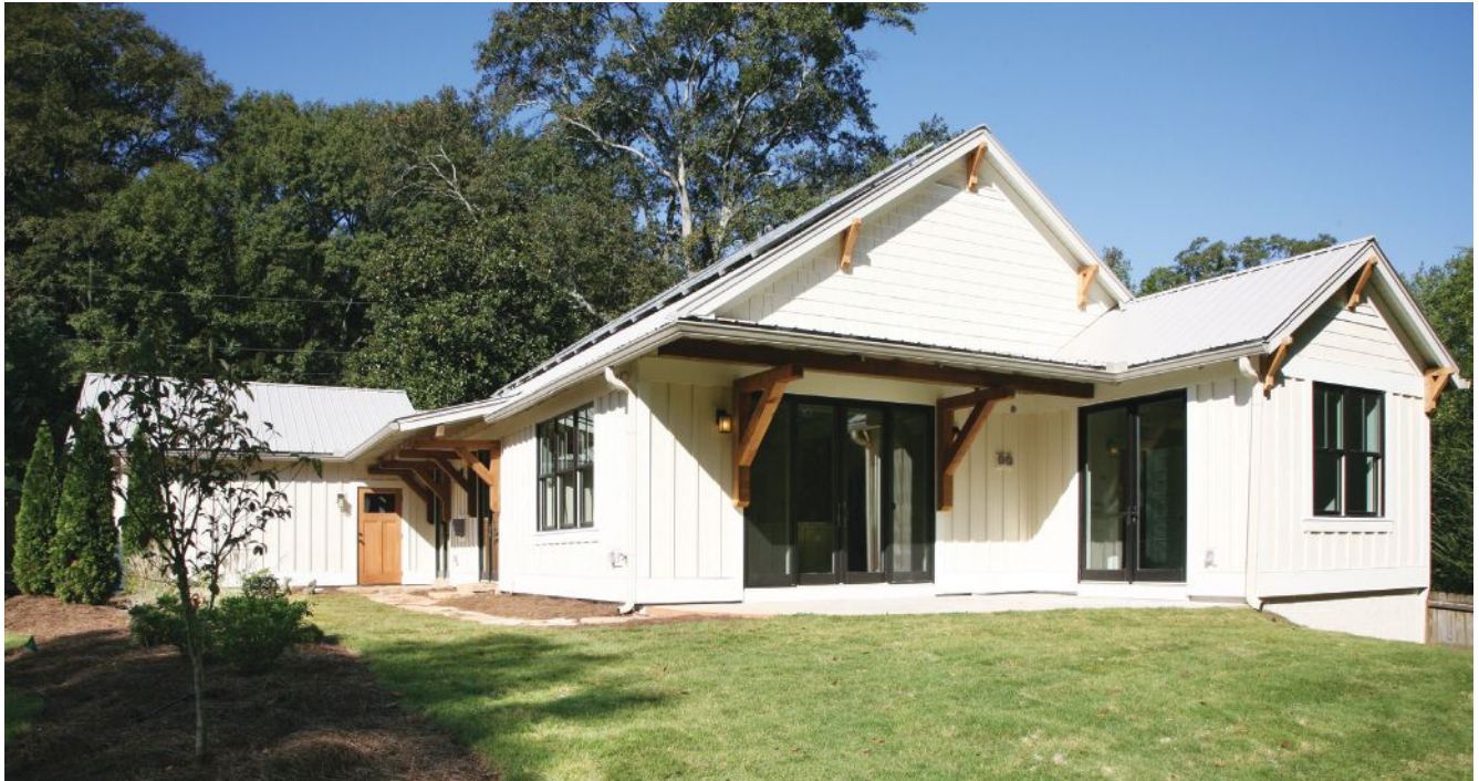
A net-zero house built by the Imery Group
