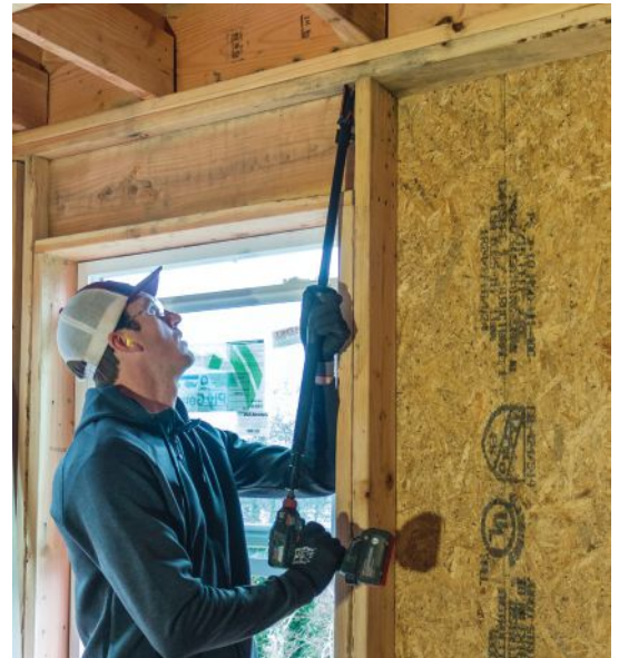
Simpson Strong-Tie's Quik Stik is an impact-driver extension that enables you to fasten through the top plate from the deck.
