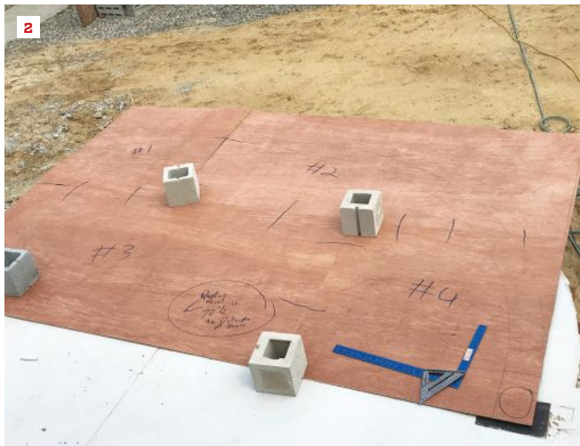
After laying out the curved beam directly on the first-floor slab (1), the author drew a full-size pattern on lauan plywood to help guide the metal fabrication (2). The porch columns would attach to the metal plates embedded in the slab. The author also made a story pole to record the heights of the two radiused beams, as well as the differences in the column heights due to the drainage slope of the slab (3).
