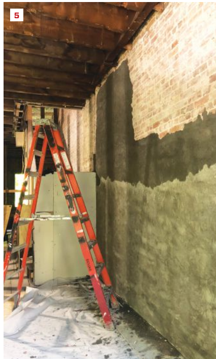
A lime mortar parge (4) is the first layer to be applied to the brick masonry after rough repair is completed. Next, the parge is coated with up to three coats of fluid-applied, vapor-open airtight sealing membrane (5). The final result is a fully membrane-coated wall (6), ready for blower-door testing to verify airtightness levels.
