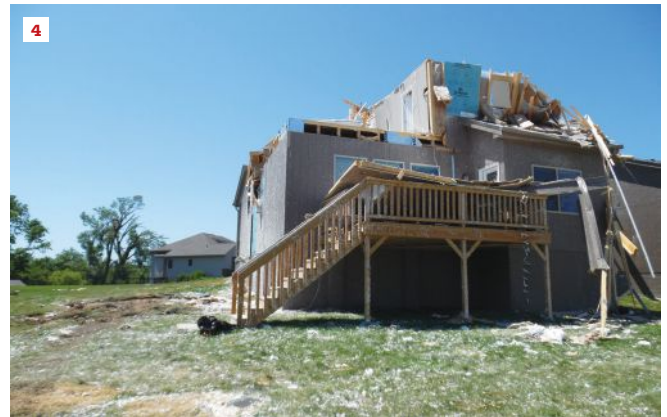
The photos above show failures in the upper portions of houses. Roof sheathing has been ripped away from trusses (1), an entire roof has been pulled off of its supporting walls (2), a gable end has been torn away from the roof and wall in one piece (3), and an entire second story has been lifted off the lower story (4). Each failure shows a different weak point in the load path.
