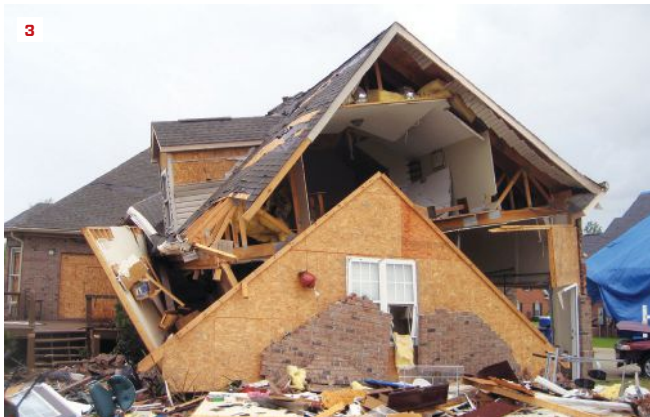
The photos above show failures in the upper portions of houses. Roof sheathing has been ripped away from trusses (1), an entire roof has been pulled off of its supporting walls (2), a gable end has been torn away from the roof and wall in one piece (3), and an entire second story has been lifted off the lower story (4). Each failure shows a different weak point in the load path.
