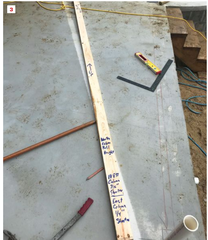
After laying out the curved beam directly on the first-floor slab (1), the author drew a full-size pattern on lauan plywood to help guide the metal fabrication (2). The porch columns would attach to the metal plates embedded in the slab. The author also made a story pole to record the heights of the two radiused beams, as well as the differences in the column heights due to the drainage slope of the slab (3).
