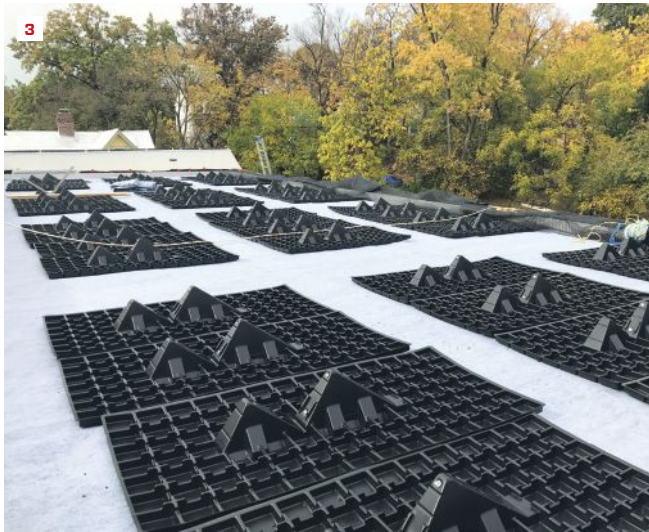
Durable plastic rack bases are set in place on the roof (3), then the geotextile mesh layer is rolled out, lapping over the plastic bases (4). Metal racking for the PV panels is anchored to the plastic bases, which will be ballasted by the green-roof growing media.
