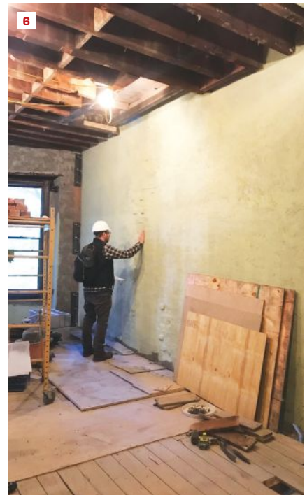
A lime mortar parge (4) is the first layer to be applied to the brick masonry after rough repair is completed. Next, the parge is coated with up to three coats of fluid-applied, vapor-open airtight sealing membrane (5). The final result is a fully membrane-coated wall (6), ready for blower-door testing to verify airtightness levels.
