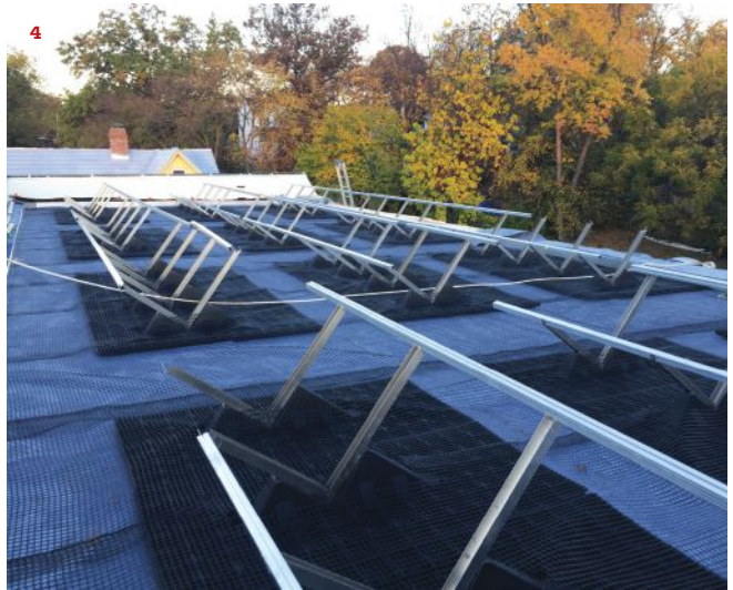
Durable plastic rack bases are set in place on the roof (3), then the geotextile mesh layer is rolled out, lapping over the plastic bases (4). Metal racking for the PV panels is anchored to the plastic bases, which will be ballasted by the green-roof growing media.
