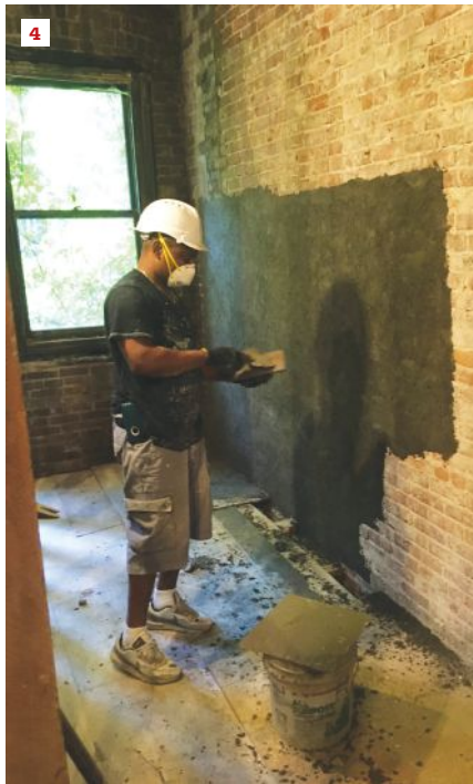
A lime mortar parge (4) is the first layer to be applied to the brick masonry after rough repair is completed. Next, the parge is coated with up to three coats of fluid-applied, vapor-open airtight sealing membrane (5). The final result is a fully membrane-coated wall (6), ready for blower-door testing to verify airtightness levels.
