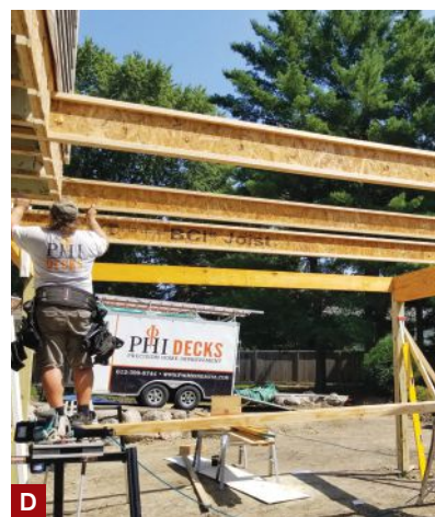
Figure 1. The deck's 6x6 PT support posts bear on Techno-Post P2 helical piles with a 16-inch-diameter helix and a 6,500-lb. bearing capacity (A). The new I-joists couldn't be hung from the cantilevered section of the house, so the crew carefully cut channels through the exterior sheathing and rim joist so that the joists could bear directly on the home's wall framing (B), and removed existing spray foam insulation for access to the basement wall framing (C). Where the 12-inch-on-center deck joists aligned with the 19.2-inch-on-center house joists, the author tied them together with mending plates (D).
