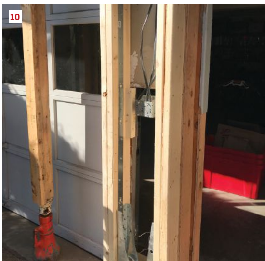
Flat straps attached with structural screws to the hold-downs and to the inside faces of the support studs reinforce the framing assembly (10). At the top, shorter straps reinforce the connection between the studs and the header (11).
