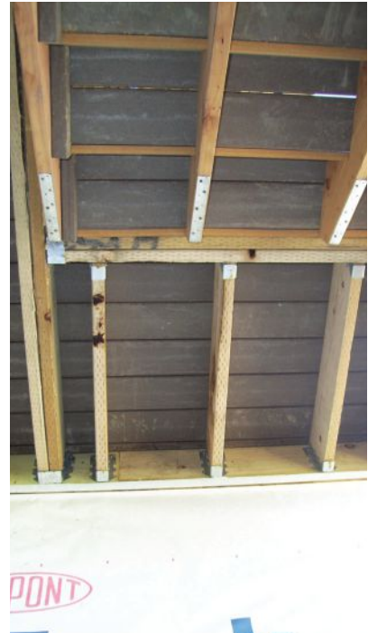
Figure 2. The double-ply beam supporting this stair landing is structurally unnecessary and could be replaced with a single 2x6, according to Table R507.5 in the 2018 IRC.
