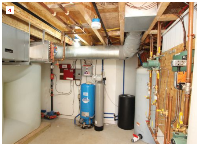
Under the floor, a fan draws outdoor air into a duct and passes it over a heating coil (4) before directing it up into the home’s living space. Controls open the intake damper, adjust the fan speed, and activate the heating coil as needed (see illustration, top).
