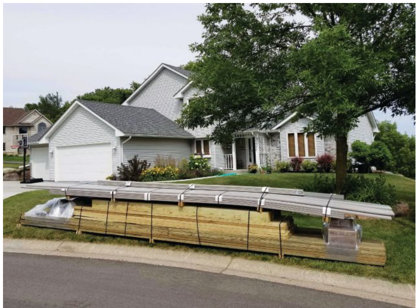
Produced off site, this deck package is ready for assembly. The same production techniques used to prefabricate the parts can be adapted to custom deck construction.
