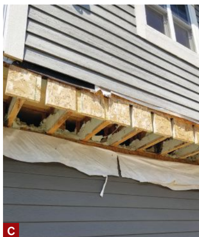
Figure 1. The deck's 6x6 PT support posts bear on Techno-Post P2 helical piles with a 16-inch-diameter helix and a 6,500-lb. bearing capacity (A). The new I-joists couldn't be hung from the cantilevered section of the house, so the crew carefully cut channels through the exterior sheathing and rim joist so that the joists could bear directly on the home's wall framing (B), and removed existing spray foam insulation for access to the basement wall framing (C). Where the 12-inch-on-center deck joists aligned with the 19.2-inch-on-center house joists, the author tied them together with mending plates (D).
