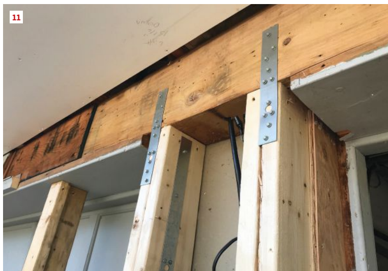
Flat straps attached with structural screws to the hold-downs and to the inside faces of the support studs reinforce the framing assembly (10). At the top, shorter straps reinforce the connection between the studs and the header (11).
