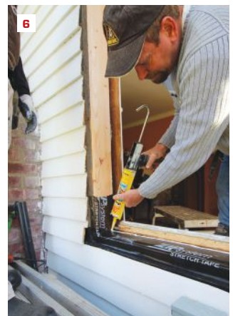
Complex interior trim (1) necessitated removing the 150-year-old windows from the exterior (2). New 2-by stock padded out the R.O. (3), while the sill “pan” was made from flashing tape products (4, 5). A bead of sealant acts as a back dam (6).
